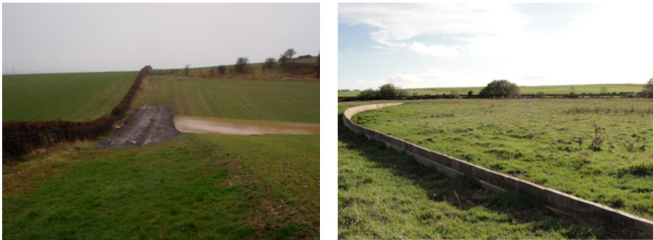
Figure 2-1: Example RAFs from Belford Northumberland (© Newcastle University)
