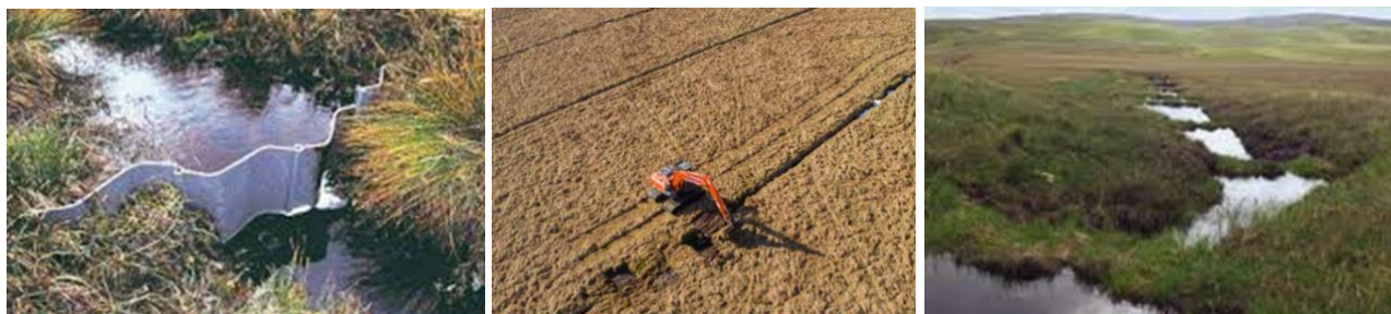
Figure 2-9: Examples of grip blocking (far left © RSPB, centre © Environment Agency, far right © Moors for the Future)
