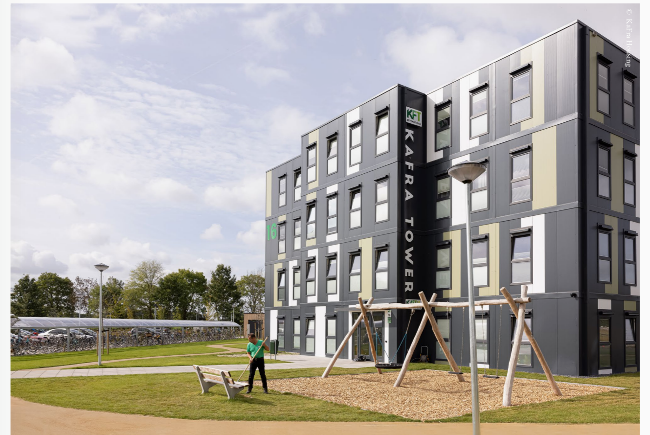
Interior and exterior of KaFra Tower Zevenbergen for labour migrants.
