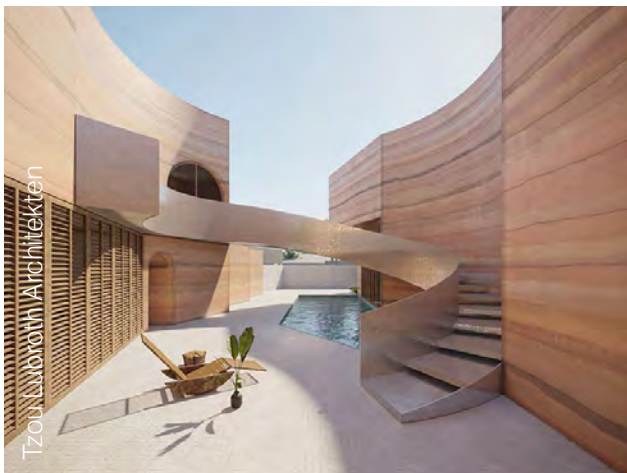
Figure 89: Example of rammed earth structure
