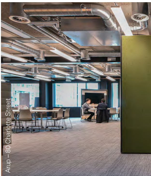
Figure 85: Examples of exposed ceiling (no suspended ceiling) versus typical demountable suspended ceiling
