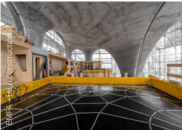
Figure 57: EMPA-ETH Zurich HiLo vaulted flooring system
