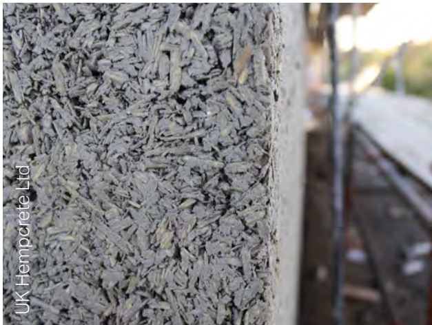
Figure 87: Example of hempcrete wall
