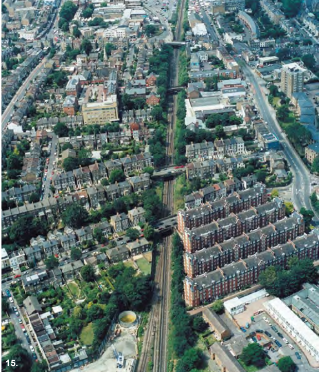
15. In North London, the HS1 tunnel runs under a densely populated area, following the route of the North London Line
