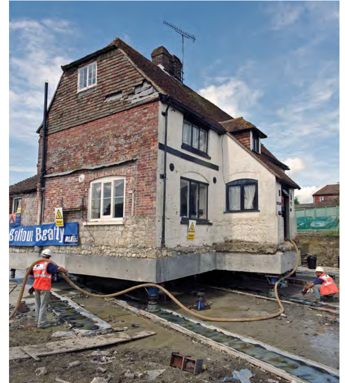
The historic Bridge House in Mersham, which stood on the HS1 route, was slid 80m to a new location
