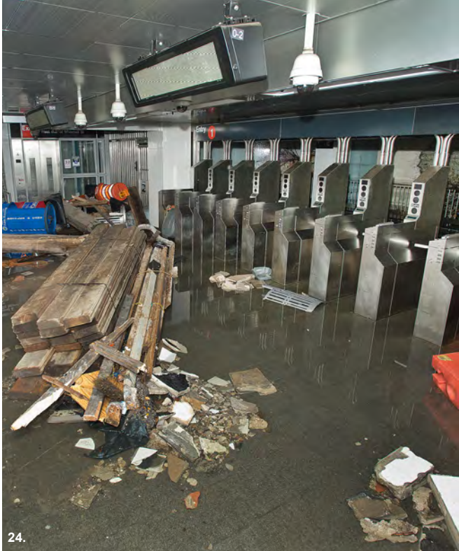
South Ferry subway station in New York was flooded during Hurricane Sandy
