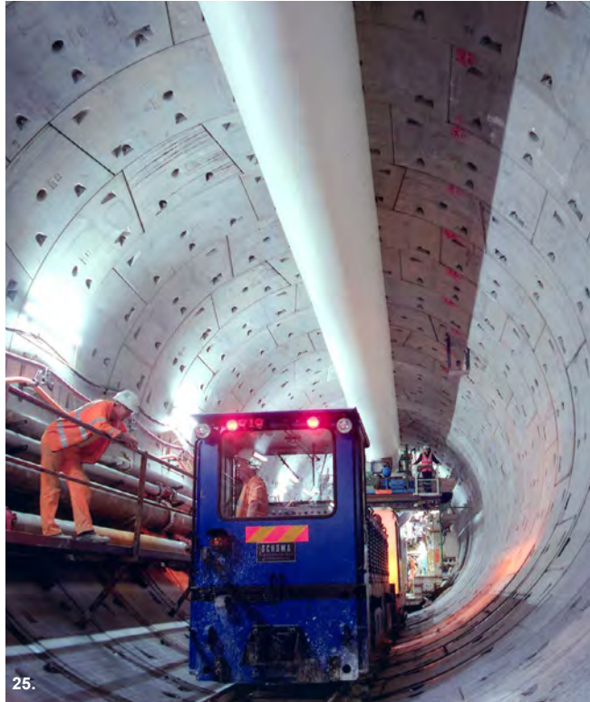
The CTRL tunnel passed under the Thames, necessitating the development of measures to prevent flooding
