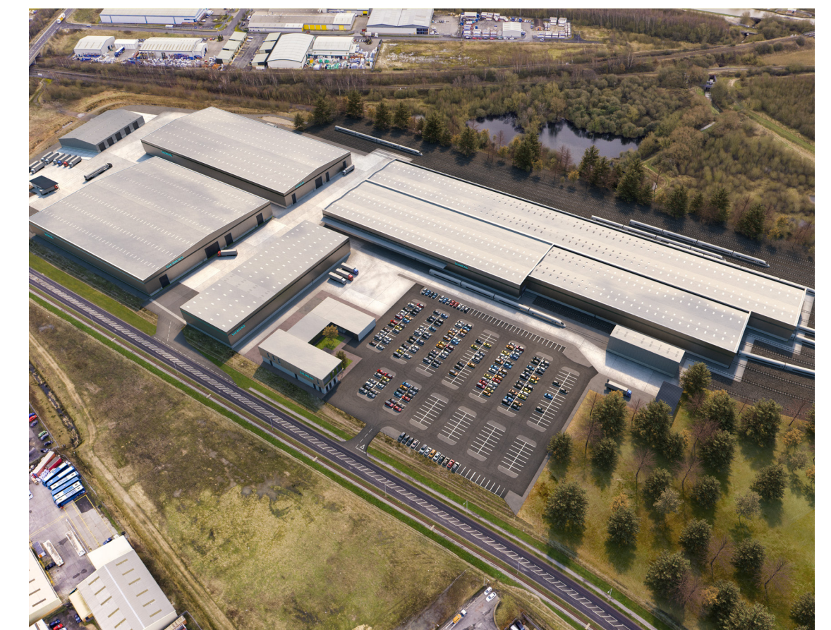
Siemens Mobility Manufacturing Facility, UK © Siemens Mobility
