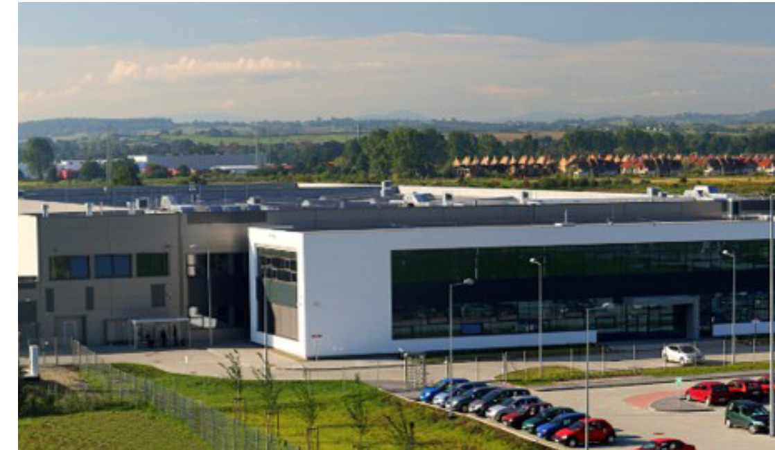
Somfy Electric Motors Factory, Niepołomice, Poland © Arup
