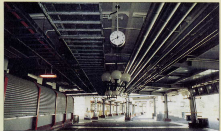
8. Service runs under roof.
