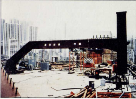
5. Lightweight steel hanging stairs. 6. Bracing between rear elevation columns.
