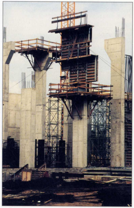
8. Construction in progress, September 1990.
