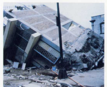
9. Foundation failure, Mexico City, 1985.
