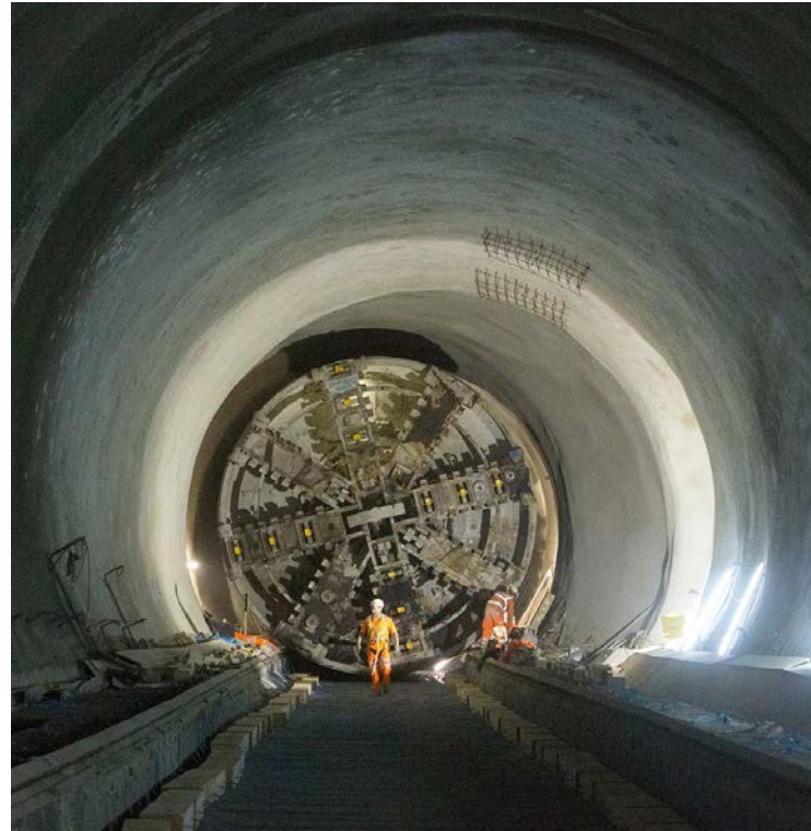
6: Arup's work on HS1 informed the tunnelling strategy and helped to minimise the number of boring machines needed 7: Arup's design work included mitigating ground movement caused by tunnel and station excavations
