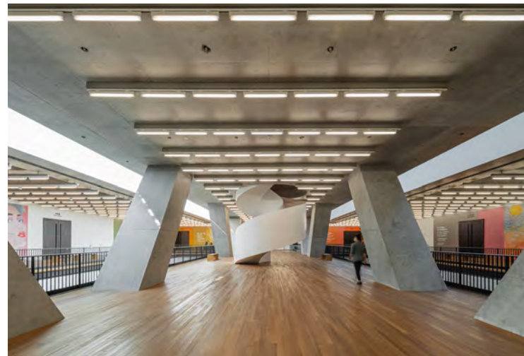
9: The transfer trusses are part of the visual design of the building, with aspects of them left exposed
