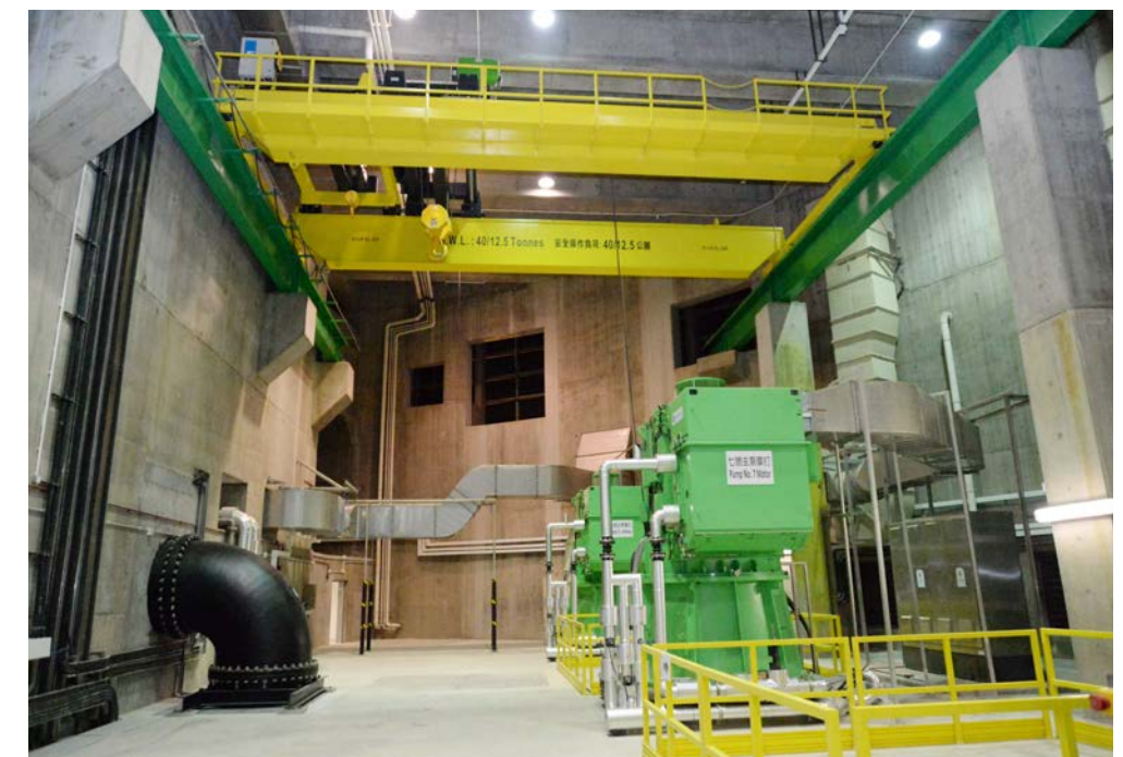
7: The Stonecutters Island main pumping station is one of the largest in the world, at 55m in diameter and 40m deep 8: There are eight main pumps in the pumping station motor hall
