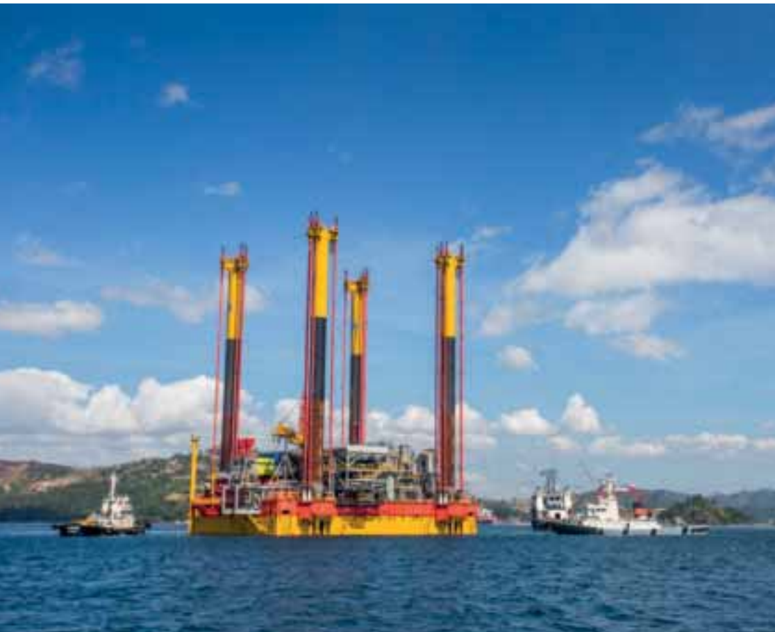
7. DCP during handover to the transport and installation contractor in Subic Bay.
