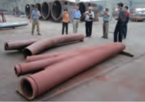
39. Casting Concourse roof elements. 40–41. Crane structures in position.
