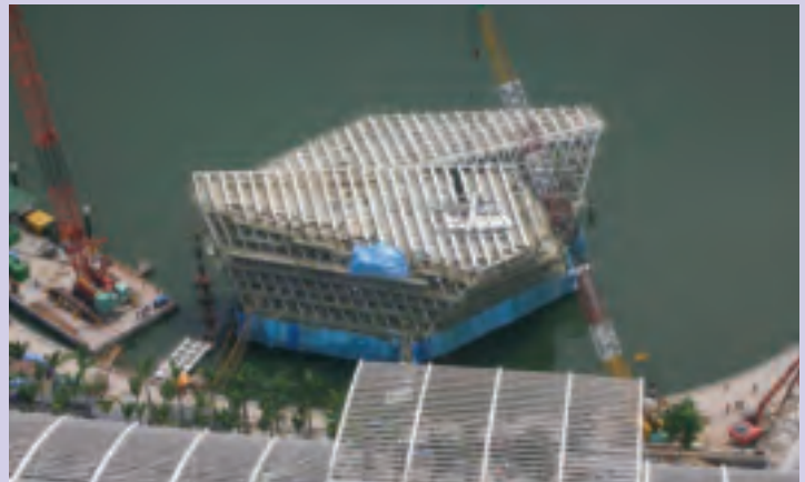
c) North Pavilion, July 2010.
