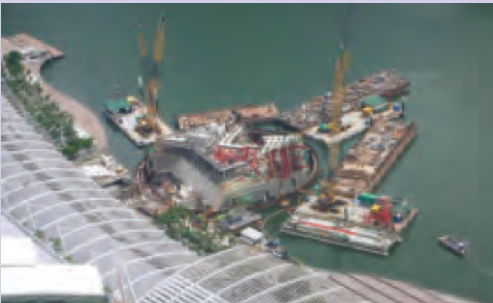
a) South Pavilion, July 2010.
