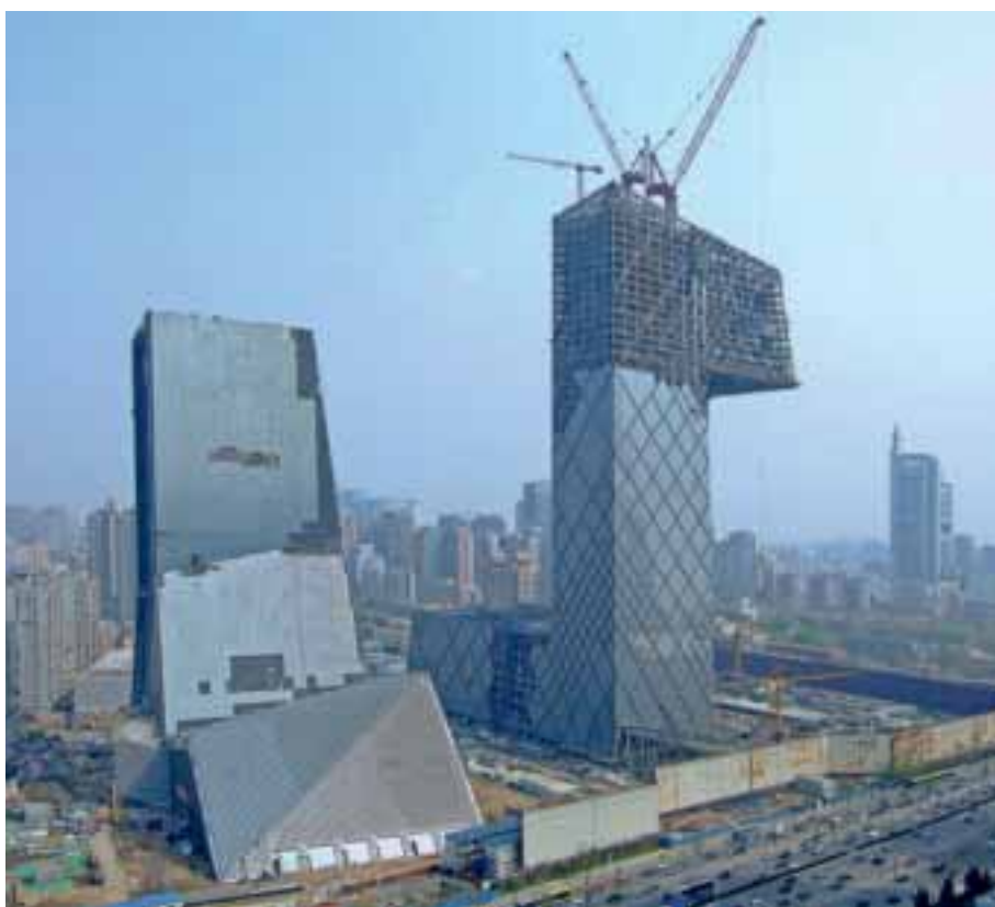
28. The TVCC building, to the left of the CCTV headquarters, April 2008.
