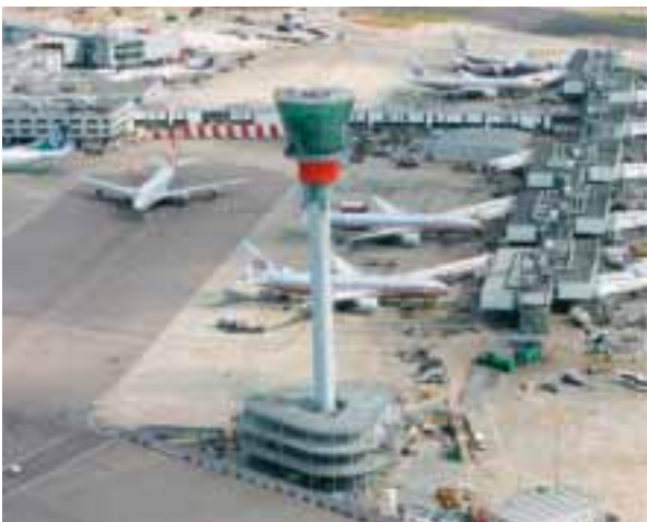
17. Tower and base building under construction.
