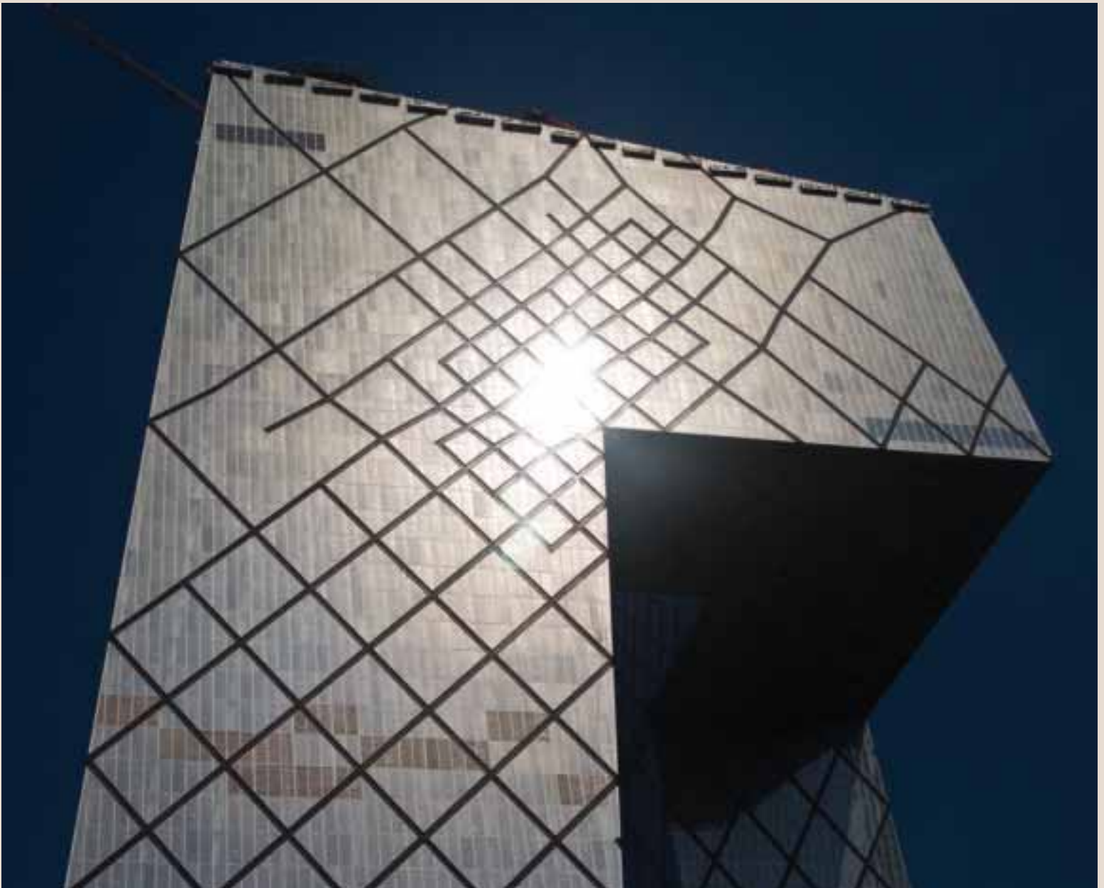
27. The façade design includes large diagonal “diagrid” elements that span between each primary floor, mirroring the structural braces.
