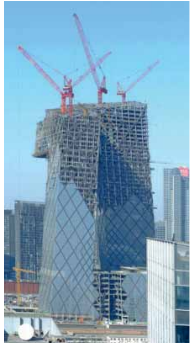
26. Construction progress at March 2008.
