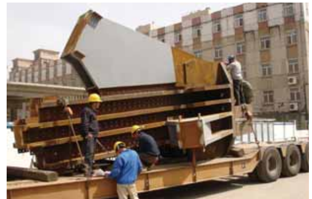
9. Delivery of column baseplate, April 2006.
