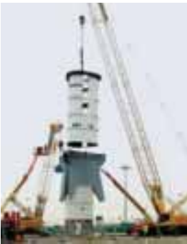
12. Erecting the two top mast sections for cab construction.
