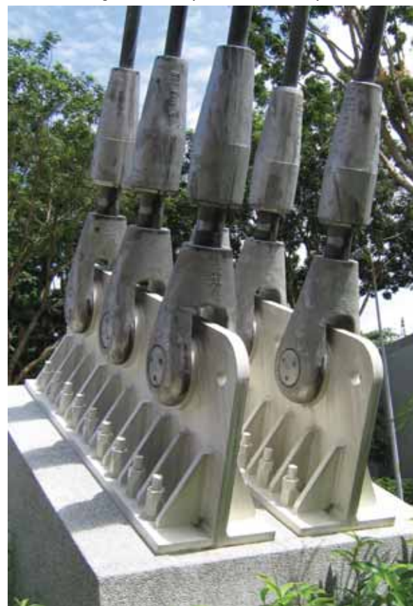
13. Anchorages in the courtyard for the cable stays.
