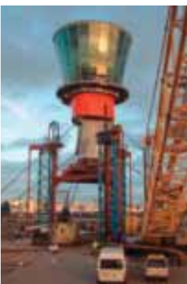
15. Jacking the cab to 87m height.
