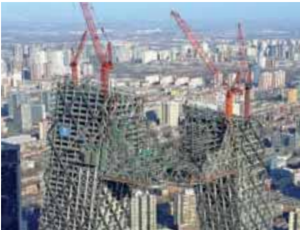
23. Installation of first connection element.
