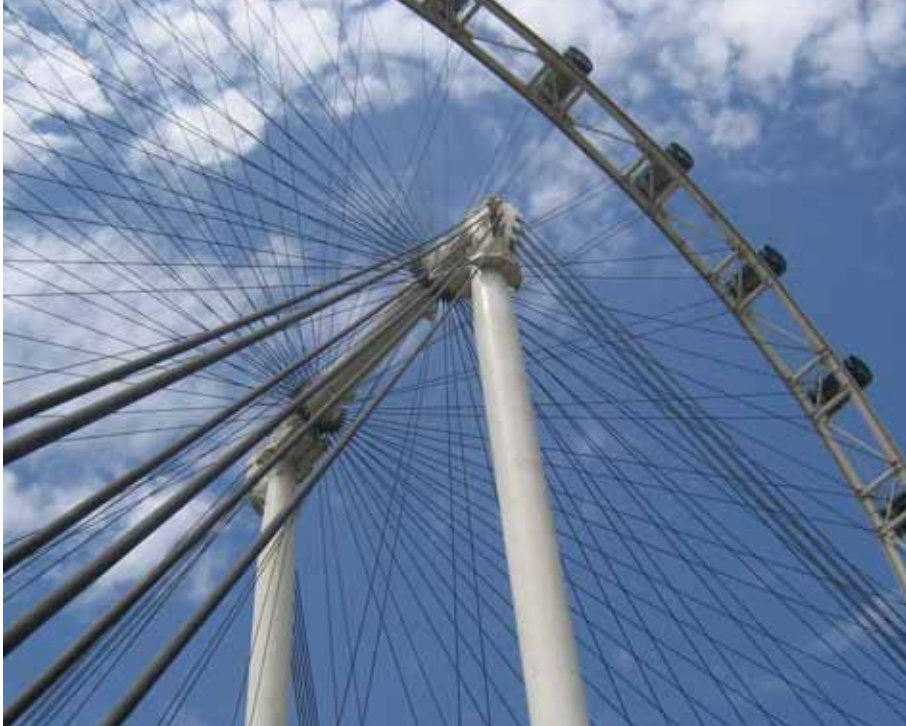
10. The wheel is supported by two 2.85m diameter columns.
