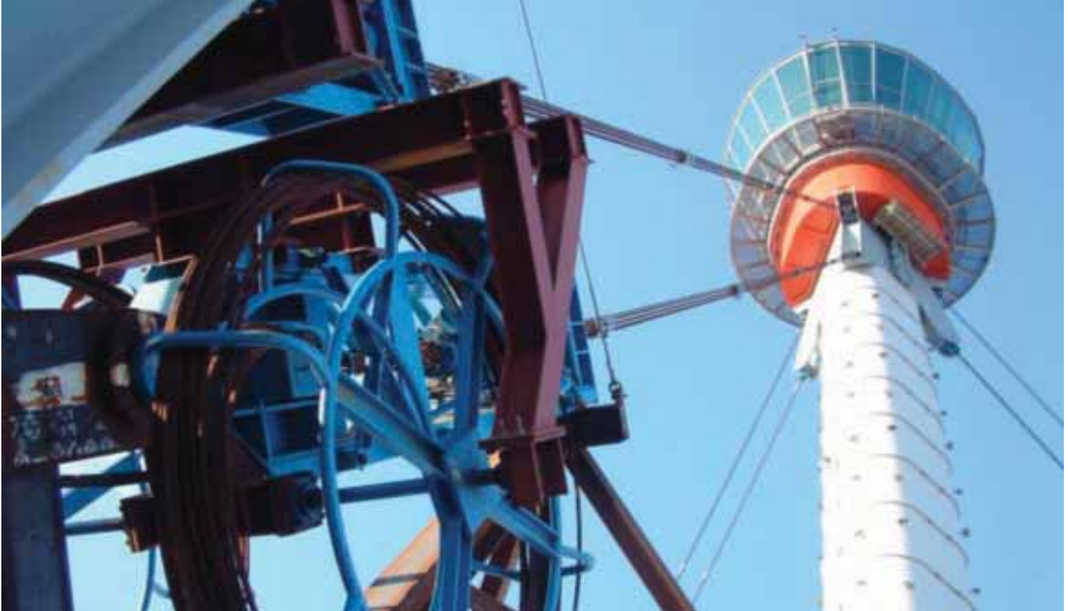
16. Jacks controlling guy cables during the lift.
