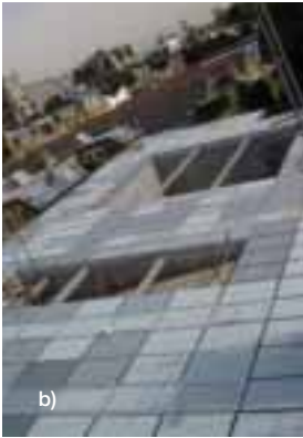
11. The Light House, Notting Hill, London: arrangement of façade and roof panels optimised to fulfil a set of internal environment parameters.
