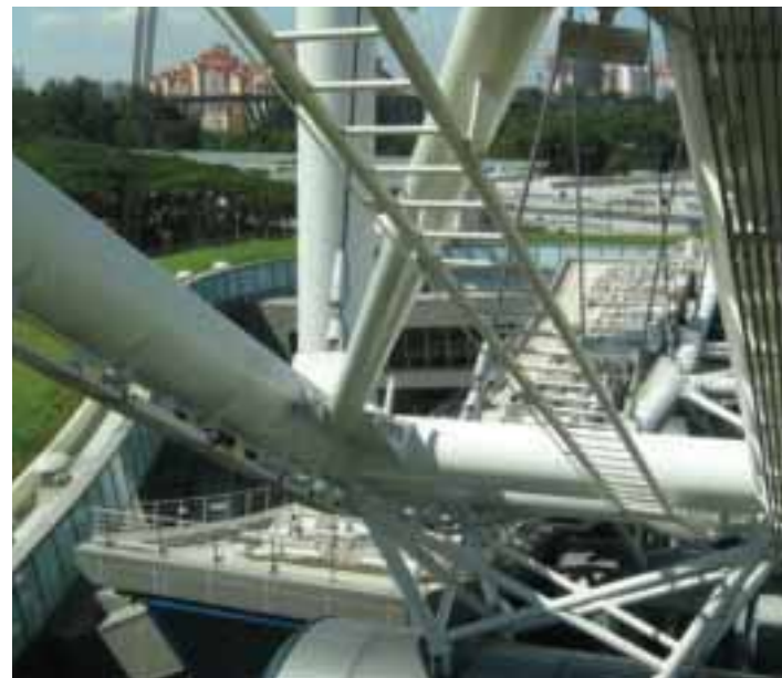
30. Passenger boarding bridge.
