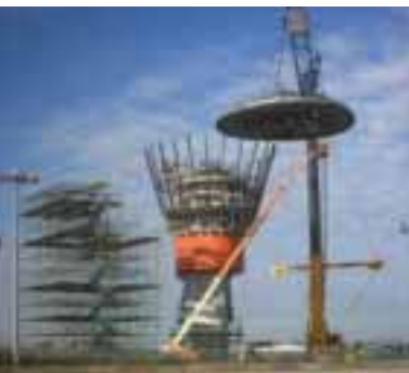
13. Locating cab roof onto 24 mullions.
