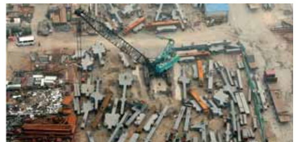
13. Prefabricated elements stored on site.
