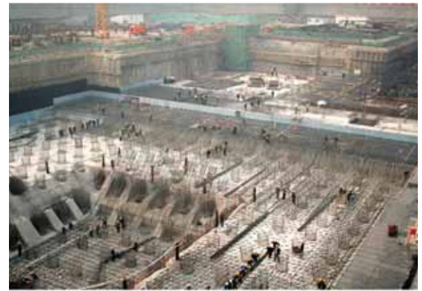
8. Preparation of foundation raft.
