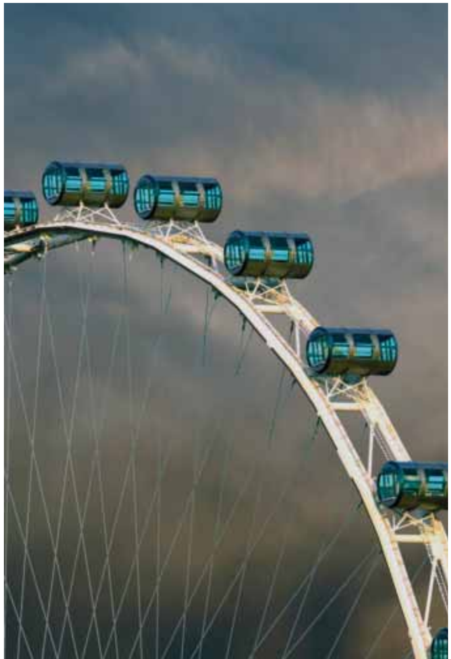
15. The Flyer rim is a “third generation” two-dimensional lattice truss.
