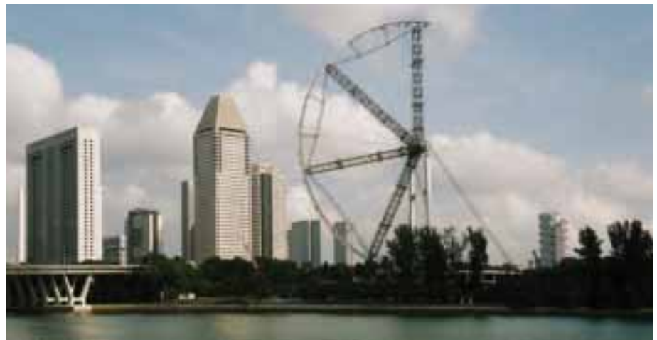
25. View looking north-west during erection.
