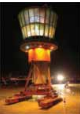
14. Moving 900 tonnes 1.5km across the airport.
