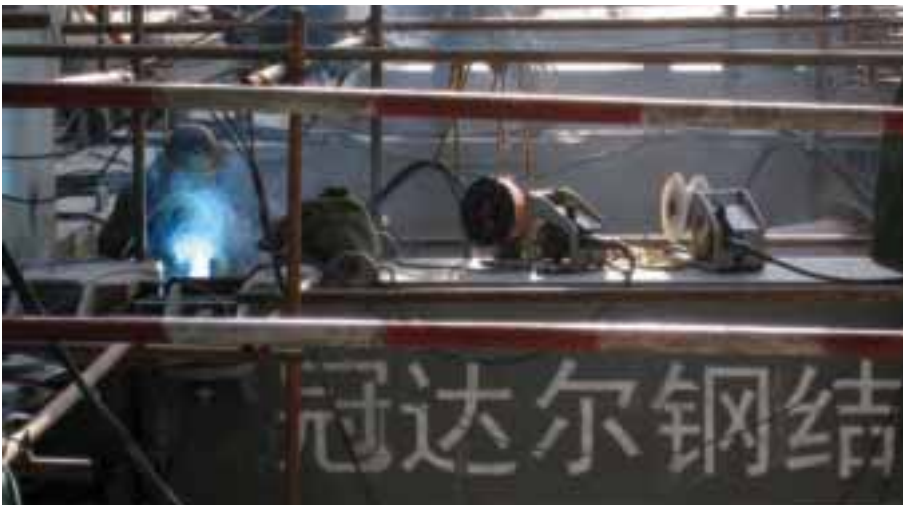
16. Welding in process.
