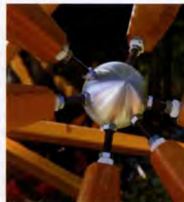
5. Completed aluminium node joint.
