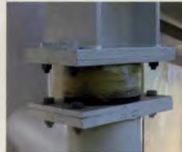
26. Elastomeric bearing at the drum bracket support.
