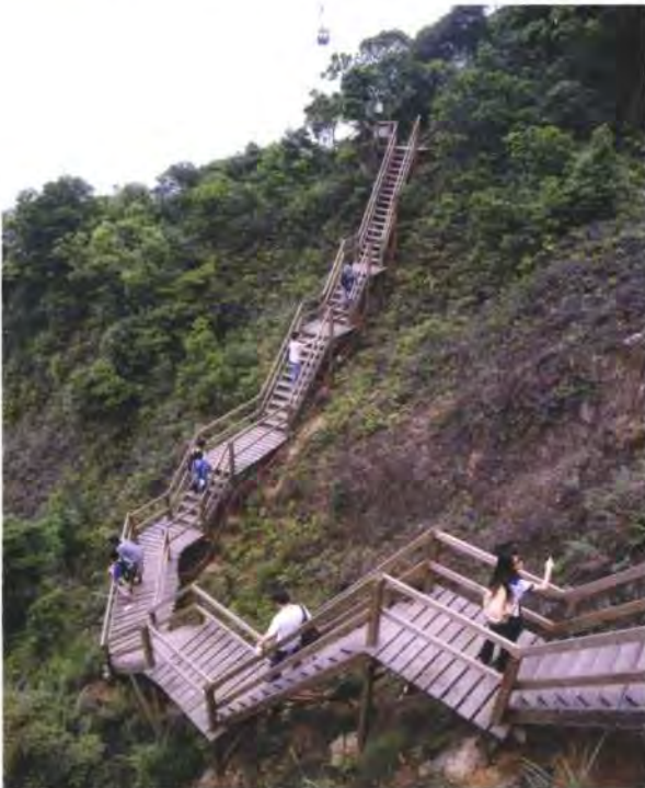
25. Detail of rescue trail timber construction.
