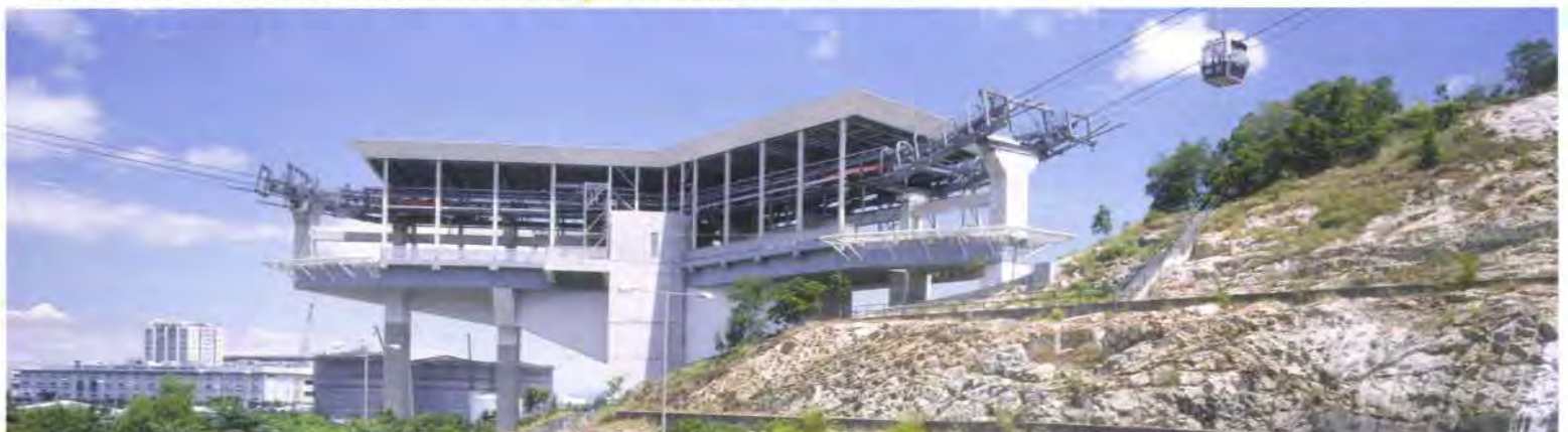
10. 120° angle between the AIAS arms leading to Tung Chung terminal building and to the NLSAS.
