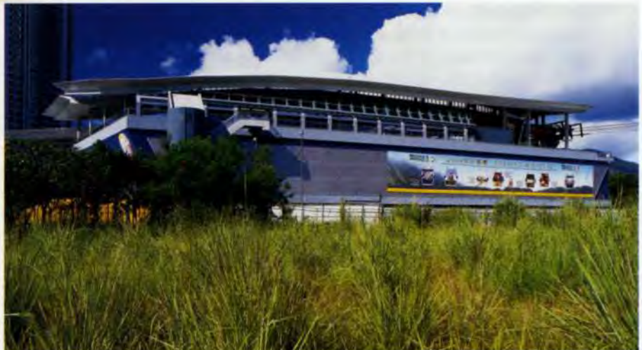
29. Value engineering at Tung Chung terminal: the roof geometry was developed with straight members and elimination of purlins for simplicity of fabrication, in spite of the complex shape.
