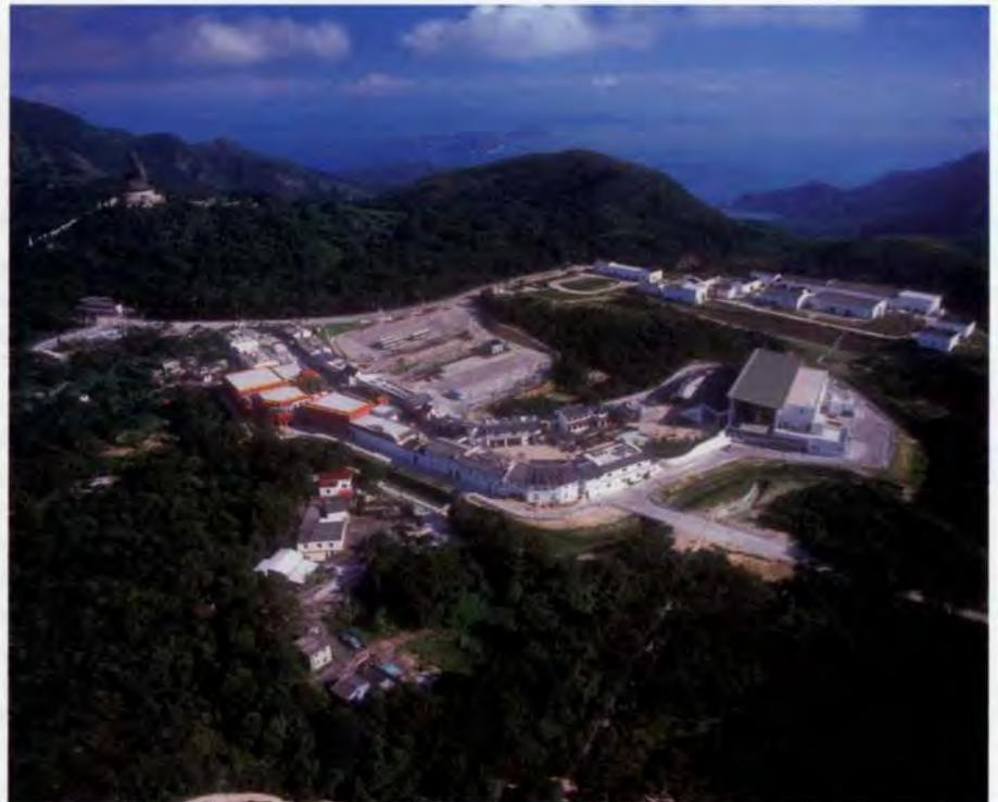
23. Ngong Ping Village: the terminal building is on the right, with Ngong Ping sewerage treatment works (another Arup project) in the background.
