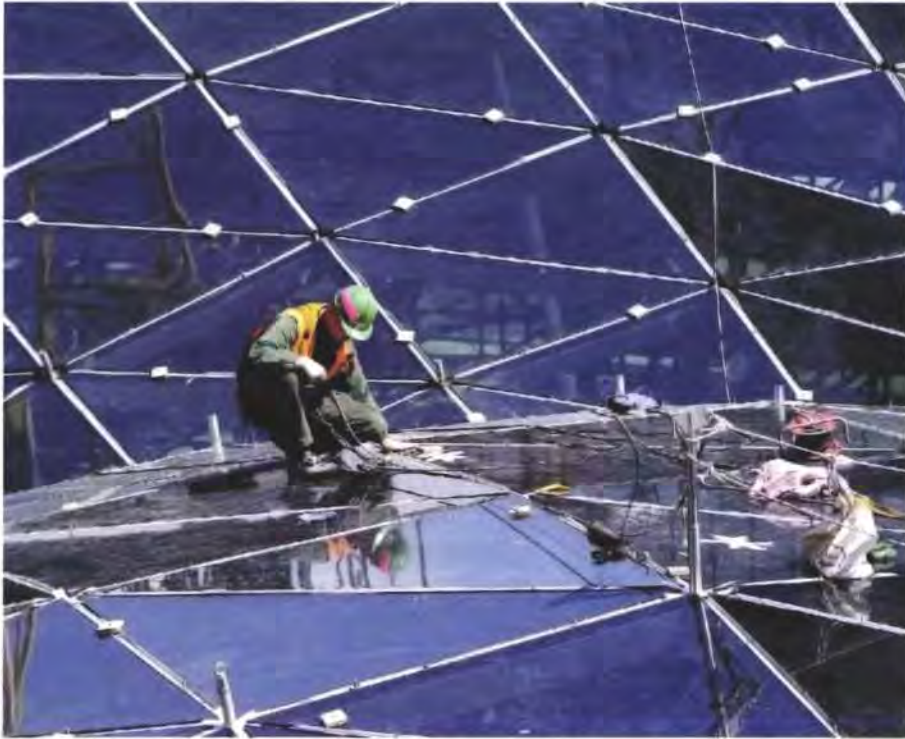
41. Glazing sealant installation.
