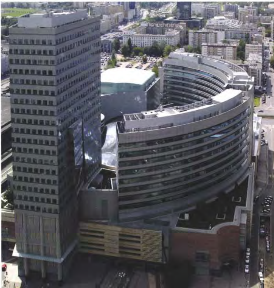
12. The "Skylight" office tower, the "Lumen" blocks and cinema from above.
