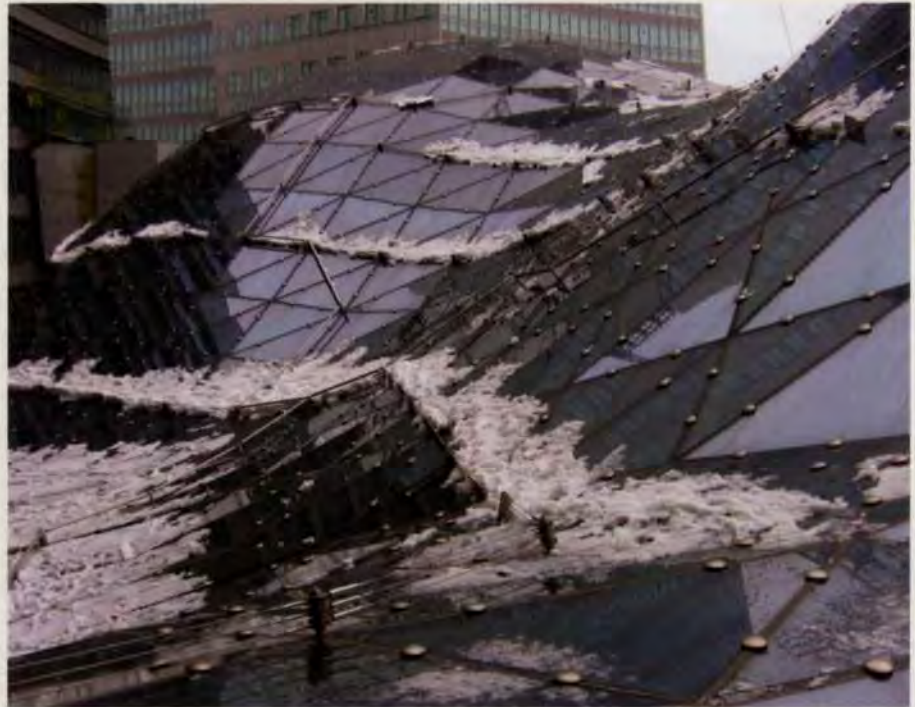
32. Snow retained on the roof by the snow fences.
