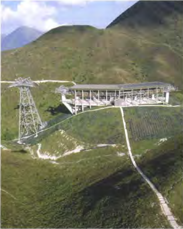
11. Nei Lak Shan angle station and Tower 4 slope reinstated after completion of stabilization works.
