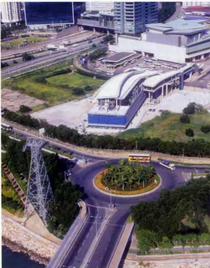
7. Tung Chung terminal building and Tower 1.
