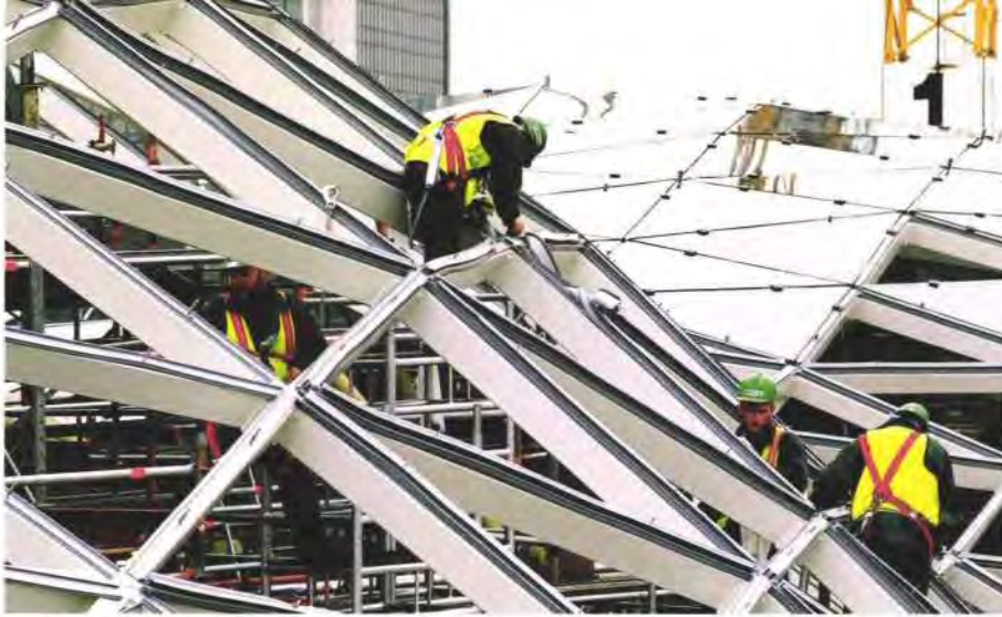
36. Glazing gasket installation.
