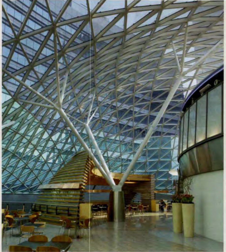
15. Internal view of atrium roof and the "Helmet" at the level 3 food court.
