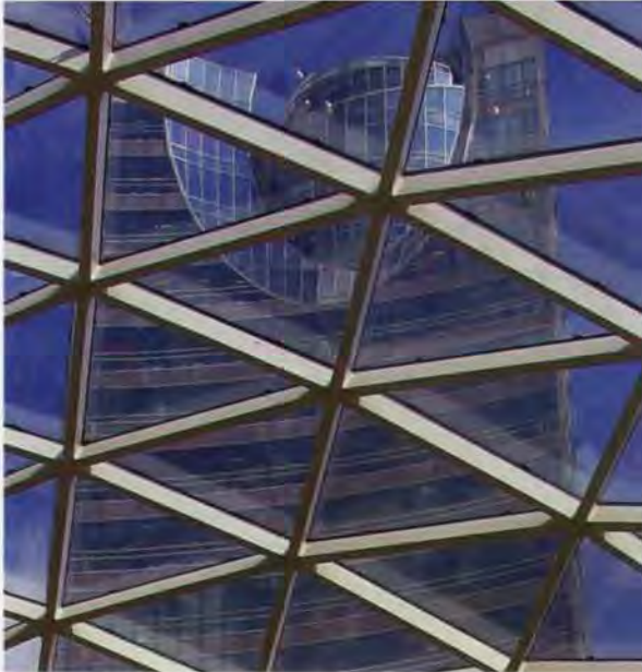
51. The "Skylight" tower through the atrium roof.
