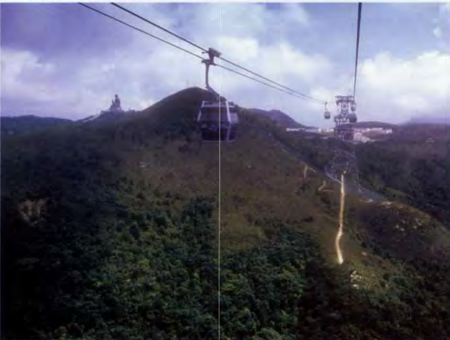
31. Cable car approaching Ngong Ping, showing the Tian Tan Buddha, Tower 7 and the rescue trail, with the theme village in the background.
