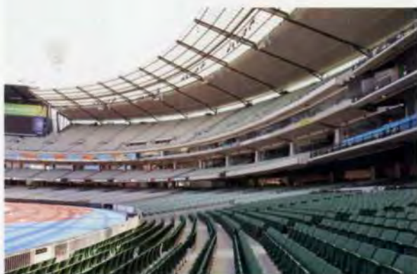
6. The extensive cantilever gives more spectator protection.
