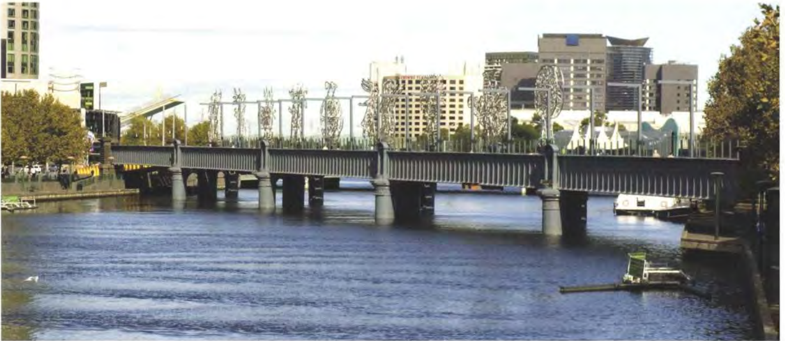
1. Sandridge Bridge with completed Traveller sculptures looking west over the Yarra River.
