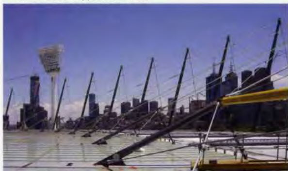
7. Cablenet supports to rafters.
