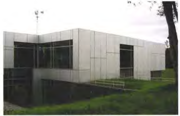
2. The new building is partially buried to further insulate against heat gains and losses.
