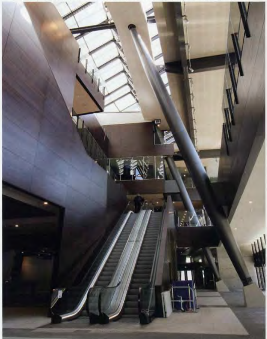
10. Sloping tapering steel columns also form part of the building's interior structure.
