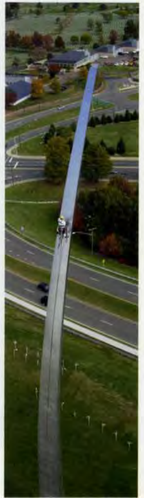
20. A cherry-picker is used to access the first access clip. The abseiler threads his rope through successive clips to prevent the ropes from sliding sideways as he ascends the curve of the spire.
