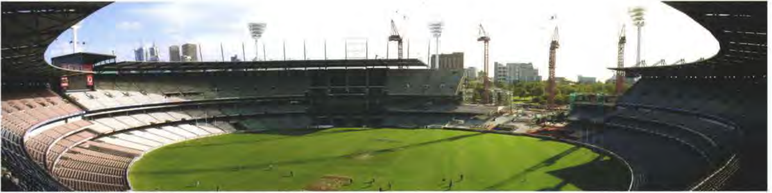
12. Construction progress, April 2006, including reinstatement of stabilized turf layer.
