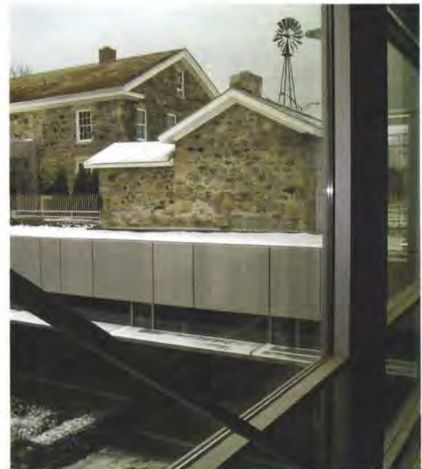
4. The historic farmhouse and sheds are integrated with the building and the site.
