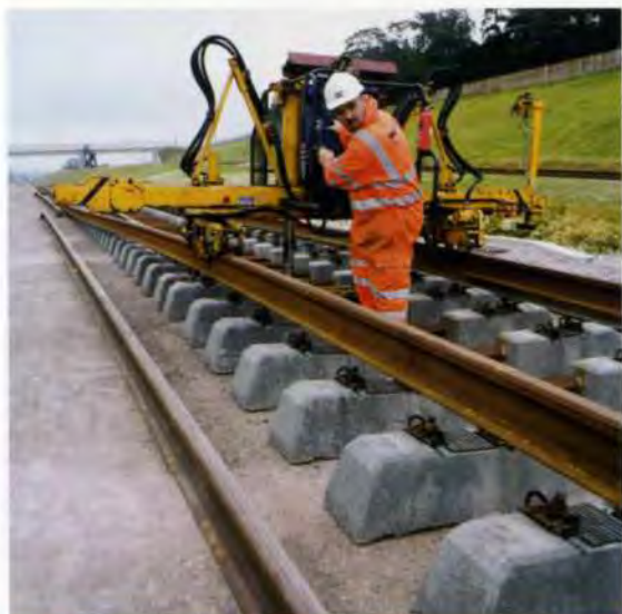
2. Installing long welded rail onto sleepers using a "rail threading" machine. 3 below: Installing permanent trackwork.
