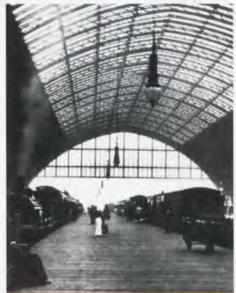
10. The original timber platform.
