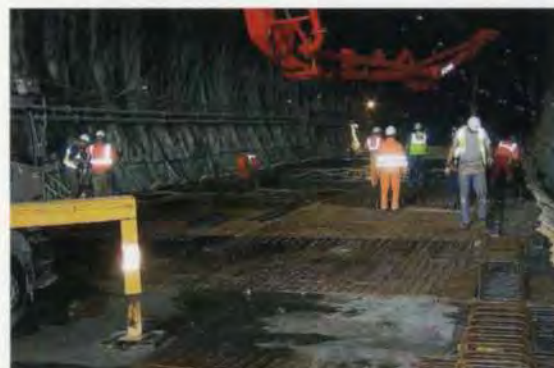
19. Reinforcement being fixed at the country portal.
