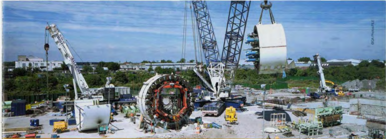
2. Tunnel boring machinery being prepared for driving the London Tunnels.
