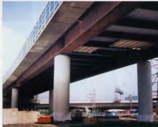
15. Choats Manor Way bridge, October 2001.
