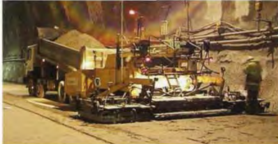
16. Paving machine laying the invert surface blinding.
