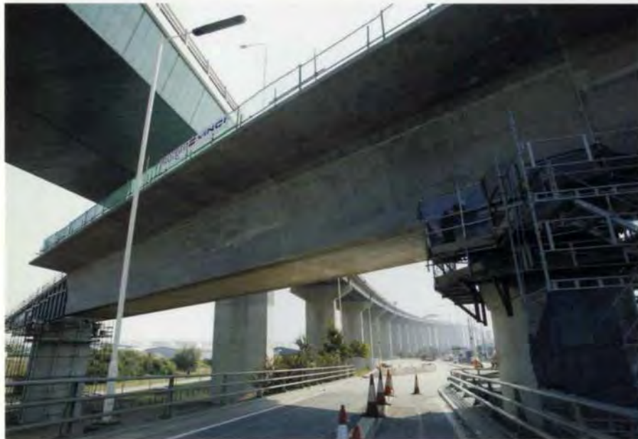
11. Thurrock Viaduct is push launched under the Queen Elizabeth II road bridge, July 2003.
