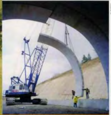
7. Eyhorne Tunnel arch being built.
