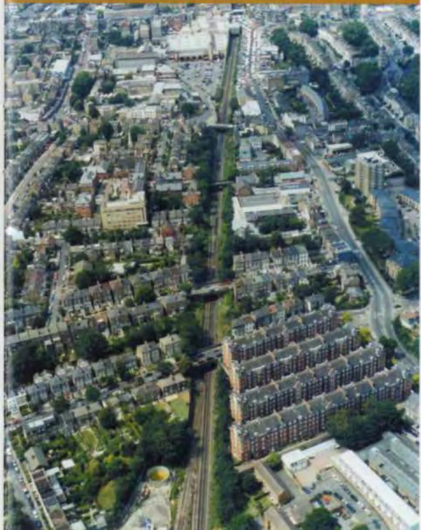
4. Aerial view of densely urbanized area, looking west along the North London Line with Dalston Kingsland bridge in the background and Navarino Road bridge in the foreground.
