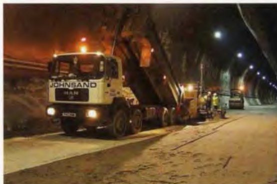
17. Surface blinding at the south (country) portal.
