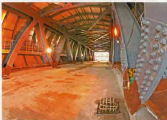
1-4. The East Coast Main Line bridge at the gateway to St Pancras was pushed into position during a single 55-hour possession of the ECML at Christmas 2003. Unusually on the CTRL, this is a covered bridge, for environmental reasons.
