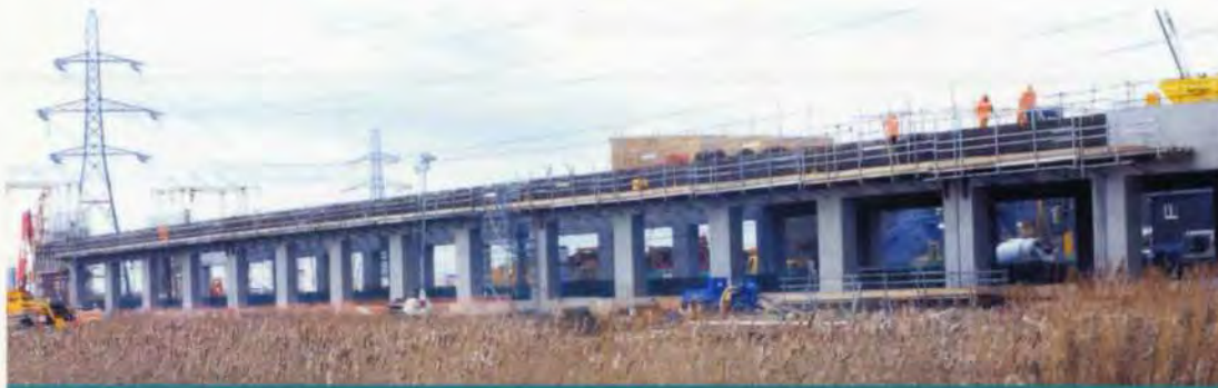
10. Aveley Viaduct crossover from marshes; under construction March 2004.
