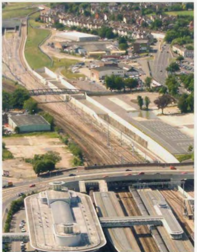
11. The two-track tunnel at Ashford International Station.
