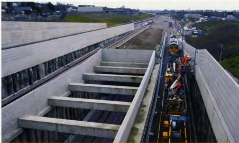
7. Track and catenary work at the start of the Ashford cut-and-cover tunnel.
