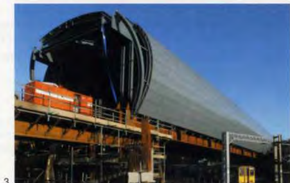
1-4. The East Coast Main Line bridge at the gateway to St Pancras was pushed into position during a single 55-hour possession of the ECML at Christmas 2003. Unusually on the CTRL, this is a covered bridge, for environmental reasons.
