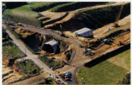
10. Sandway Tunnel precast arch.
