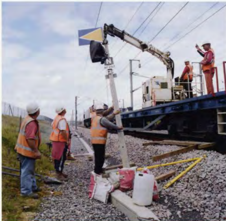
5. Installing a signalling mast (see p44).
