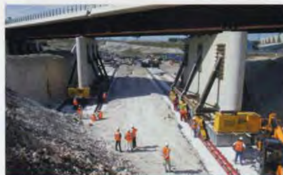
17. North Kent Line bridge being slid into position, May 2003.
