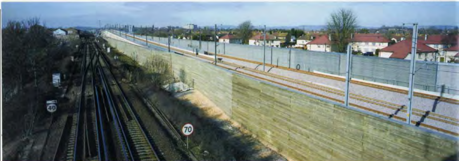
1. Acoustic fence protection on Section 1.
