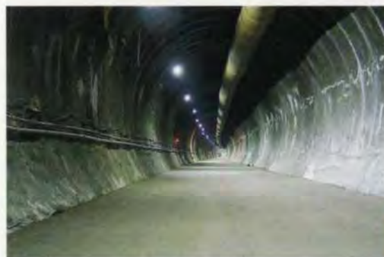
18. The completed tunnel invert after blinding.
