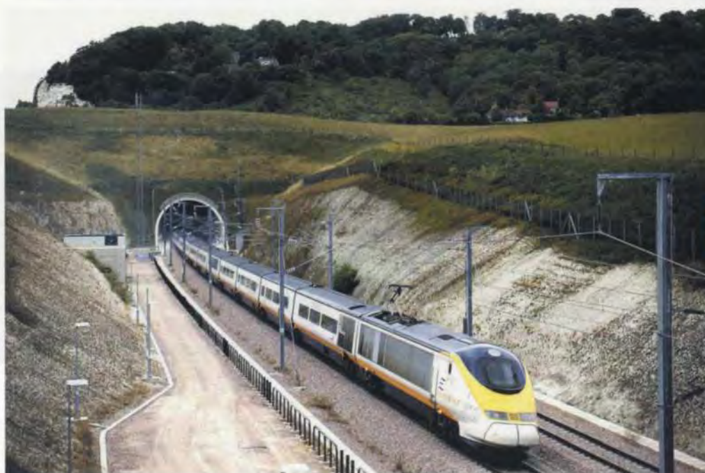
20. Eurostar exiting the North Downs Tunnel.
