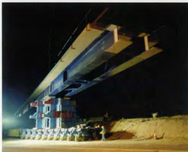
9. Steel composite: M20 rail bridge roll-out at Tutt Hill, between junctions 8 and 9.
