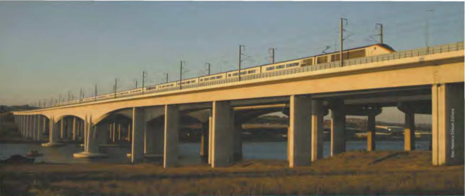
3. A Eurostar train in service on the 1.2km Medway Viaduct, the most prominent above-ground civil engineering structure on Section 1 of the CTRL.
