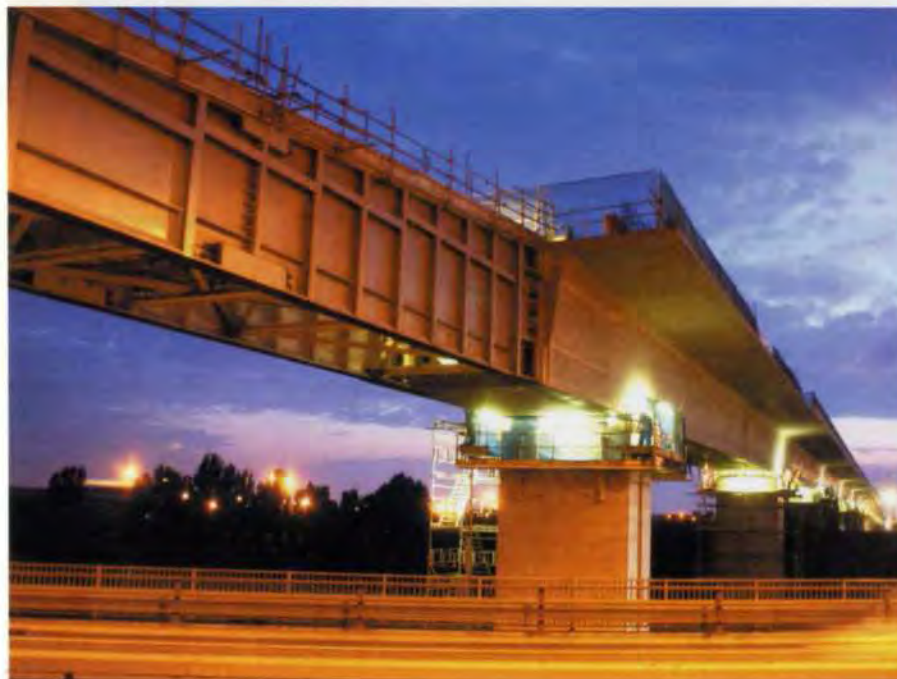
12. Thurrock Viaduct launched over major road at the Dartford River Crossing.
