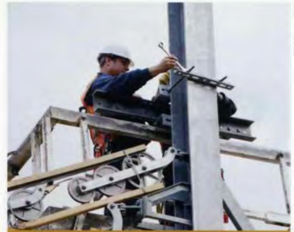
6. Installing OCS equipment.
