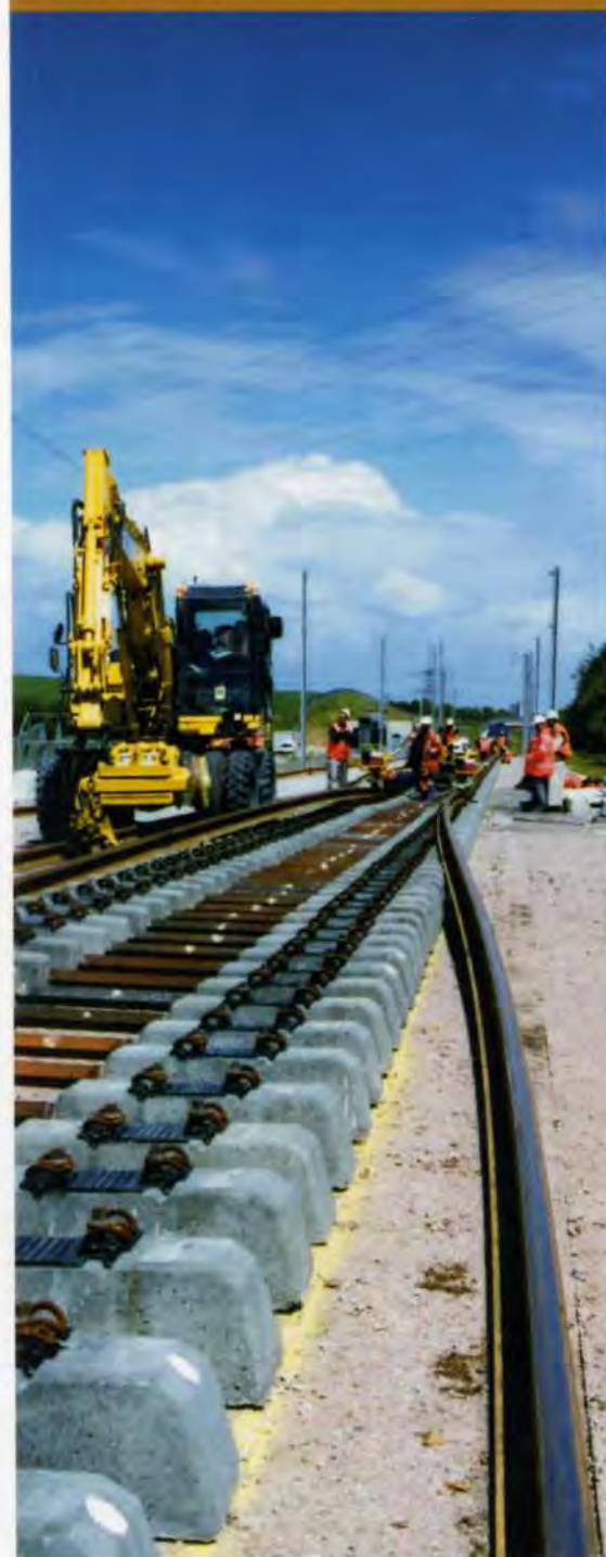
2. Installing long welded rail onto sleepers using a "rail threading" machine. 3 below: Installing permanent trackwork.
