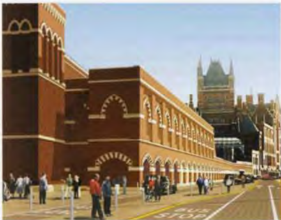
16. New east side building, looking south to St Pancras Chambers.
