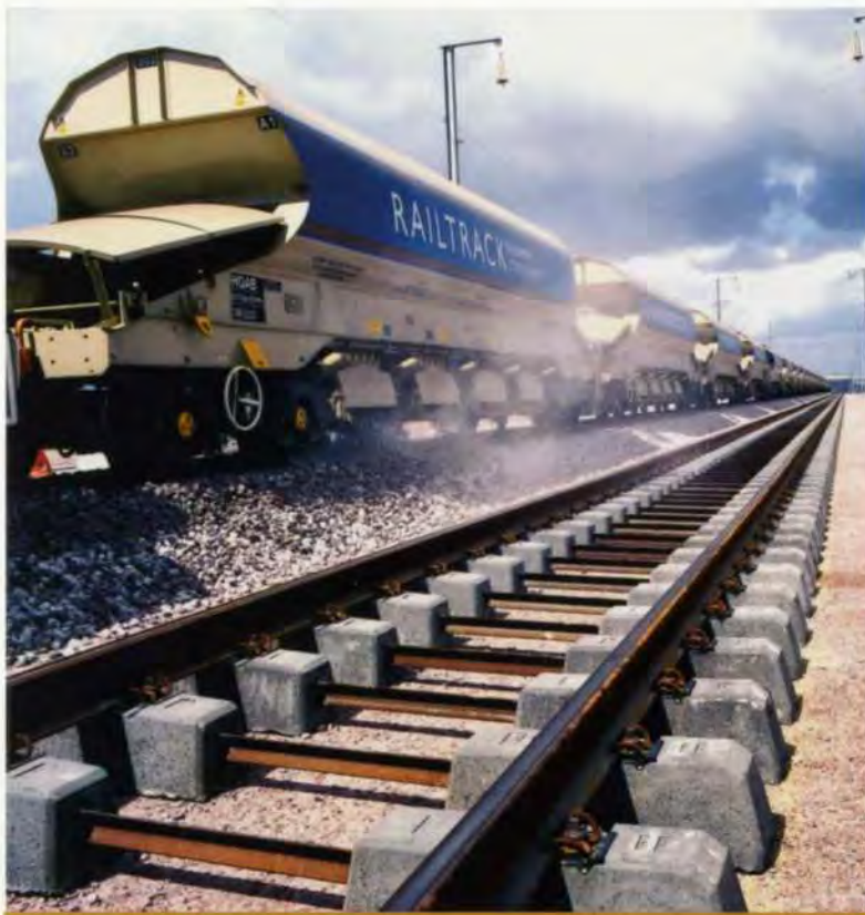
4. Laying ballast using remote control discharge wagons.
