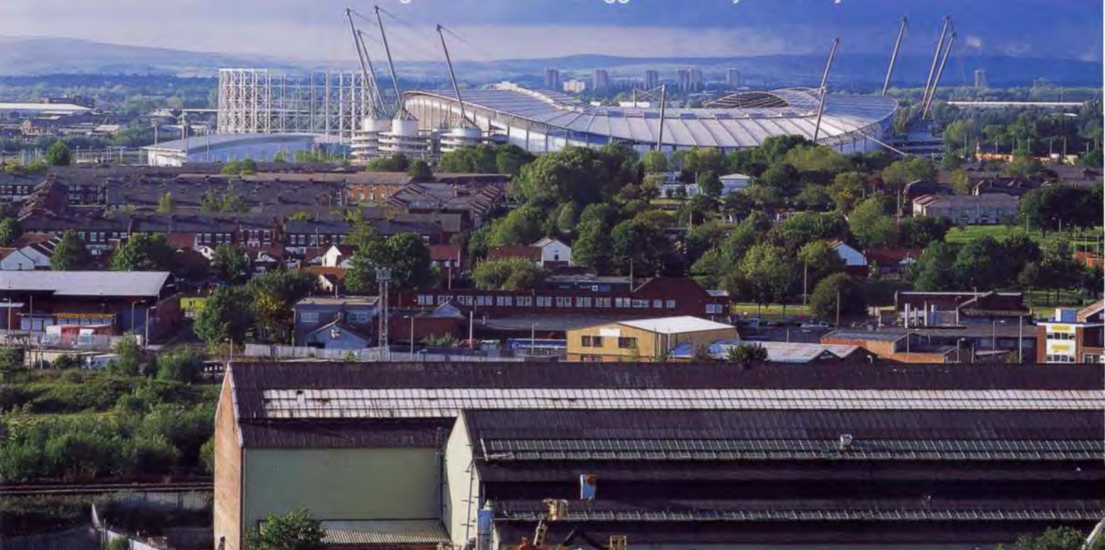
1. The City of Manchester Stadium in its Eastlands setting.
