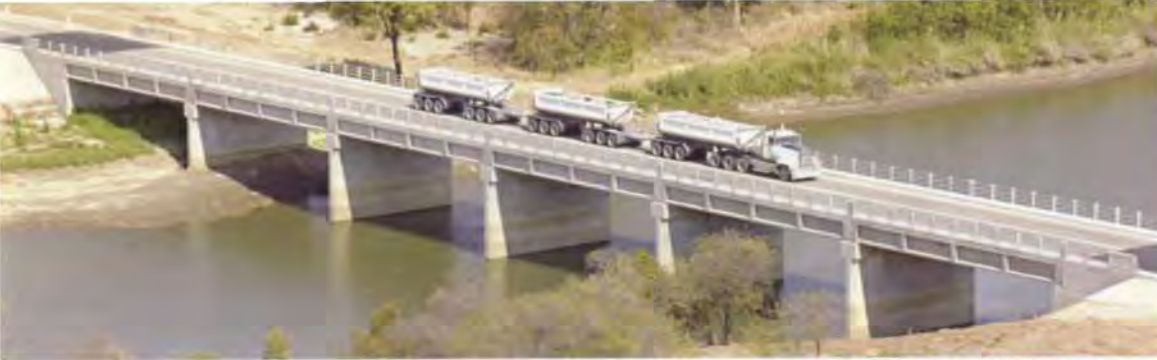
12. Mupfure River Bridge: 112m long with precast concrete beams and cast in situ slab. This method cost more than the traditional cast in situ beam and slab, but was faster and did not require staging in the potentially flooded river bed.
