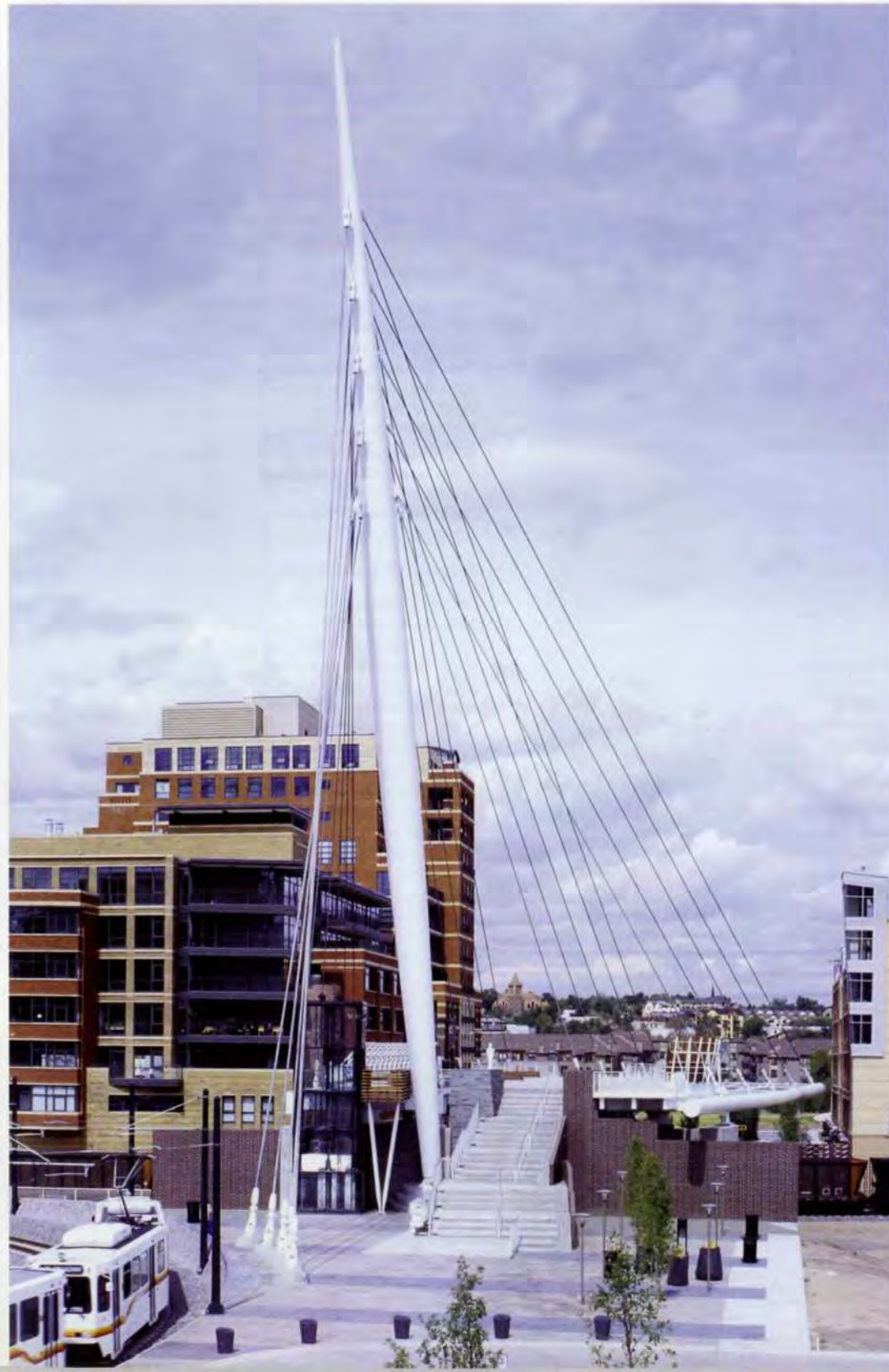
8. The bridge viewed from the city.
