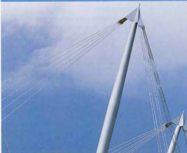
Mast top detail: 11 above: as designed; 12 below: as built.
