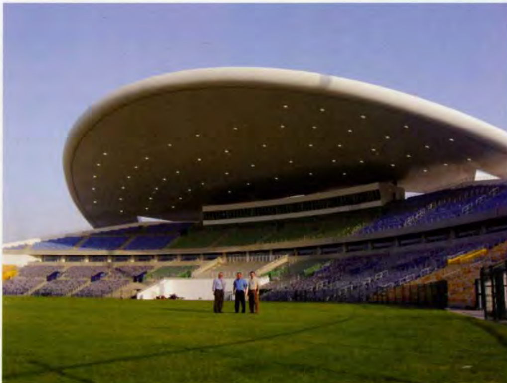
7. The completed roof in position.
