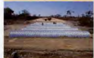
8. Six-bore Armco multiple culvert.
