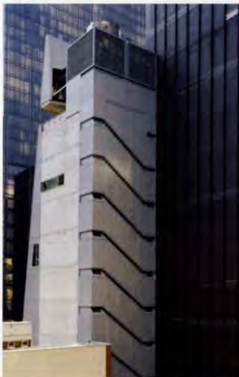
9. Staircase with water tower above, ventilation louvre at each side, and cooling tower louvred enclosure.
