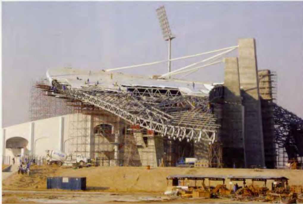
4. Cladding in progress, closely behind erection of the steel.
