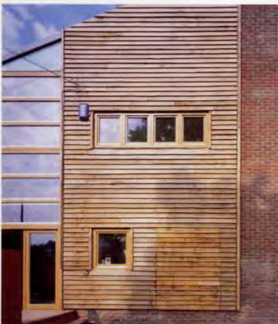
10. Use of materials: triple-glazing + locally-sourced untreated oak cladding + local brick.
