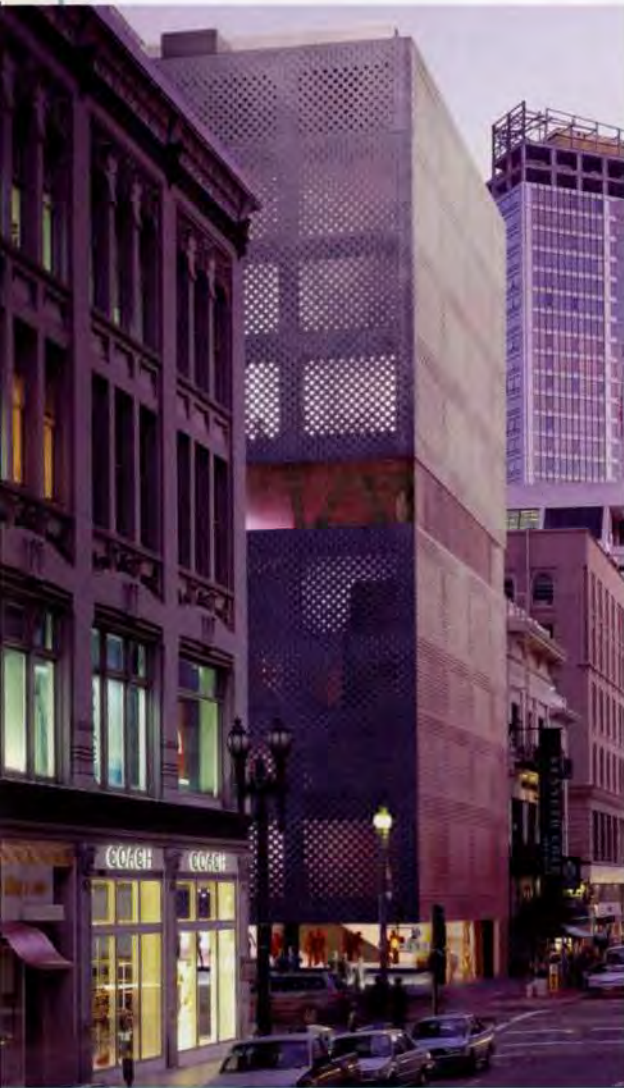
8. San Francisco: a 13-storey retail store (providing 22 000ft 2 (2040m 2 ) of retail and office space) with a unique structural system of base cantilever and perforated steel shear panels to resist lateral forces.
