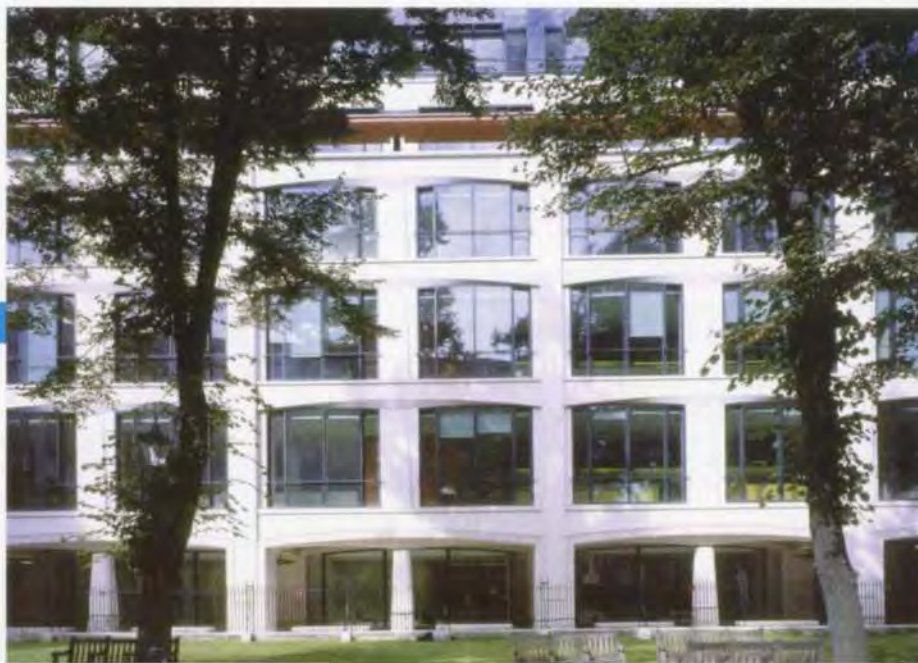
11. Main building façade.
