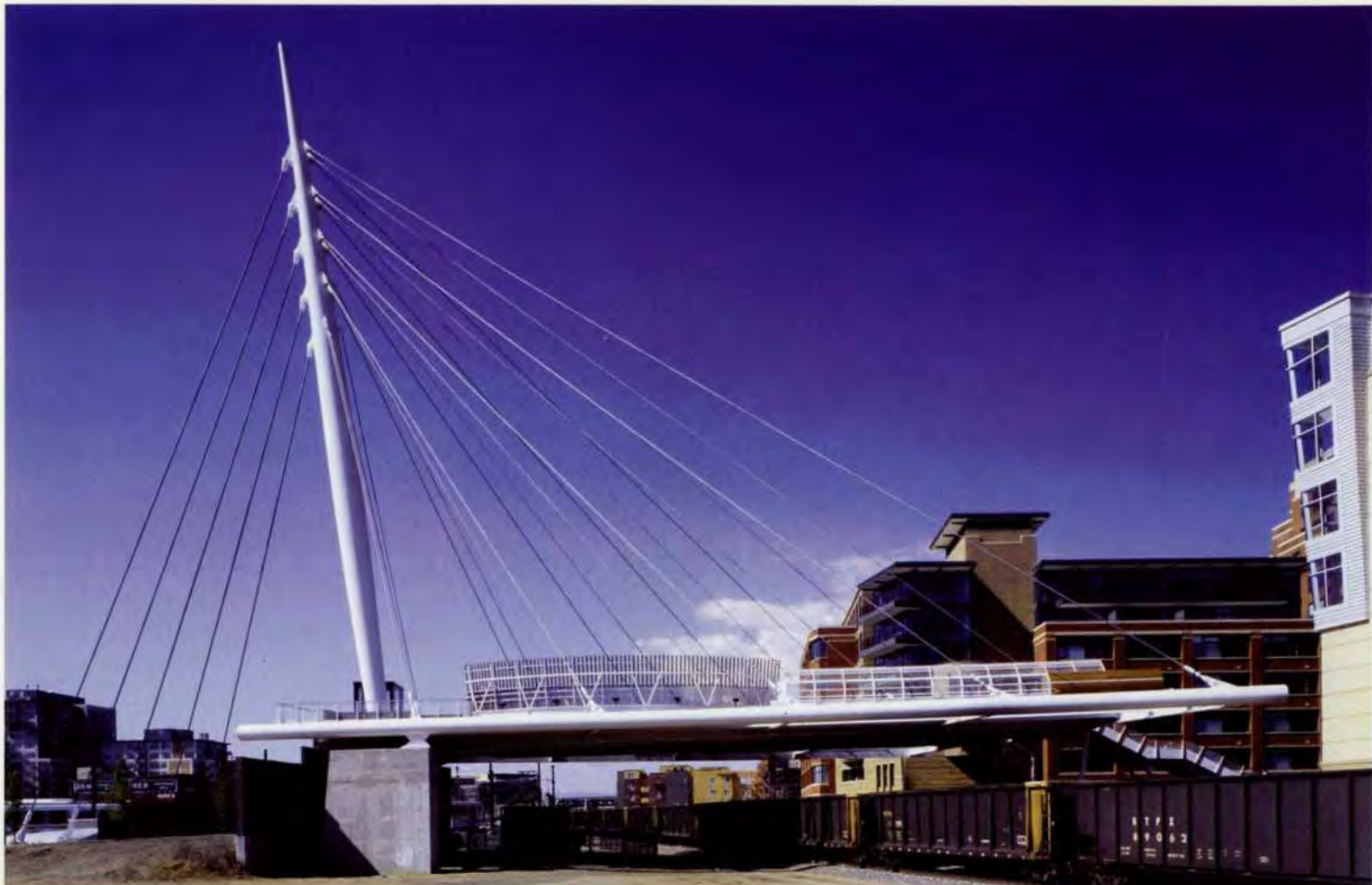
4. Side view from the north, showing the bridge crossing the consolidated main line railroad tracks.
