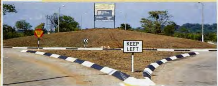
4. Roundabout crossing with main Harare/Bulawayo road raised centrally to prevent glare from oncoming vehicles. This requires street lights for 24-hour operation.
