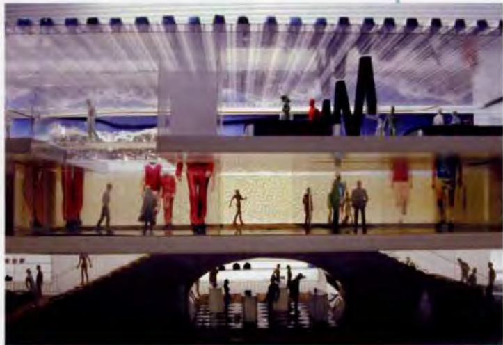
10. Beverly Hills: The unique system provides column-free spaces as well as the full 110m wide floor and has a steel moment-resisting steel structure. The building began construction in January 2003.
