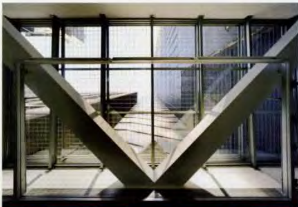
4. View from atrium, looking up through glass roof, of north vertebrae façade.
