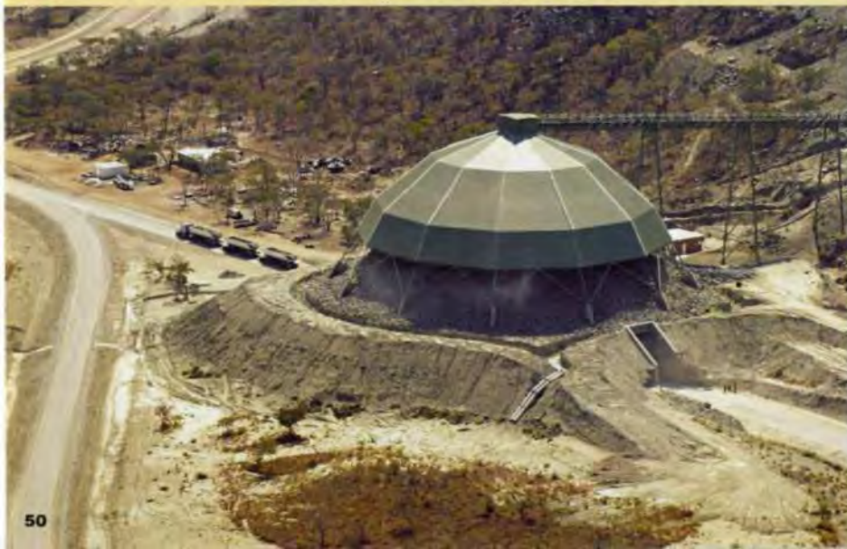
5. Ngezi mine load out dome and tunnel, with crusher to the right. A full 152 tonne road train on the left begins its 77km trip to the SMC.
