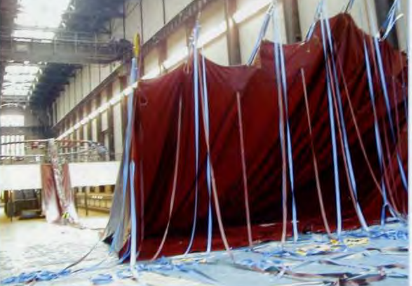
8. Raising membrane at east end.
