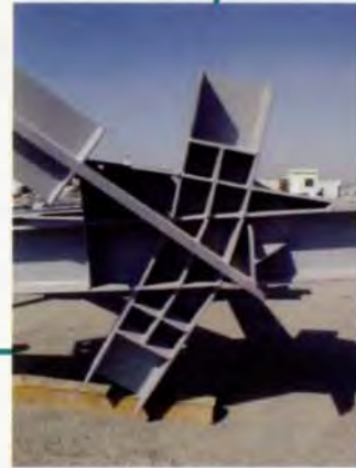
6. Truss intersection node.
