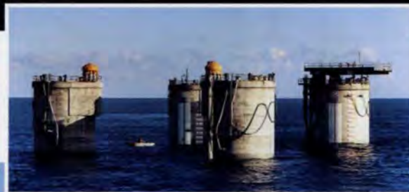
11. The CGS fully submerged in position awaiting topsides.
