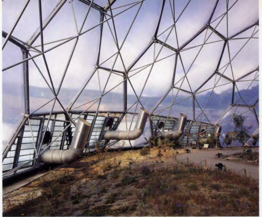
8. Air outlets in the Warm Temperate Biome.
