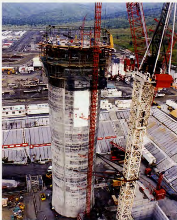
4. Utility shaft under construction, October 1999
