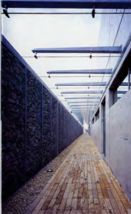
13 left: Exterior corridor, the long gabion wall is on the left.
