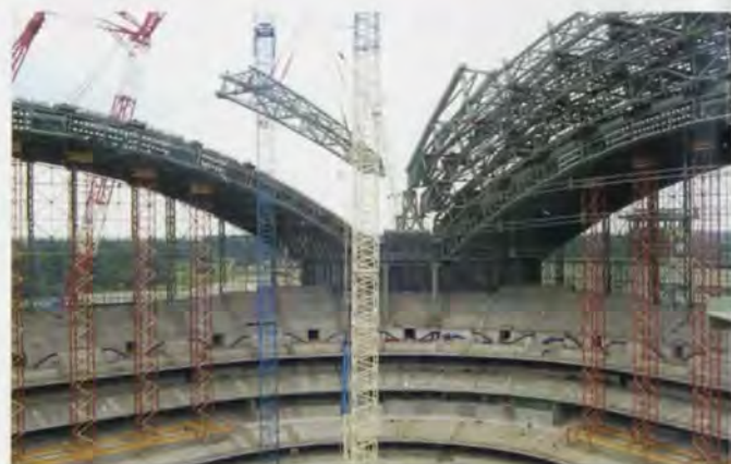
10. Block erection.
