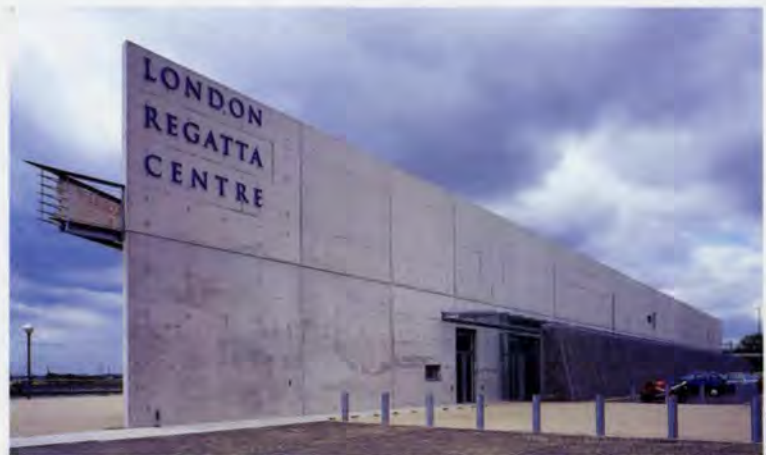
4. Main entrance, with gabion wall on right.
