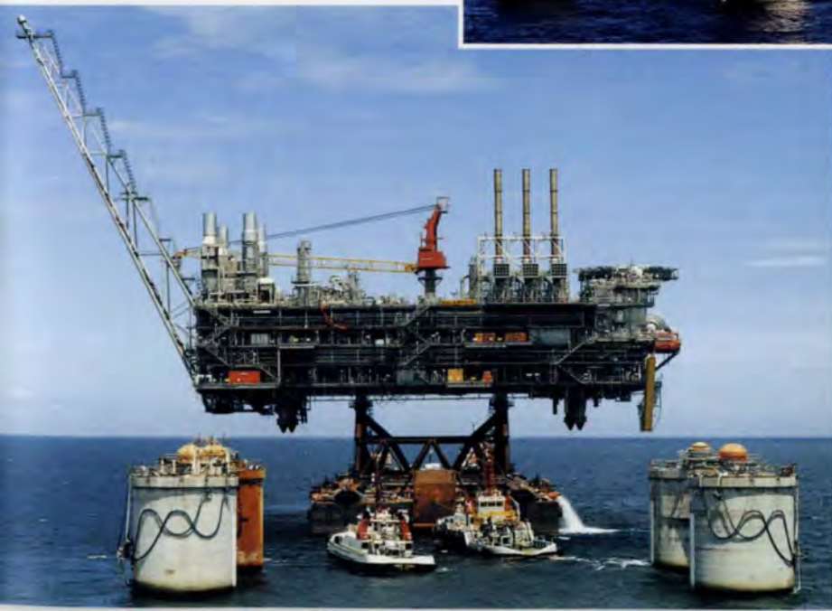
12. The topsides approaching the CGS for installation.
