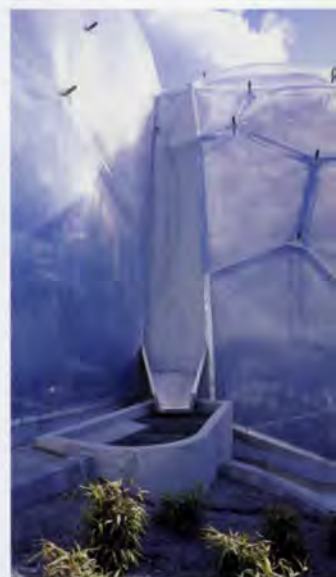
20. Typical rainwater collection point.
