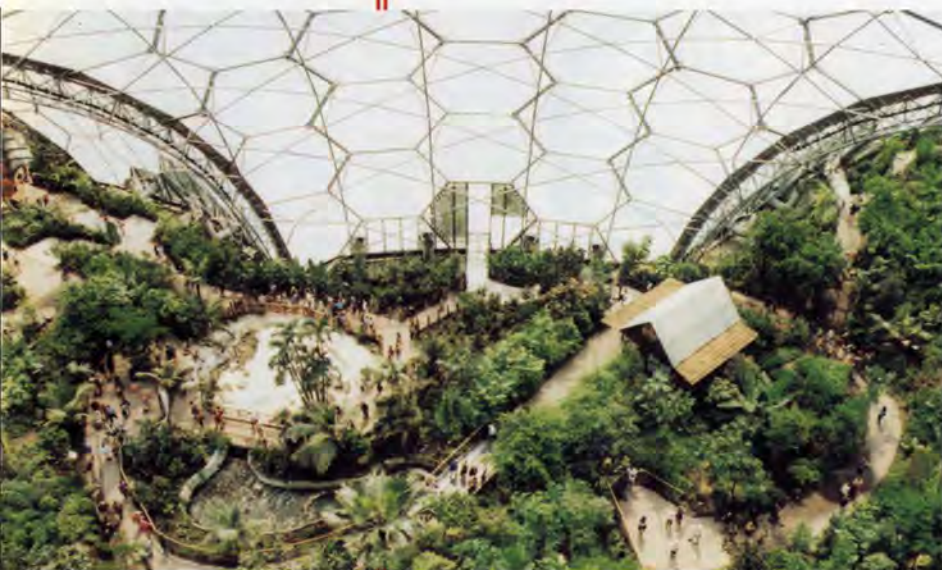
18. Interior of Humid Tropics Biome, showing distances involved for escape in case of fire.
