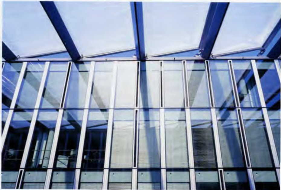
2. The façade, the atrium, and the PTFE roof (open).
