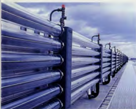
12. Roof-mounted solar panels providing solar water heating.
