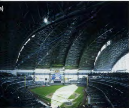
4 a) to e) below: Opening the roof.
