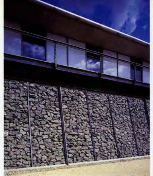
10. Part of the line of gabions along the clubhouse.
