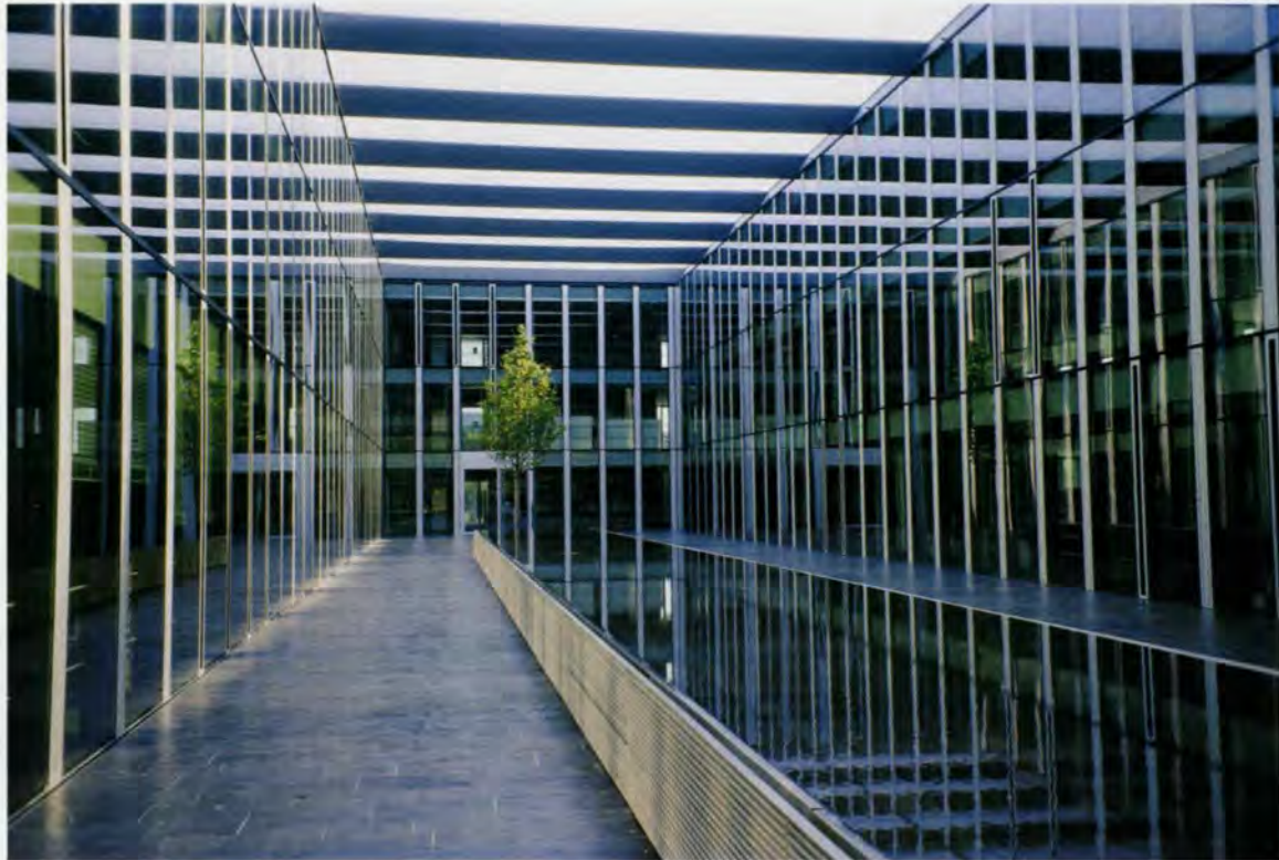
11. The central atrium, showing the air supply grilles from the underground ducts beside the water feature.
