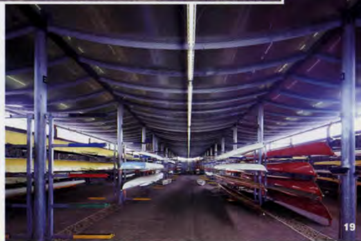
5. The boathouse with its catenary roof, and racks supporting 20m boats needing level storage.
