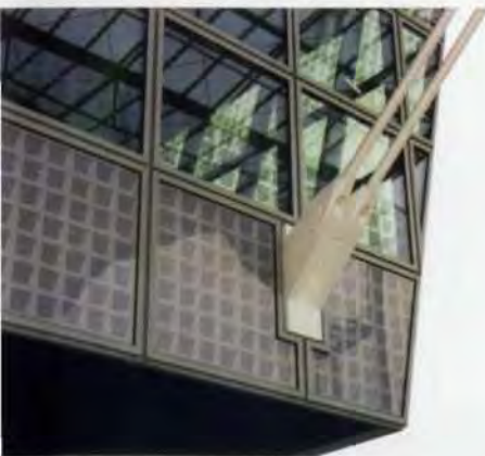
6. Backstay connection to building.
