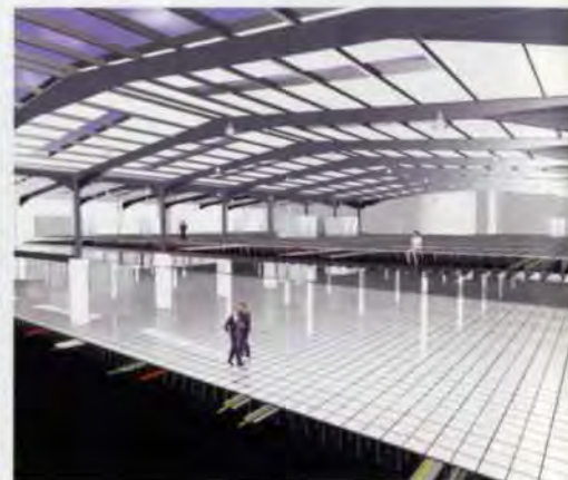
4. Cut-through of typical datacentre
