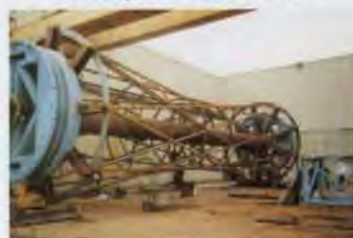
1. Assembly of structural 'sleeve'.
