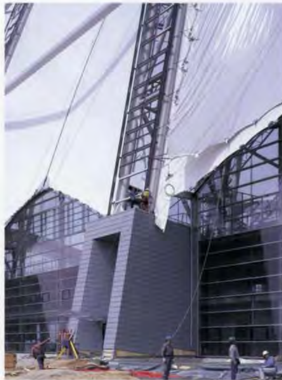
5. One of the building's two main parts: the steel arch-supported, fabric-covered bays. The arches spring from concrete plinths which also act as covered entrances giving protection against snow avalanches.
