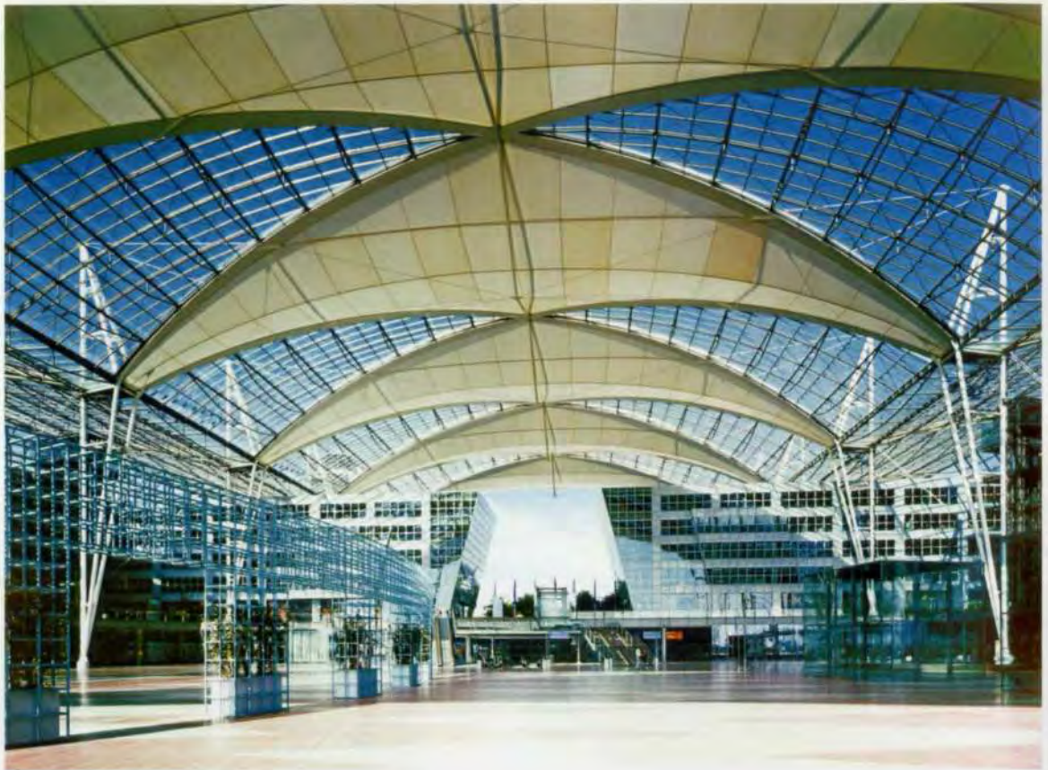
9. The roof seen from the Forum space along the central axis; the main entry platform is at the far end.
