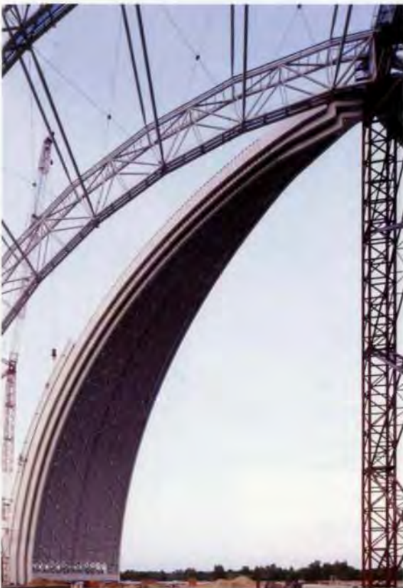
15. Near the ridge the perfect match of the z-shaped doors is clear.
