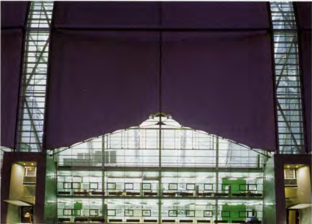
16. The two-storey office building between the concrete bases of the hangar's arches.
