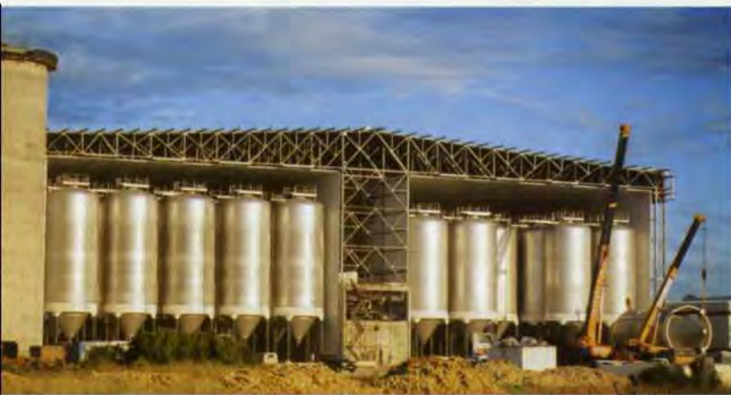
6. Cellar building at completion of tank installation.
