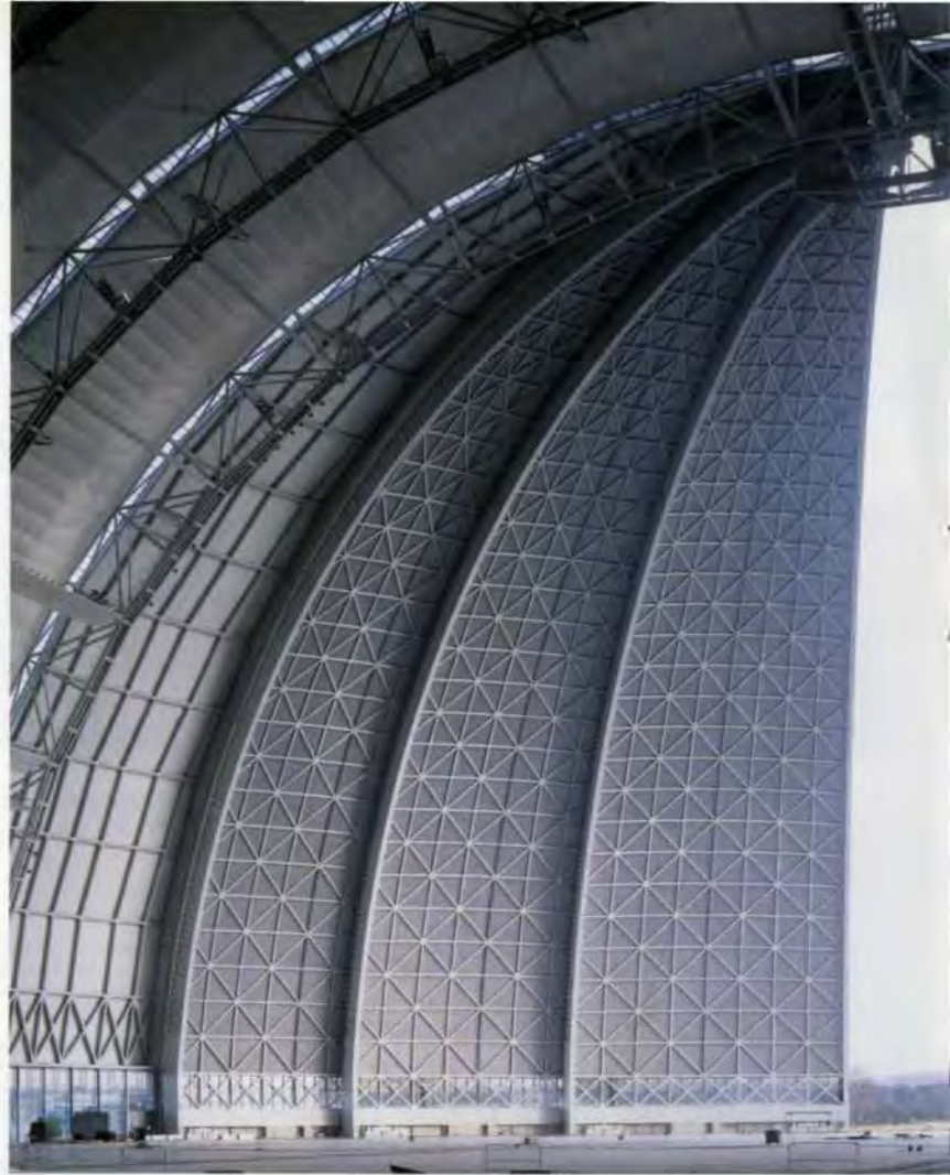
14. On opening, the door segments nest inside each other.
