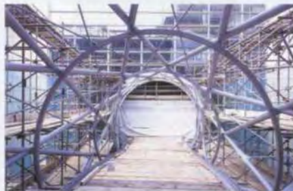
4. Tubular sleeve and alternating rods in place.
