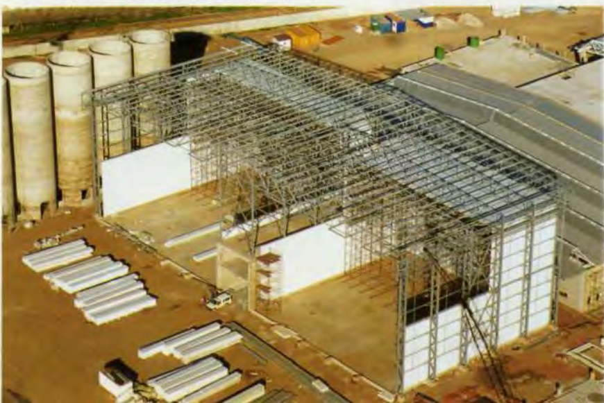
7. Cellar structure's insulated paneling partially completed.
