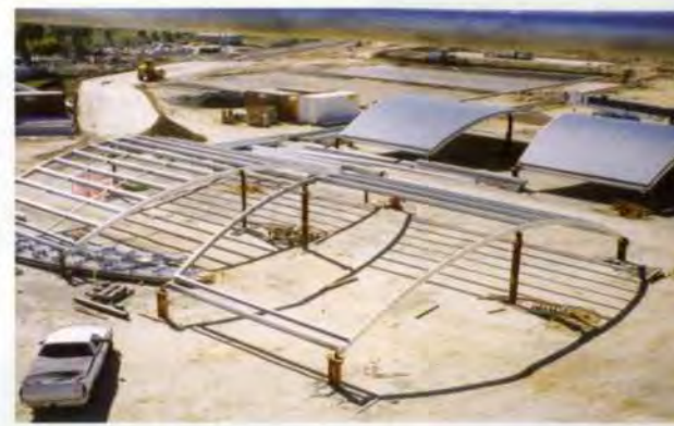
11. Roof panel prefabrication.
