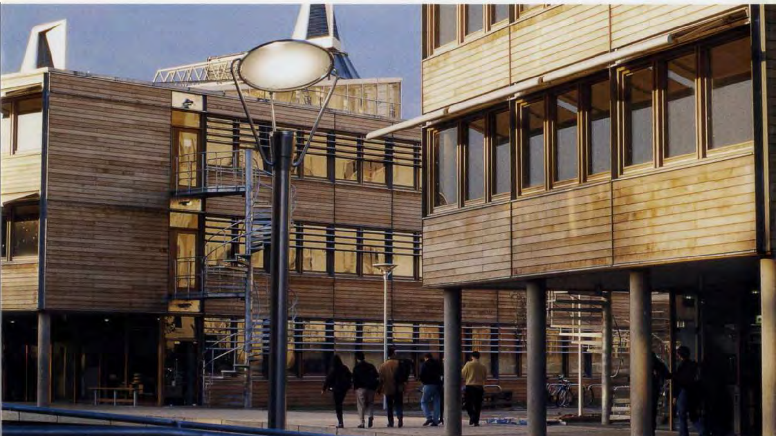
14 below: Looking past the Central Teaching facility to the School of Management and Finance; note light fixture - designed by Arup.
