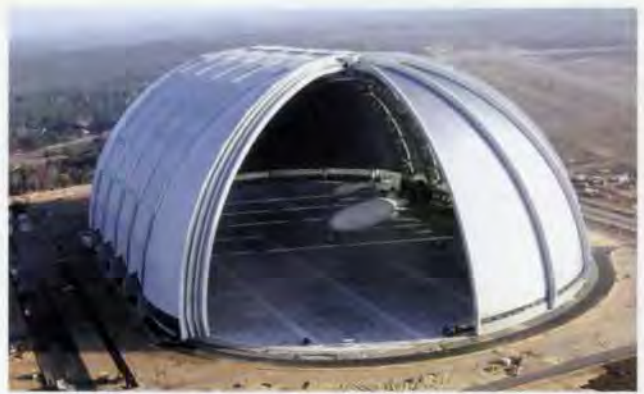
4. The clam shell doors slide underneath each other, opening the hangar to the outside world. Inside, small versions of the CargoLifter are visible.
