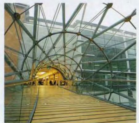
5. Interior towards Arndale Centre.
