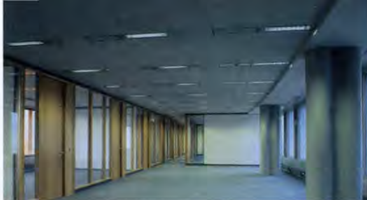
12. Linear fluorescent fittings provide artificial lighting for the offices.
