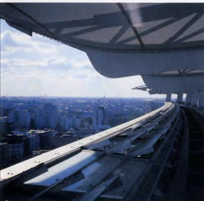
4. View from the roof of the tower with the top of the thermal flue in the foreground.
