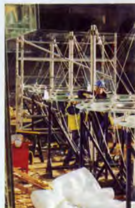
2 right. Beacon units prior to assembly
