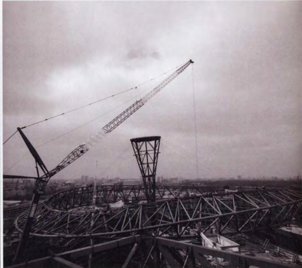
(c) Prefabricated kingpost supported in scaffolding.
