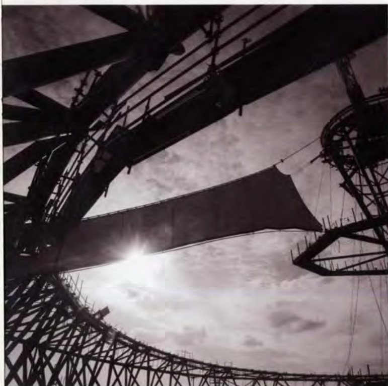
(d) Fabric segments being craned into position.
