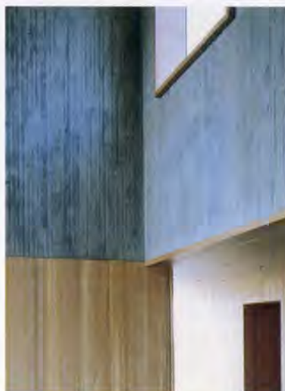
2. Timber cladding with boardmarking above.
