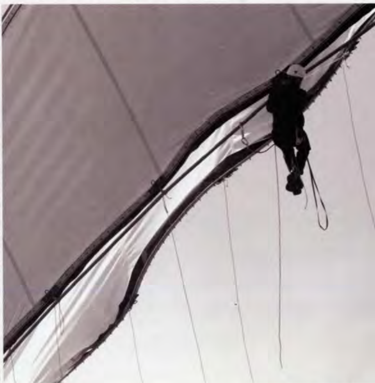
(e) Fabric segment being connected to ridge and valley cables.
