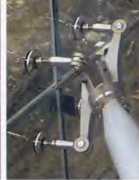
8. Detail of the wind star showing double-pinned struts.
