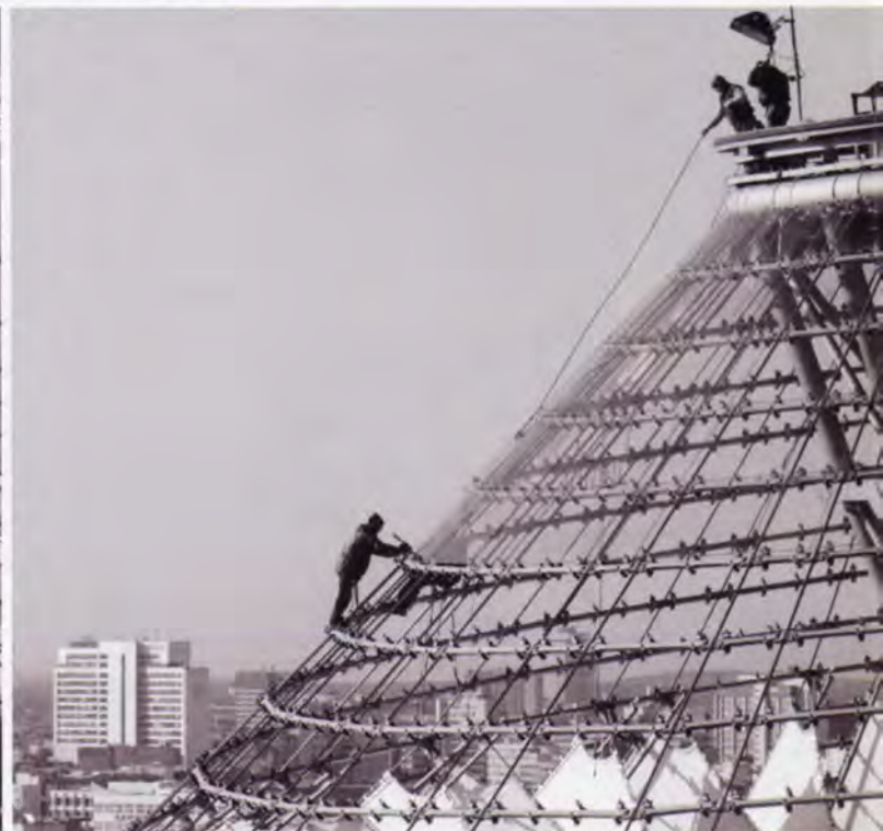
(k) Installation of the glazing.
