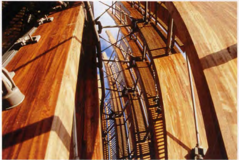
6. Detail of structure.
