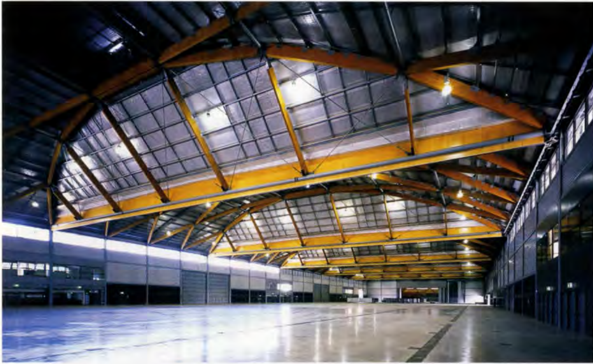
3. Circular vault roofs to the rectangular halls.
