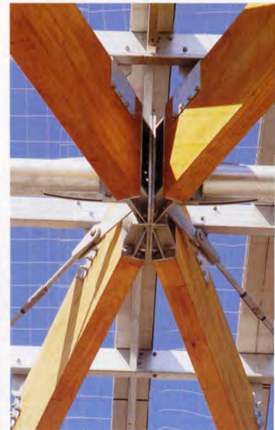
12. Typical end-plate bolted joint to vault framing.
