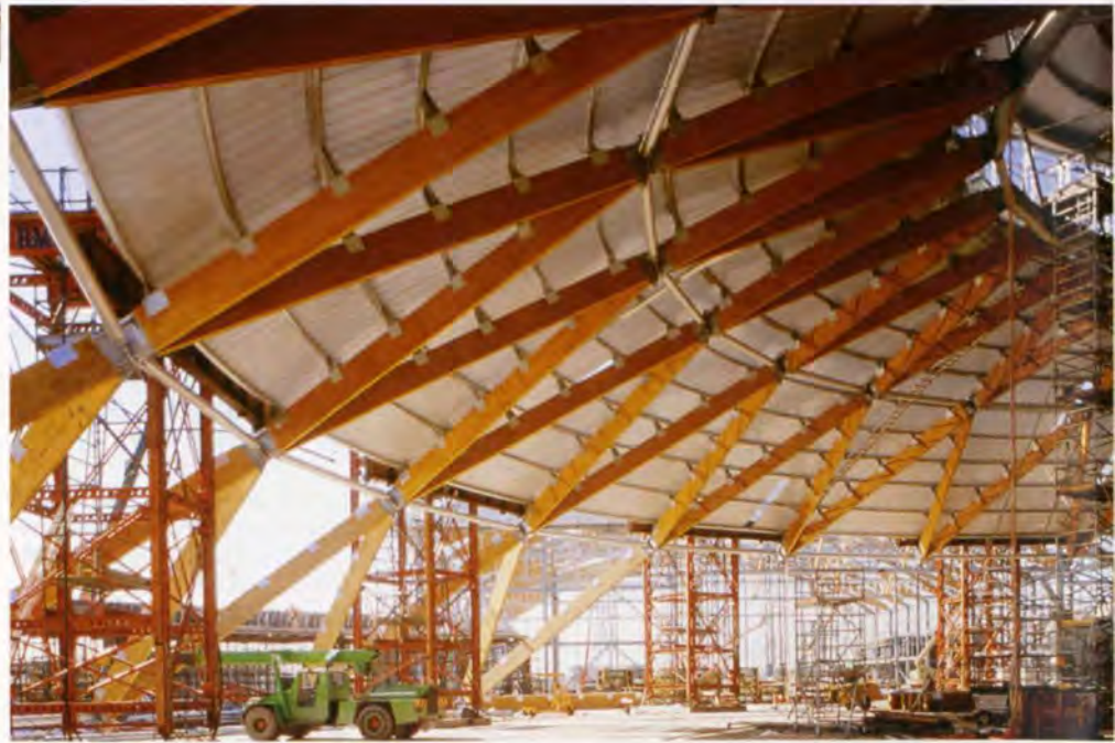
7 below: Partly completed dome suspended from jacking towers.
