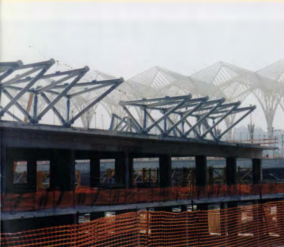
4. Tetrahedron units being erected on site.
