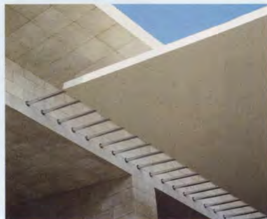
9. Cable attachment of canopy.
