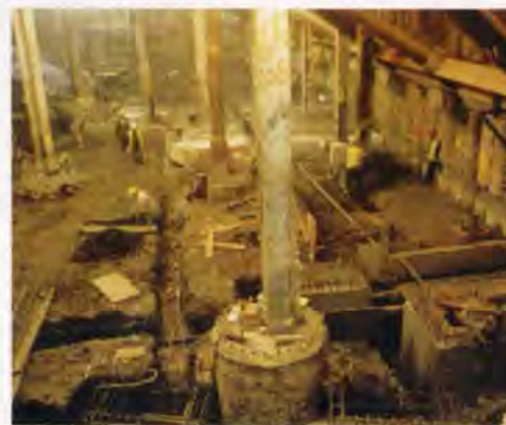
8. Top-down construction under way in the basement, October 1996.
