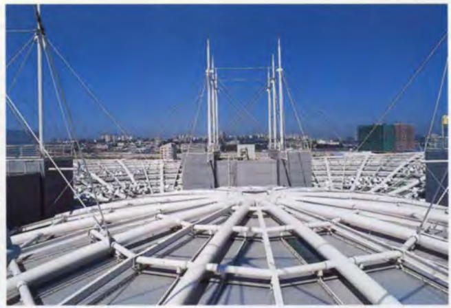
4. Detail of roof structure.
