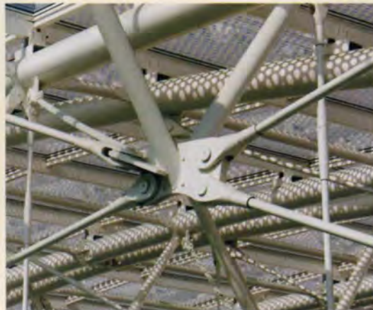
5. Junction of Macalloy bar and tensioned rod components.
