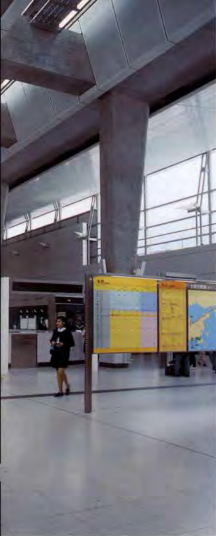
7 left: The concourse from the west: roof soffit and side cladding to central rooflight are perforated metal acoustic panels.
