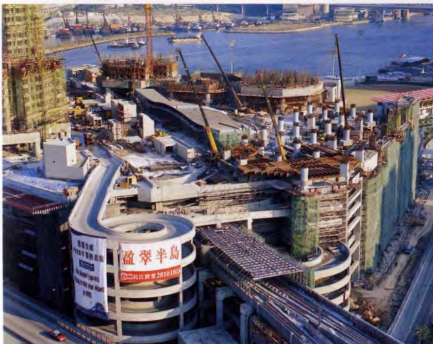
7 right: Residential tower development under construction. Along the northern elevation, adjacent to Tsing Tsuen road, a 300m long, 12m wide cantilever noise canopy framed in structural steelwork is provided to lessen the effect of traffic noise on the residential towers above.
