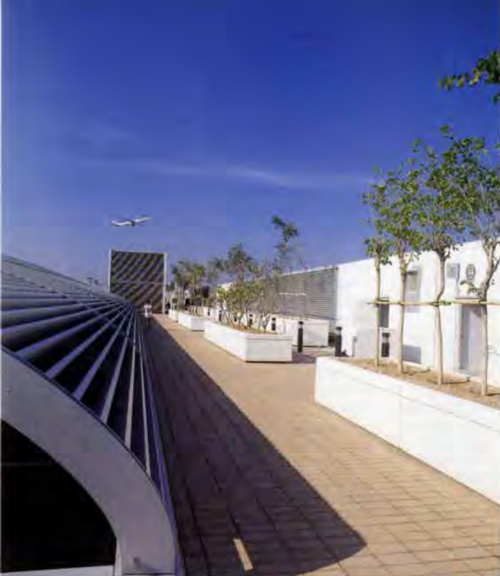
16. Part of roof garden.
