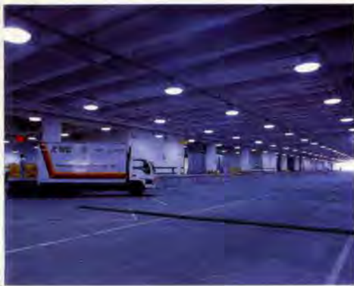
15 Truck dock area in Terminal.
