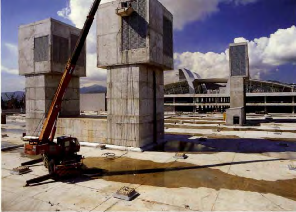
7 above: Podium deck directly above Station box, with Station entrance beyond. Stub columns with couplers for future development can be seen in the foreground. The railway ventilation shafts are constructed to their final level so as not to cause disruption when more development decks are built around them.
