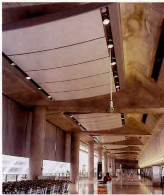
8. Sound-absorptive roof at Airport Terminal Building.
