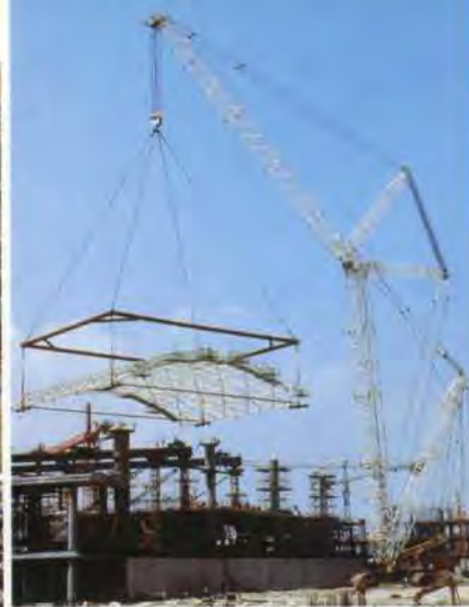
13. Erection of a roof module, summer 1996.
