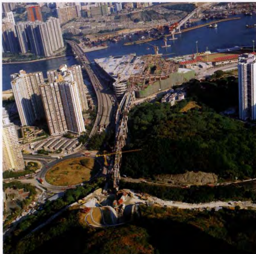
5. The Station podium and viaducts during construction.
