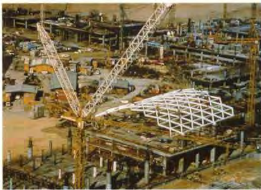
12. The first roof module being lifted into place, December 1995.
