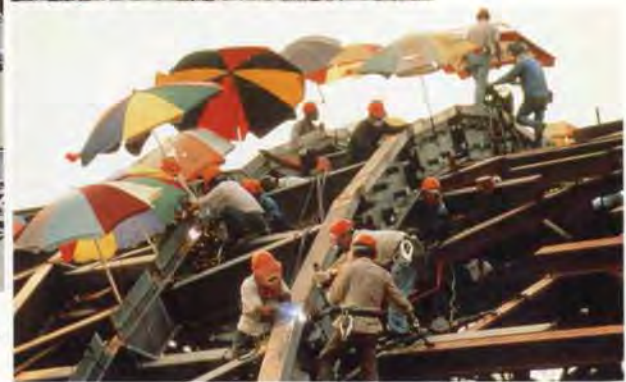
15. On-site fabrication of roof modules.
