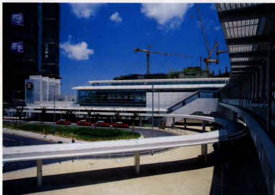
3. Main station entrance area viewed from footbridge; MTRC developments under construction left and behind.
