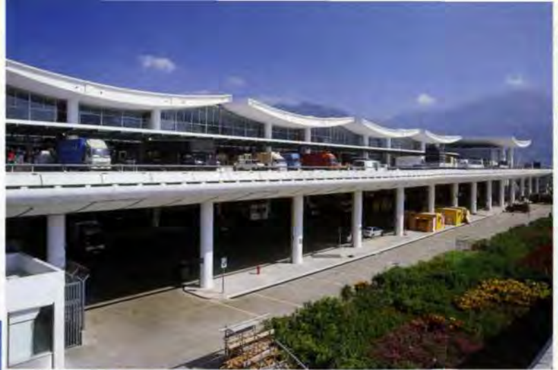
13 above: West façade of Express Centre.
