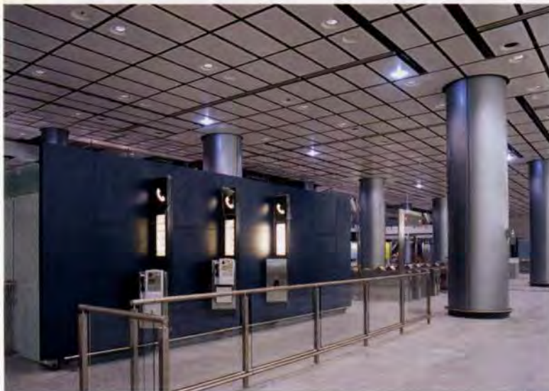
2. Flat panel ceiling over Hong Kong Station's Airport Express Line concourse.
