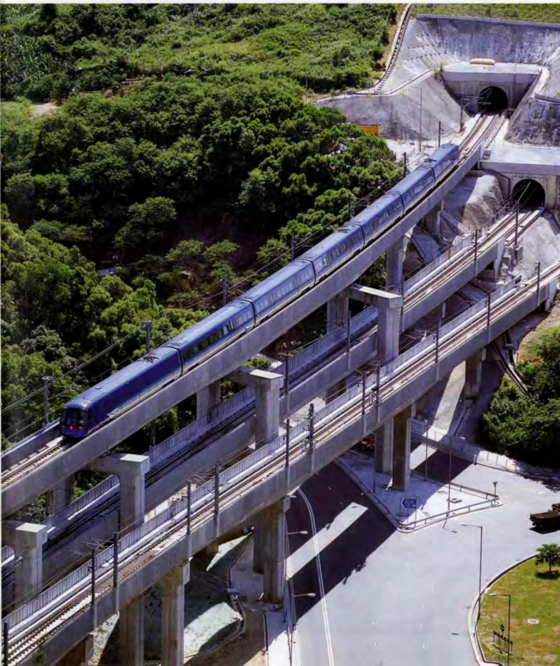
16. Viaducts crossing Tam Kon Shan Interchange with Airport Express train.
