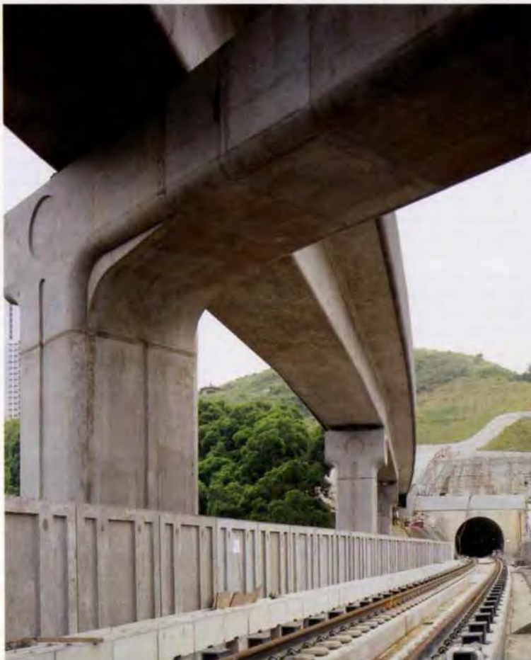
14. Pier details of viaduct near tunnel portals.
