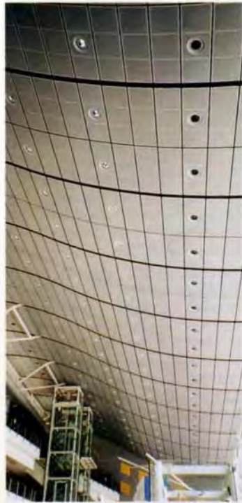
1 left: Curved ceiling panels above the main entrance of Hong Kong Station's in-town check-in Hall.
