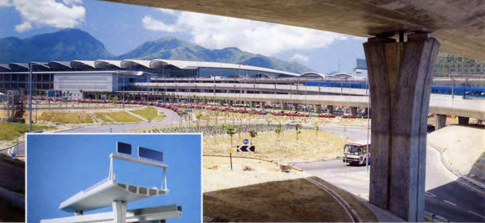
4 left: Model showing the differing cross-sections of the highway viaduct and railway viaduct.
