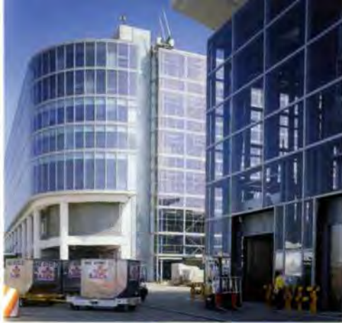
11. Entrance to dolly train lift in Express Centre (right foreground).
