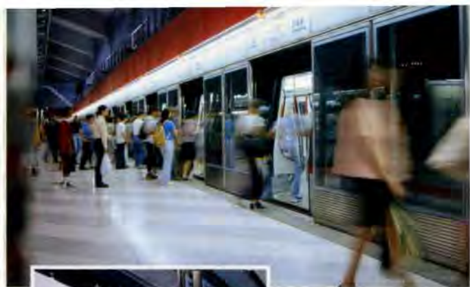
4. PSDs in use on TCL platform at Lai King Station.
