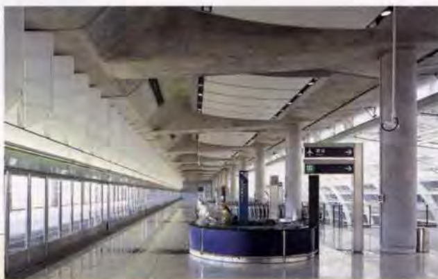
6. Platform for Airport Express trains arriving from Hong Kong.
