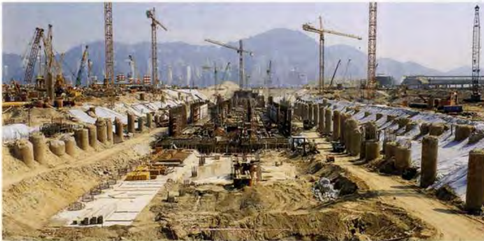
5. Station excavation complete, with TCL base slab and perimeter retaining walls under construction. Bored piles exposed by the open cut excavation can be seen either side of the box.
