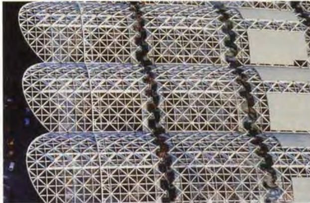
14. Roof modules in processing building awaiting infill elements and de-propping.
