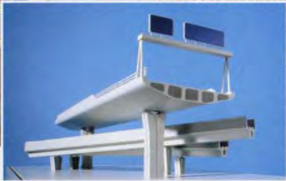
4 left: Model showing the differing cross-sections of the highway viaduct and railway viaduct.
