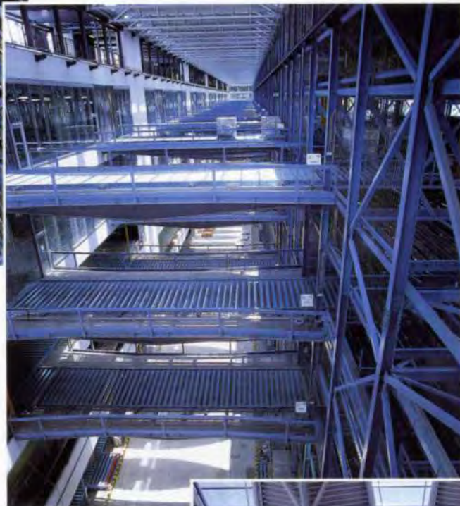
7. Roadway viewed from upper bridge.
