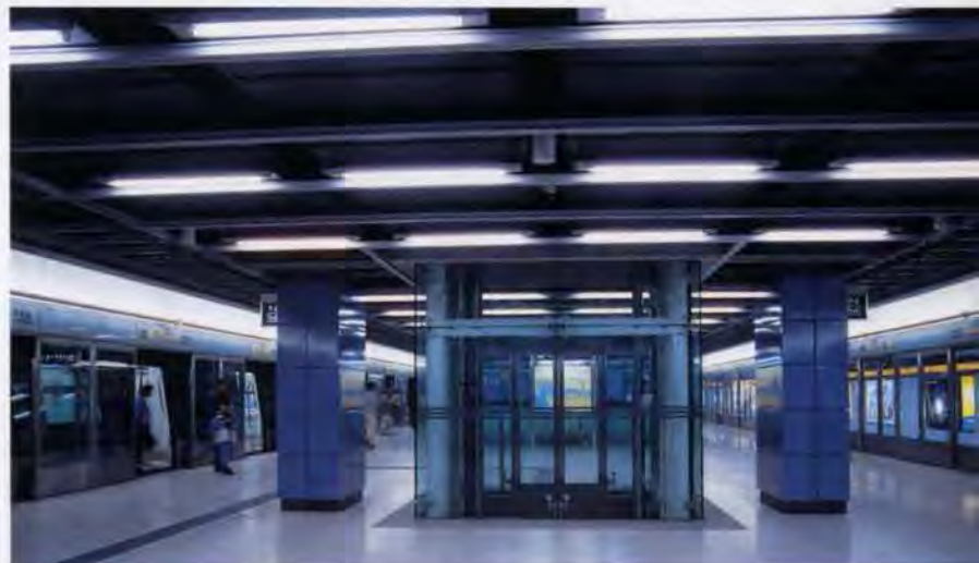
5. Island platform with columns clad in vitreous enamel steel panels. The glass-enclosed lift is customised for each station but developed from system-wide generic principles developed for MTRC by Arup Associates.
