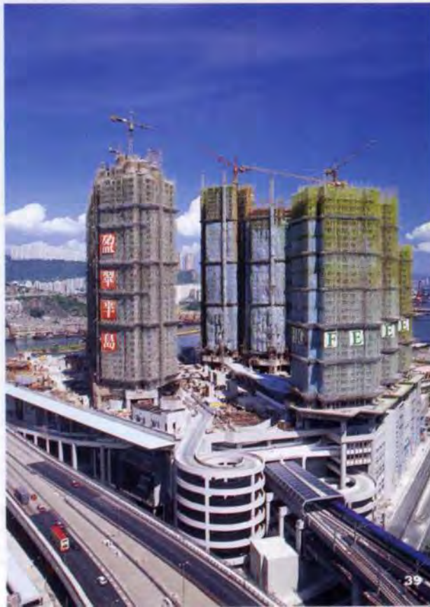
7 right: Residential tower development under construction. Along the northern elevation, adjacent to Tsing Tsuen road, a 300m long, 12m wide cantilever noise canopy framed in structural steelwork is provided to lessen the effect of traffic noise on the residential towers above.
