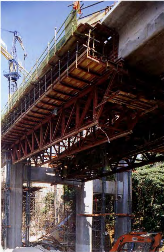
13. Prestressed concrete box viaduct superstructure under construction.
