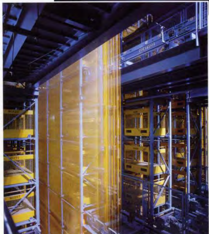
9. Stacker cranes operating within BSS.
