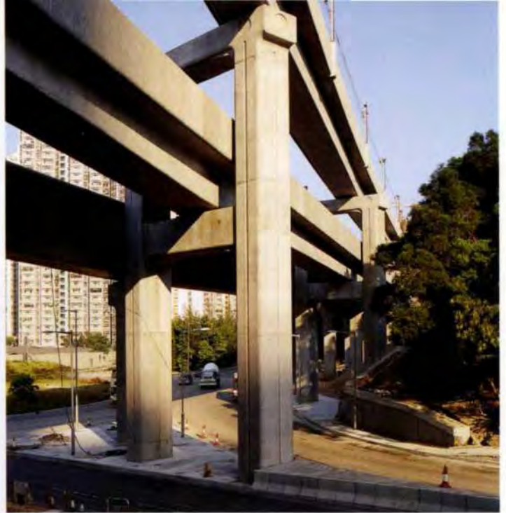
15 above: Viaducts at Tam Kon Shan Interchange.
