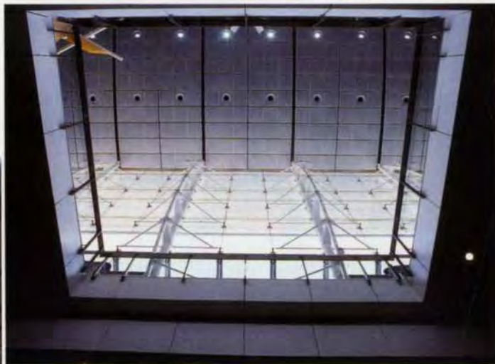
22 below: Light-well viewed from AEL concourse into check-in hall.
