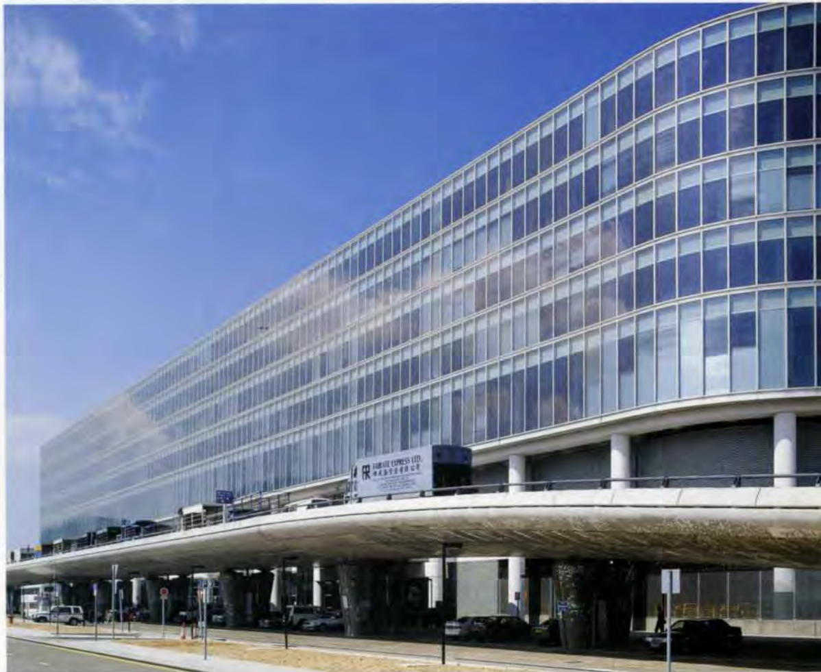
10. South façade of Terminal.
