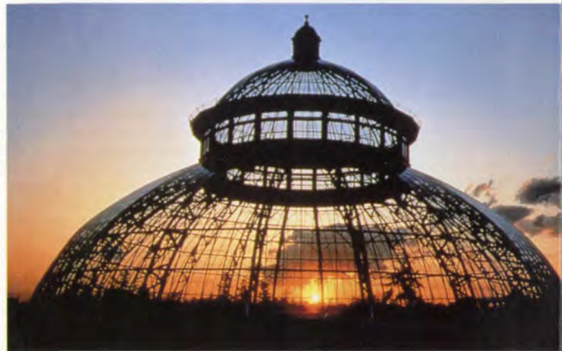
7. House 6, after restoration.
