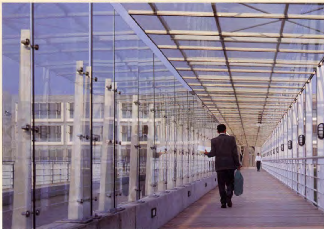
4. Interior of glazed bridge to main entrance.
