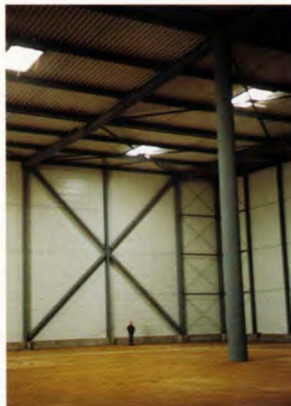
9. The clear internal height is 14.6m.
