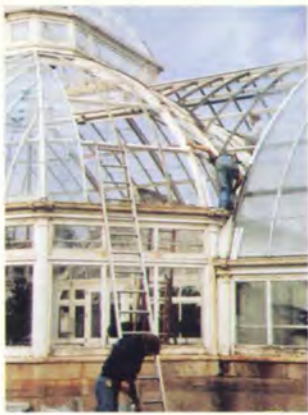
3. Mock-up work under way prior to issuing of construction documents.
