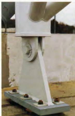
4. Spaceframe column connection to foundation.
