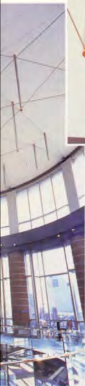
10 above. Detail of tensegrity structure of Rotunda.
