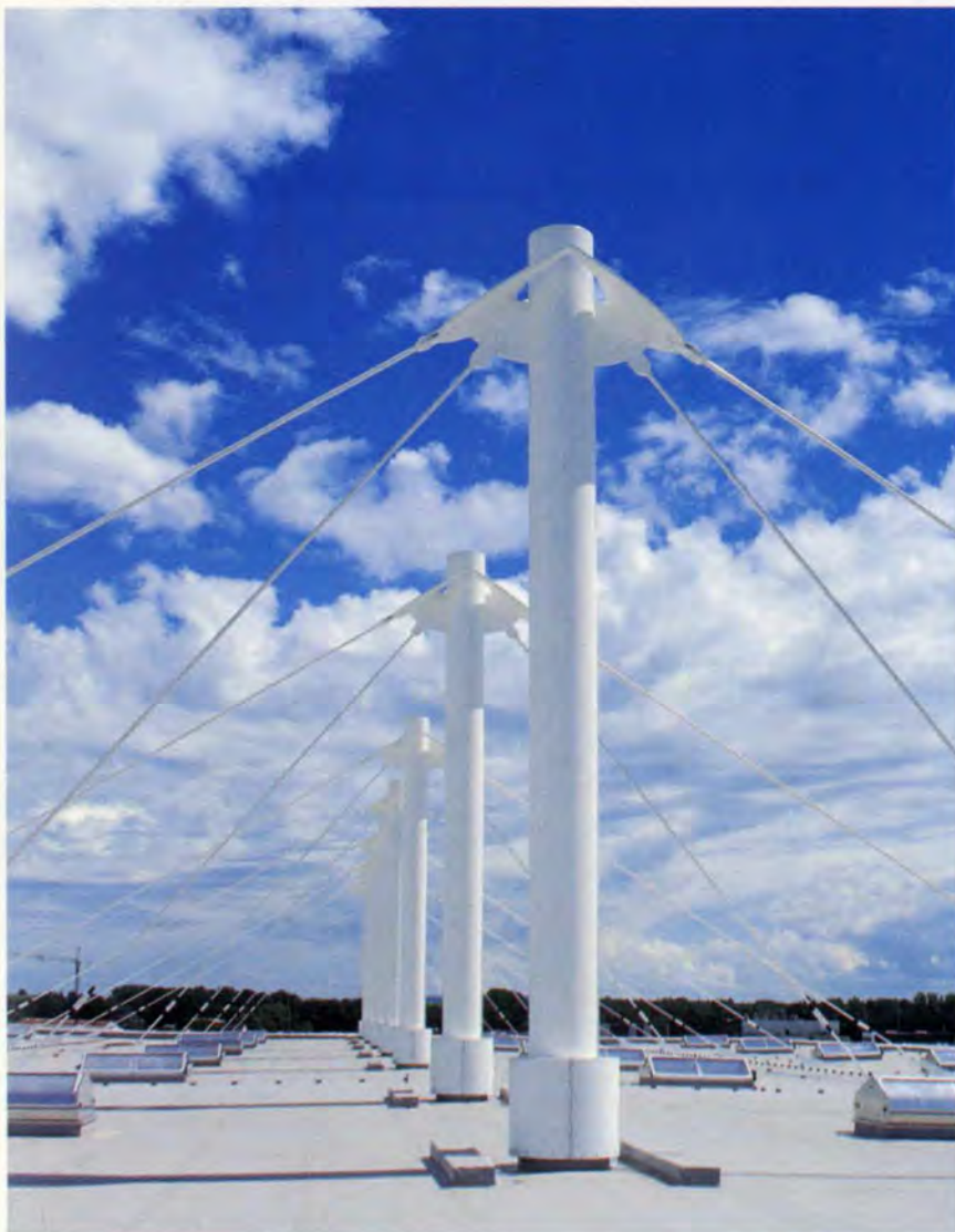
8. The 12.5m main column extensions at roof level.
