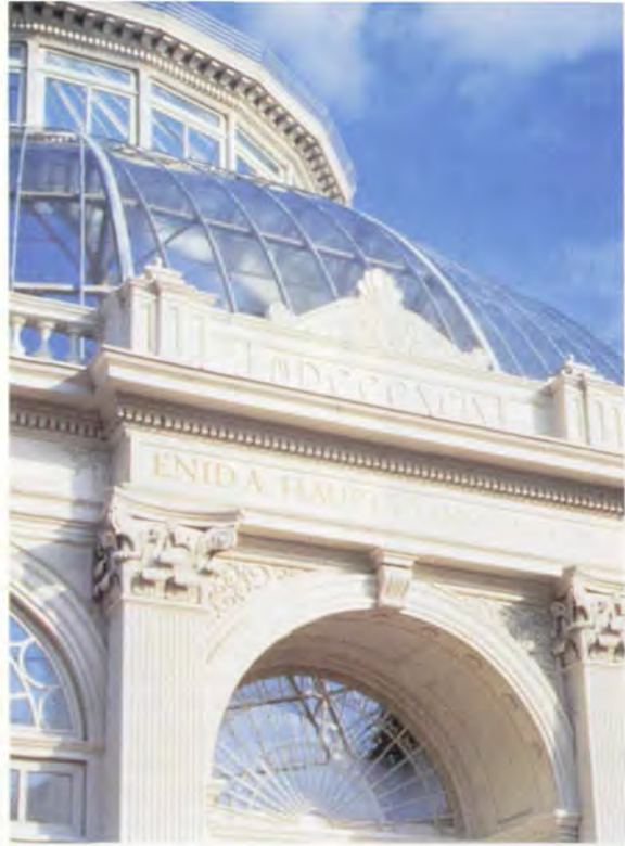
6. Cast aluminum entry to House 6 after restoration.
