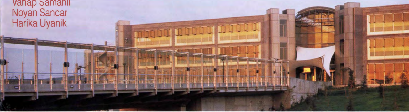
1. Bridge leading to main entrance. View from south-west.
