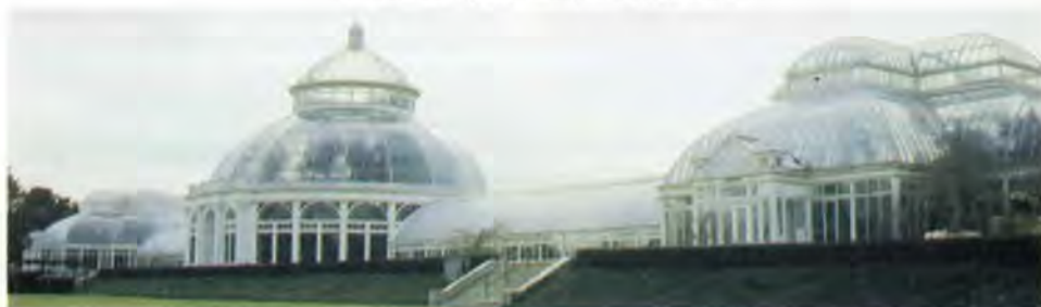
2. View looking southeast prior to restoration.
