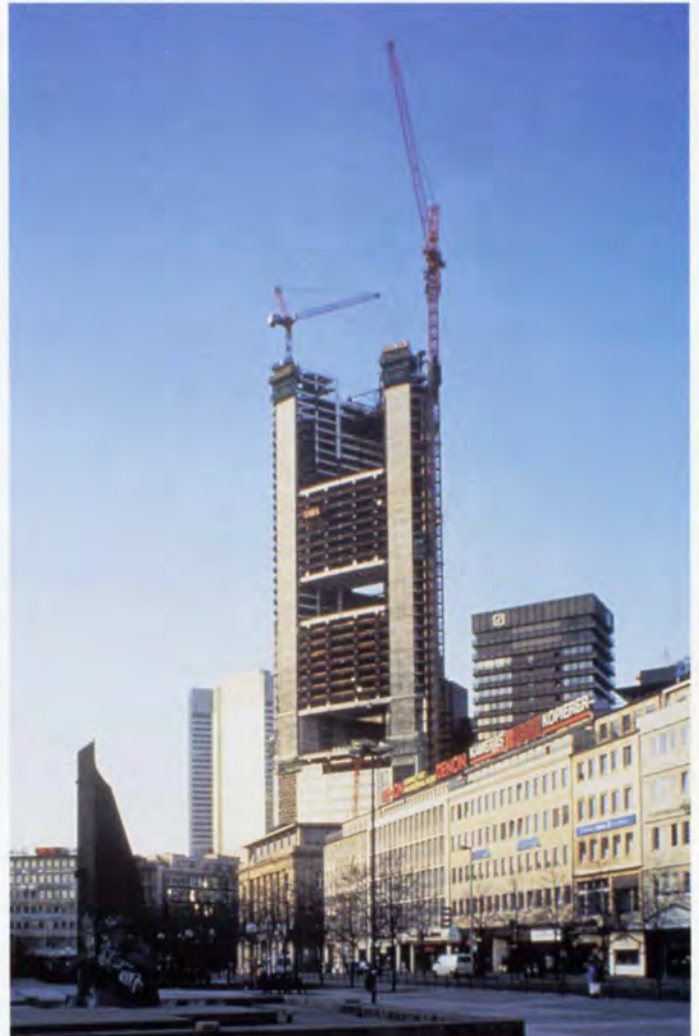
27. Construction at April 1996.
