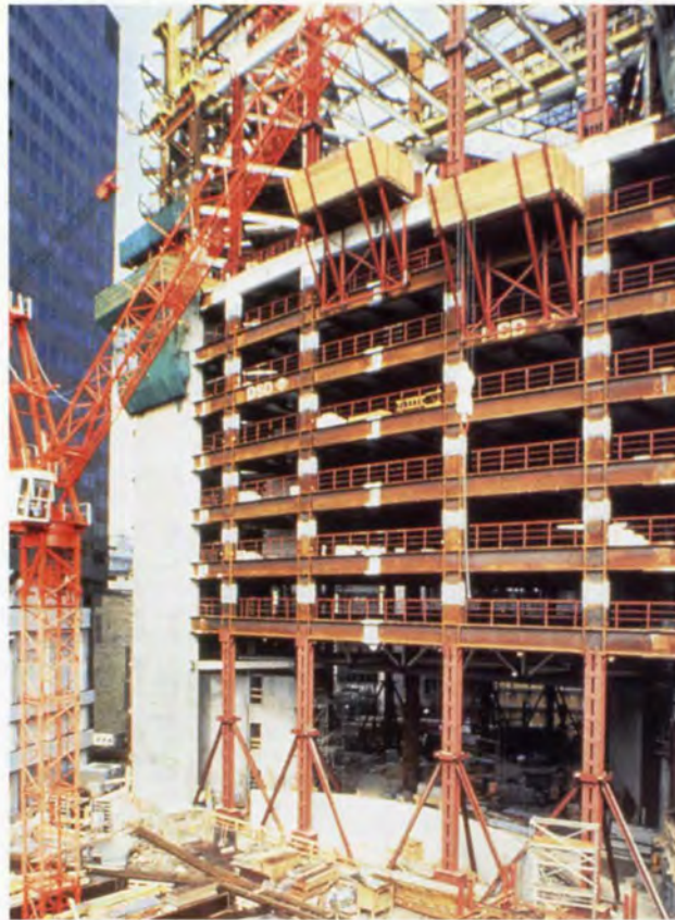
26. Construction of first vierendeel showing temporary props.
