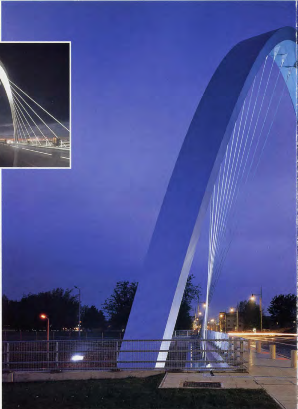
2. The completed bridge.
