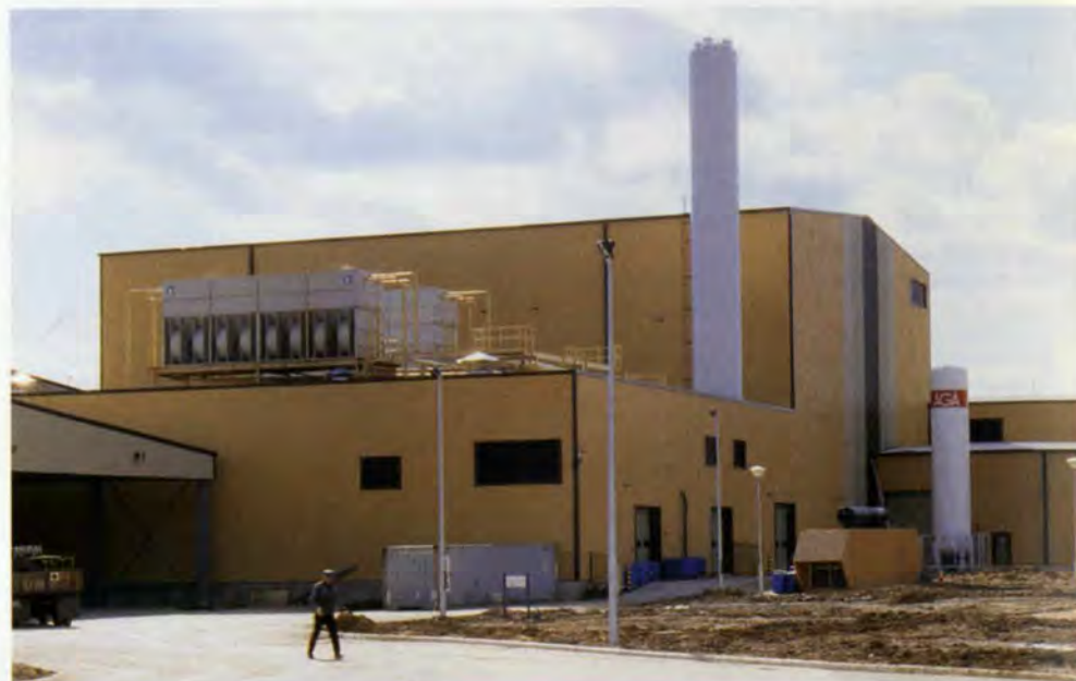
6. Energy centre (foreground), with the chocolate manufacturing building behind.
