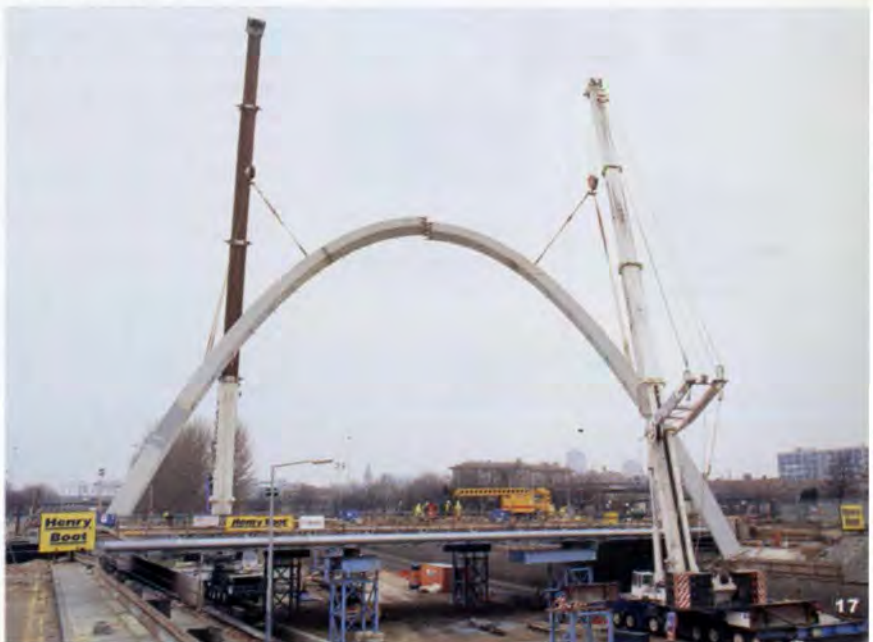
10. Arch erection.
