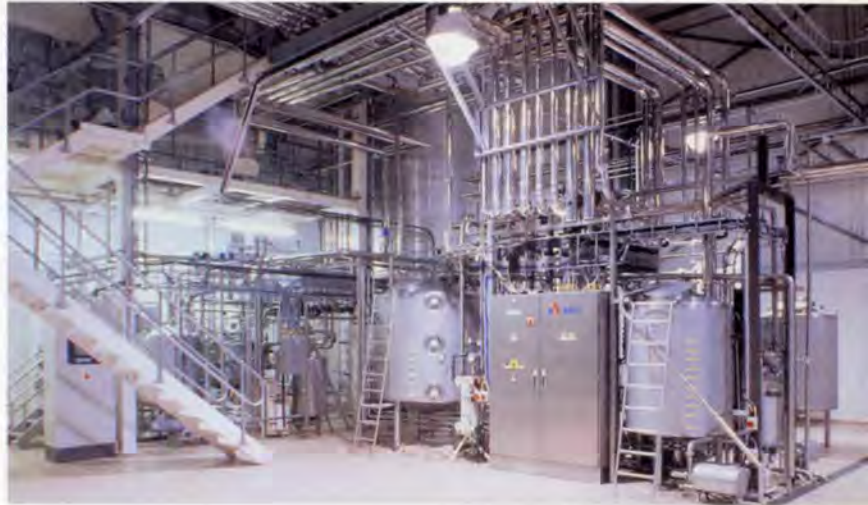
8. Caramel making plant.
