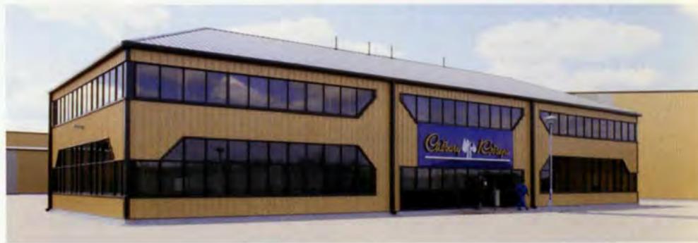
5. Front of administration block.
