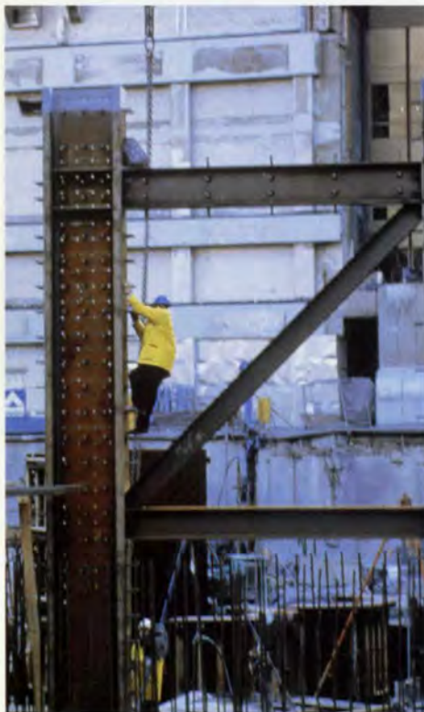
25. First lift of floor column steelwork.
