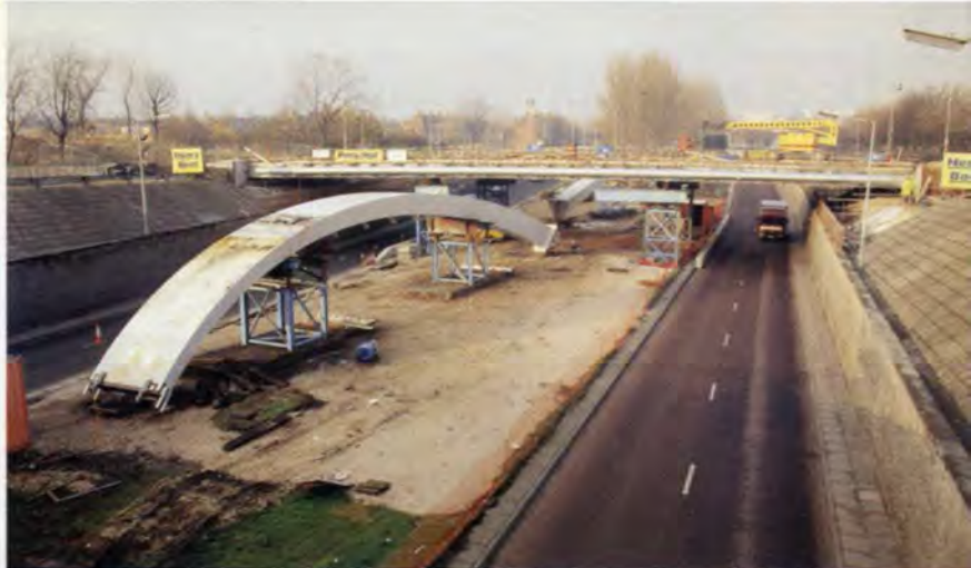
9. Arch half in Princess Road central reservation.
