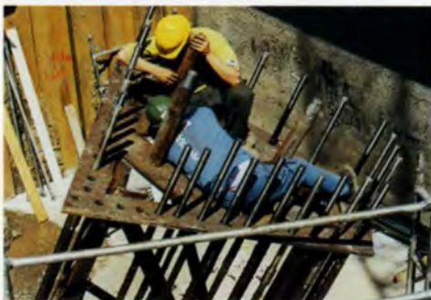
6. Macalloy bars in 'rocket launcher' support framework.
