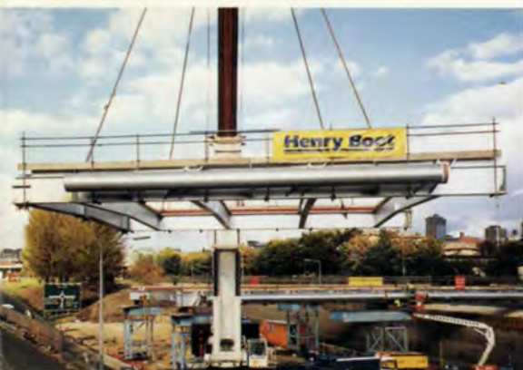
5. The deck being placed.
