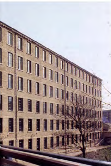
from new bridge.
