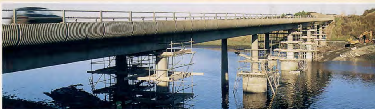
4. North Seaton Bridge, with temporary coffer dams for remedial works
