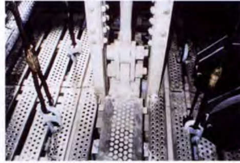
4. The 1st grid before renovation.
