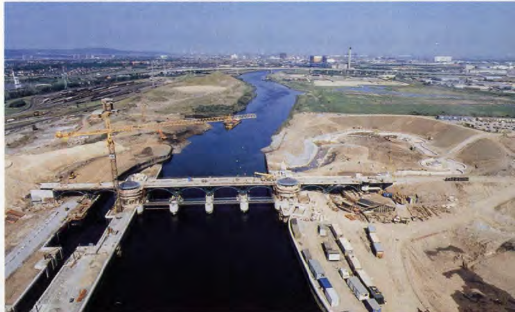
15. The bridge under construction: early 1994.
