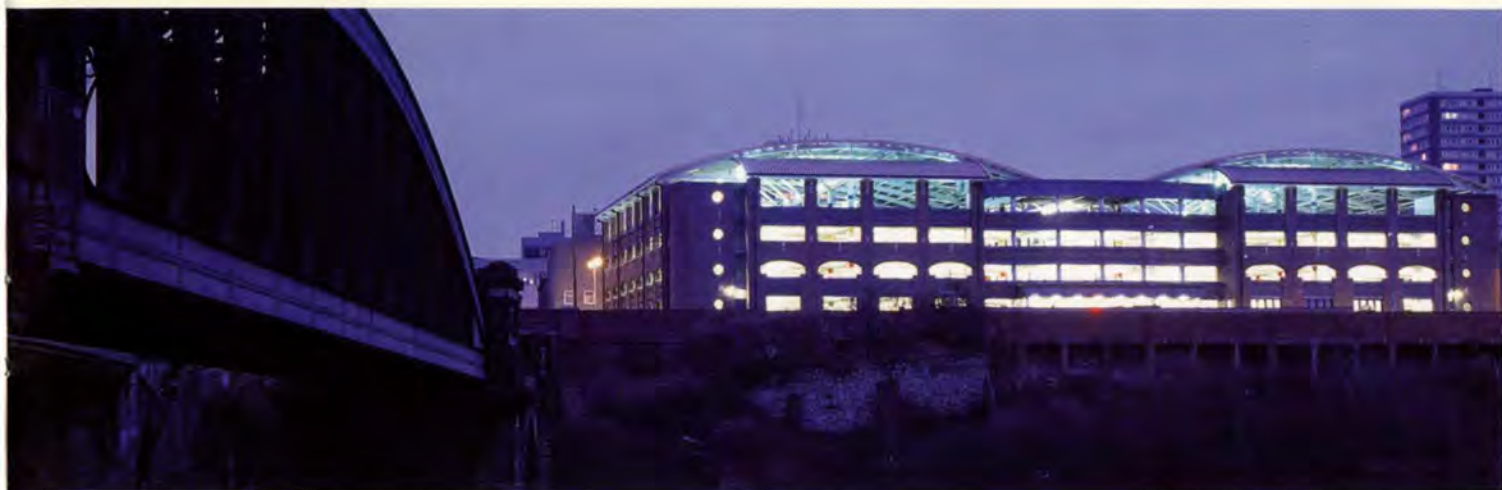
6. Night view of the brightly lit car park. Wearmouth Bridge is seen left of picture.
