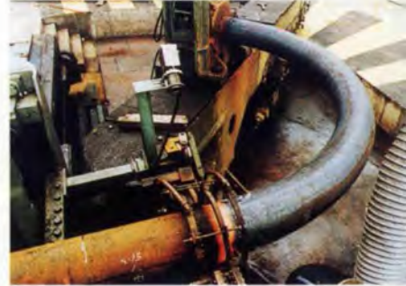
12. Induction bending in progress.
