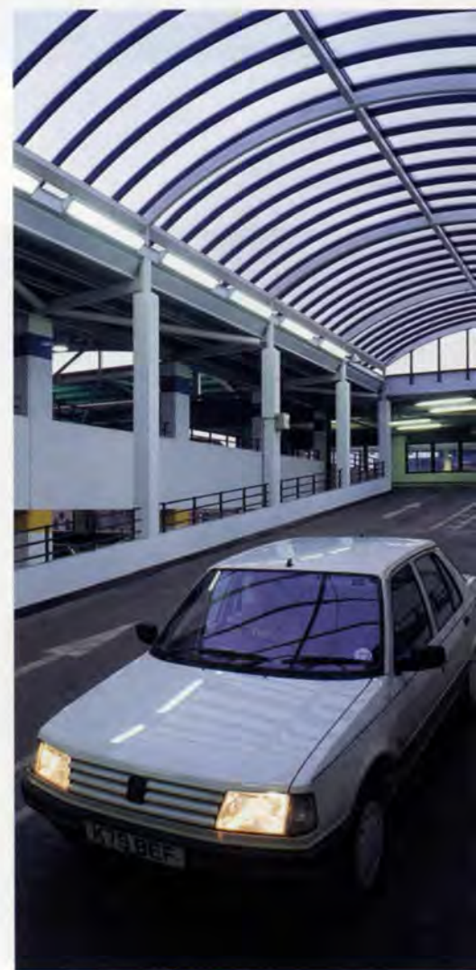
1. St. Mary's Car Park : a new concept in design both for vehicles and pedestrians. Secure, brightly lit and user friendly.
