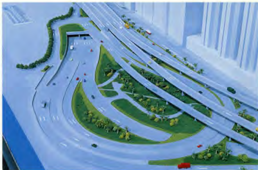
9. Part of model of grade-separated interchange between tunnel approaches and Route 7 (note tunnel portal in upper left of picture).
