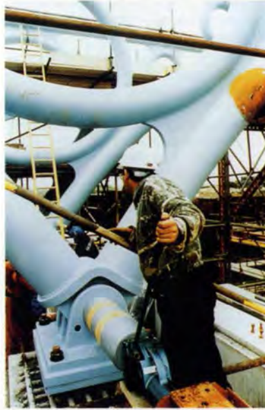
14. Inserting arch pin.
