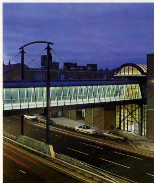
5. Glazed pedestrian bridge over ring road at second floor level provides direct access to city centre shopping area.
