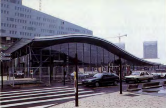
9. End glazing exterior where the Le Corbusier Viaduct divides the station: The gap between the tops of the façades and roof structure is clearly visible.
