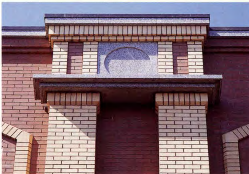
1. Brickwork detail on the refurbishment.
