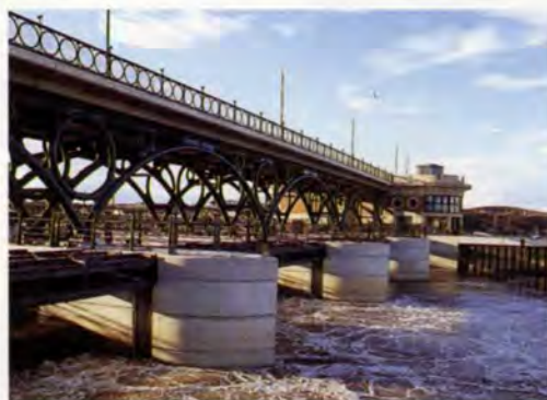
8. Concrete barrage piers.
