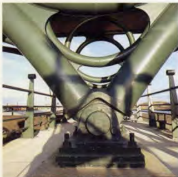
9. Detail of pinned arch supports.
