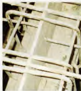
6. Close-up of original inverted T-beam.
