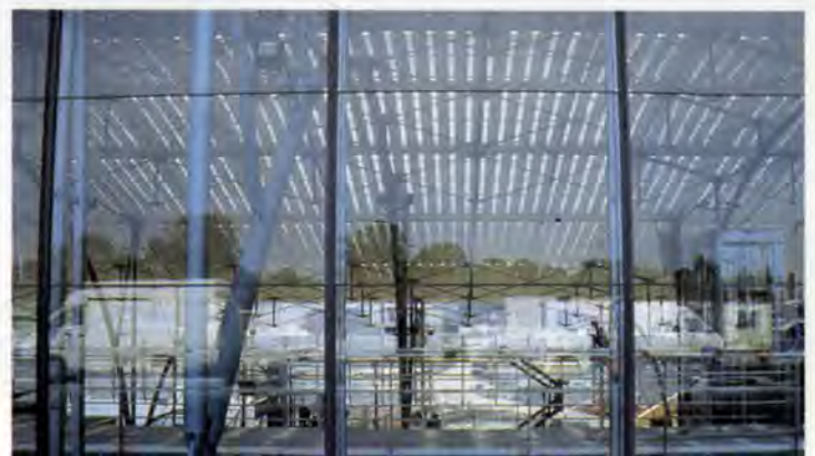
8. Elevation of east façade, with inside of roof clearly visible.
