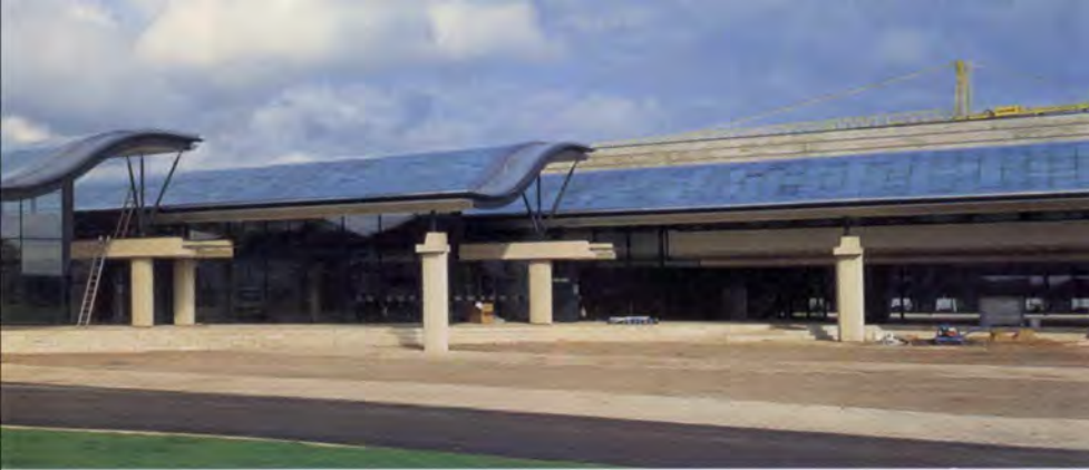
3. The lecture rooms: with the curving, 'floating' roofscape.
