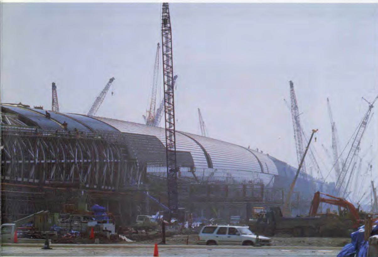
10. Wing under construction, August 1993.
