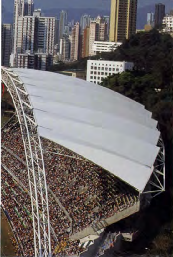
9. The fabric roof.
