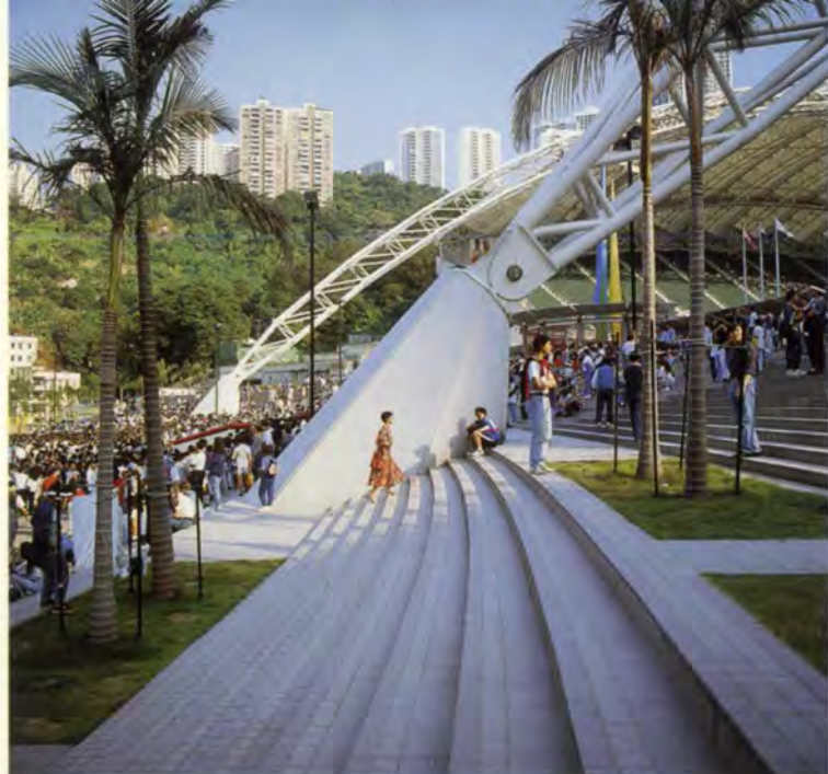
15. View of roof truss bearing and abutment.
