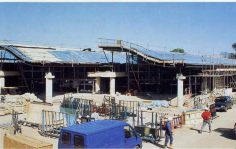
12. Construction work in progress.
