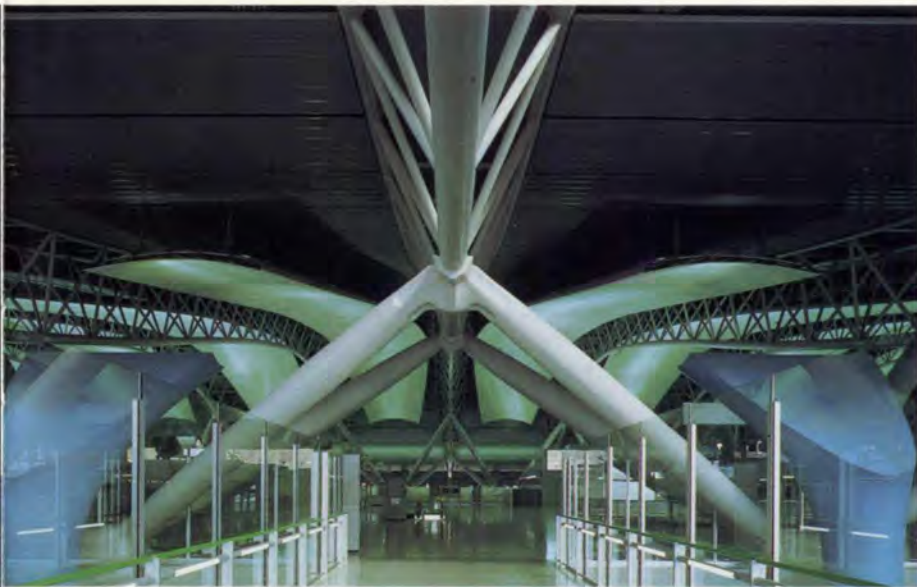
9. Macro jets supplying air to MTB using open air-ducts.
