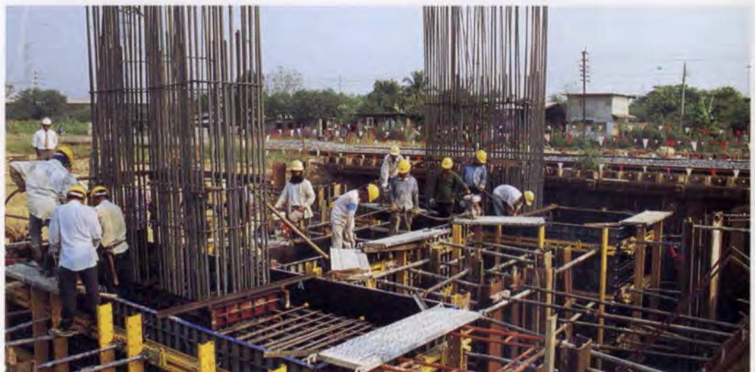
8. Pilecap construction.
