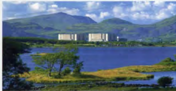
b. The reactor buildings lowered to c.30m.
