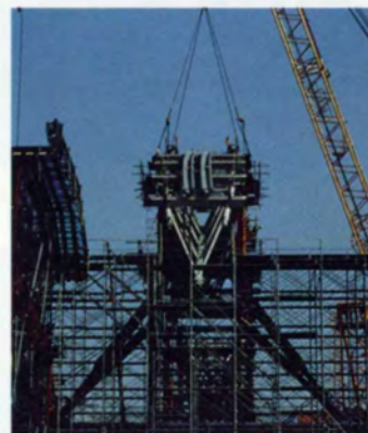
7. MTB roof trusses, and (below) 8. during erection in April 1993
