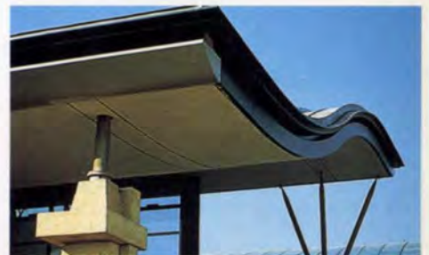
10. Detail of roof corner support.
