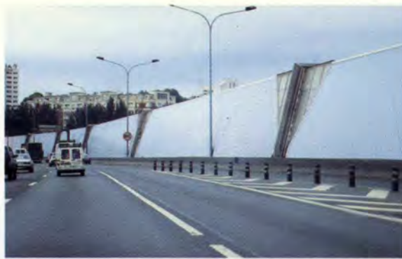
13. High steel barrier in Paris, and right: 14. Transparent barrier in Holland: this reduces noise but also allows views out for the motorist.
