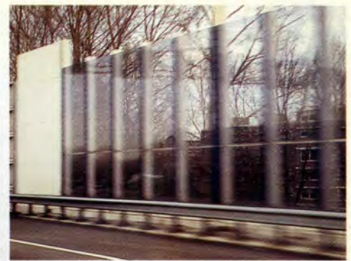
13. High steel barrier in Paris, and right: 14. Transparent barrier in Holland: this reduces noise but also allows views out for the motorist.
