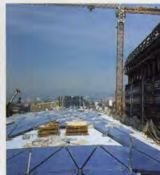
◀ 14. Layers of Deliberatif roof; top: insulation and vapour barriers in steel frame; middle: plywood panels; bottom: weather seal membrane (white).
