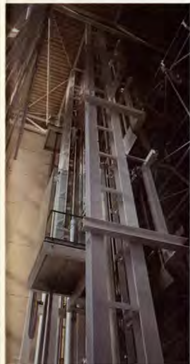
8. Lift at UK Pavilion, Expo '92, Seville, 1992.
