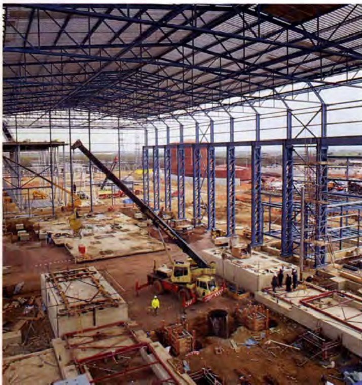
5. Peterborough turbine hall under construction, showing gas turbine and steam turbine blocks.
