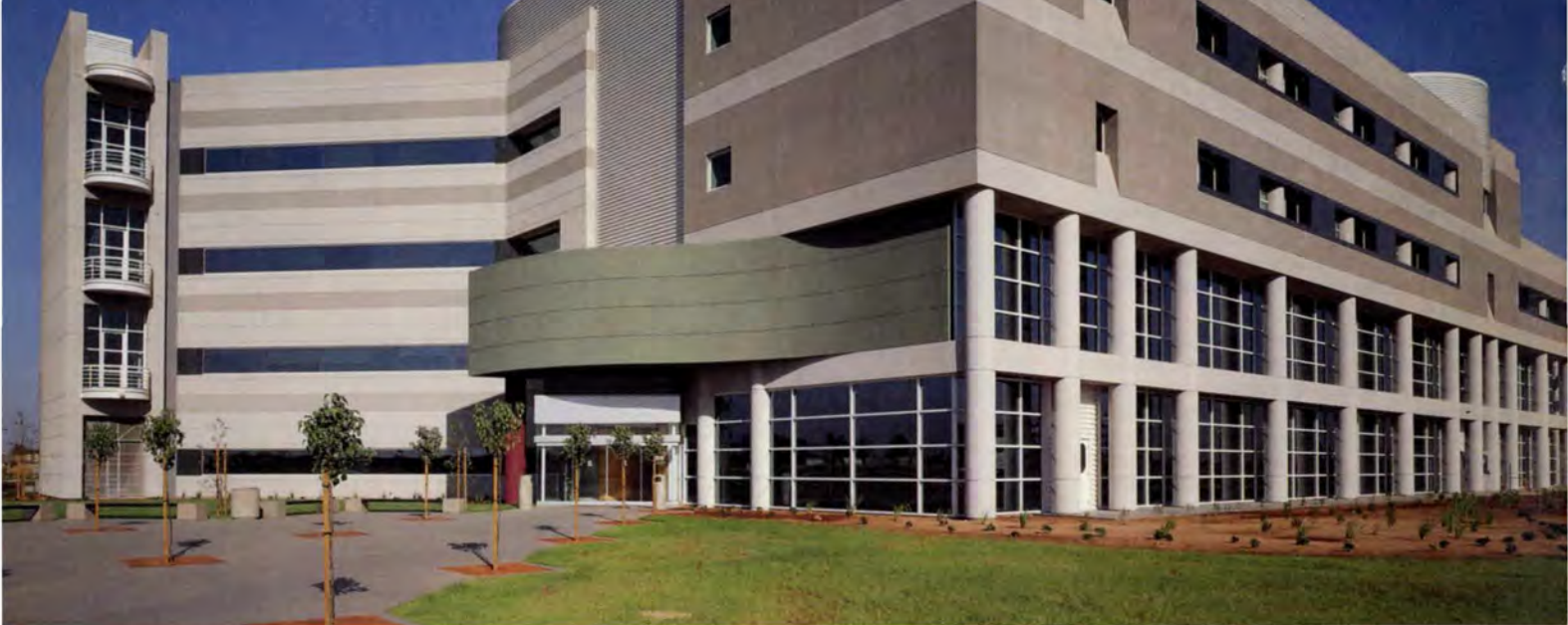
1. Phase 1 MOB and mall. The latter has expressed columns and beams at the two lower levels.
