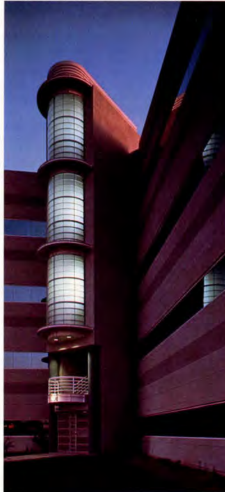
3. Phase 1 MOB from interior courtyard, looking north.
