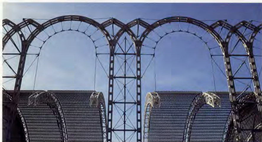
7. The stone arches of the Pavilion of the Future for Expo '92 in Seville, Spain. Similar to a web, the lightness of the structure is achieved by designing for deflections rather than preventing them.
