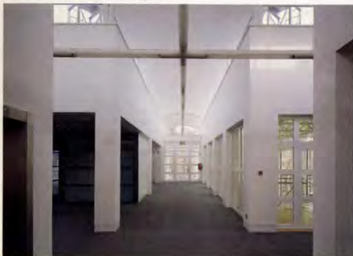
9. Interior showing natural top lighting.
