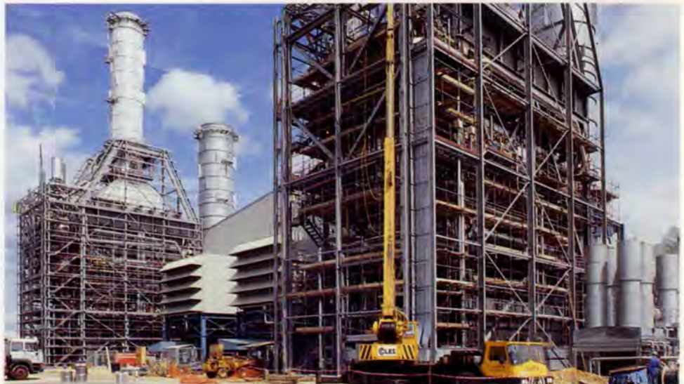
14. Peterborough heat recovery boilers under construction.
