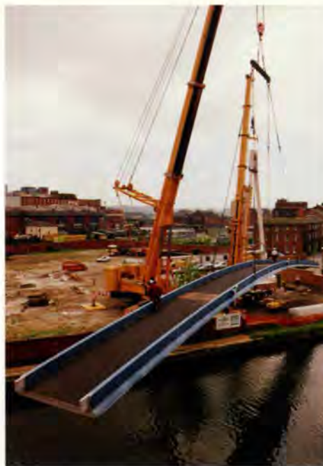
2. Lifting the deck, 10 June 1992.
