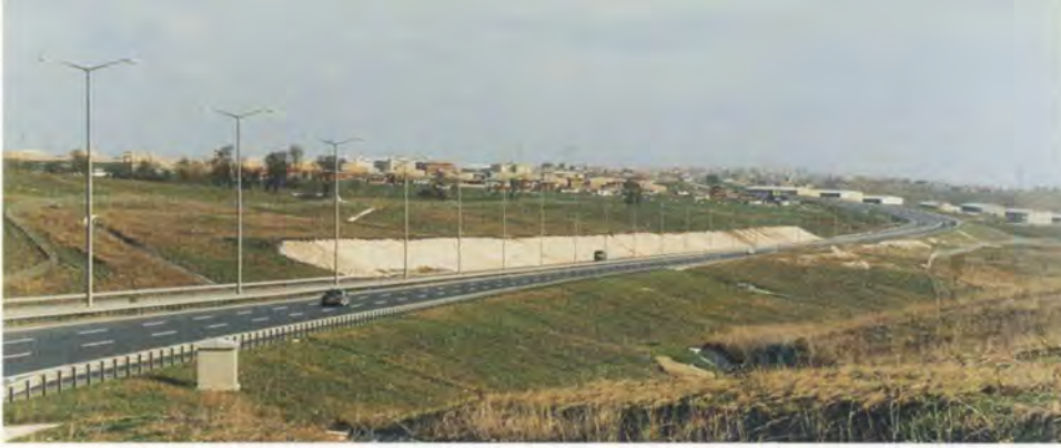
8. 15m deep cutting in sidelong ground, Lot 1.
