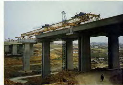
3. Apparatus for launching deck beams on structures.
