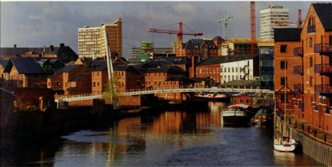
5. The bridge viewed from the east.
