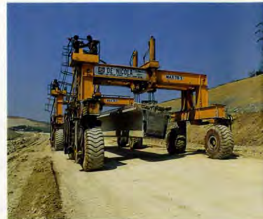
2. Deck beam being transported between casting yard and viaduct location.
