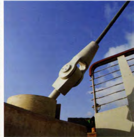
6. Backstay anchorage and the 'nautical' handrail on the southern bank.
