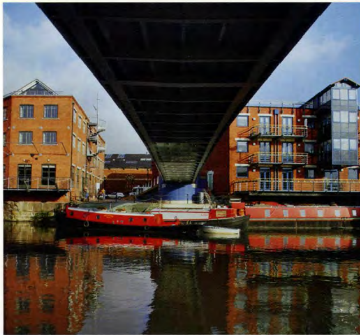
4. Underside of the deck, showing transverse and longitudinal stiffening.
