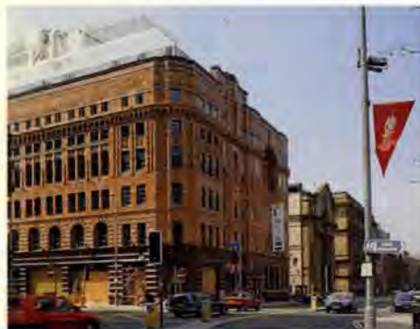
7. The new three-storey building above the refurbished terracotta.
