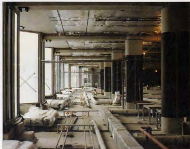
10. Services placed in circumferential route prior to floor laying.
