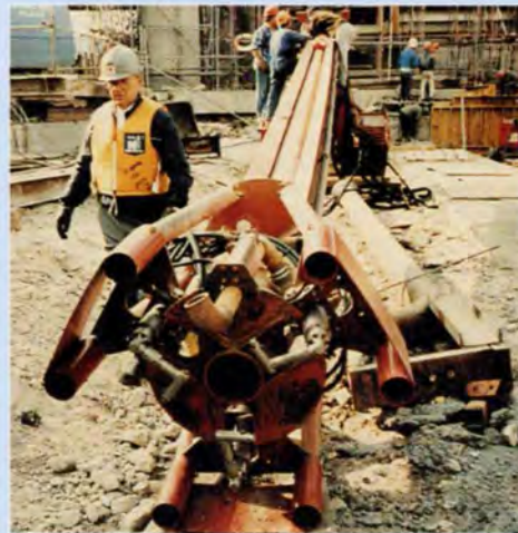
B. (below): Specially-developed hydraulic auger.
