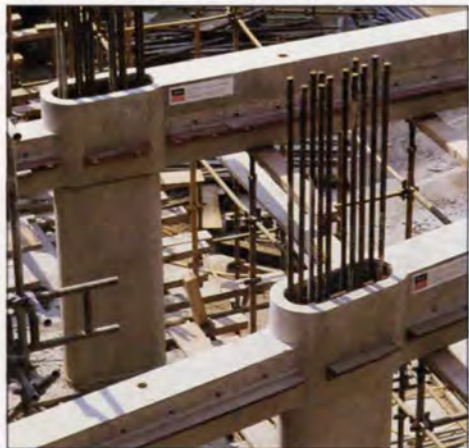
7. Reduced depth beam/column connection showing stepped beam on left, and steel angle floor supports in foreground.
