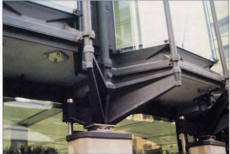
Left 14. Façade support bracket, with stainless steel tension rod on left and below 15. Gunmetal support bracket.
