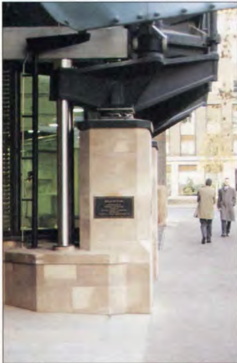
Left 14. Façade support bracket, with stainless steel tension rod on left and below 15. Gunmetal support bracket.
