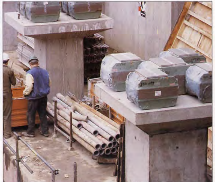
12. Acoustic isolation of new offices.
