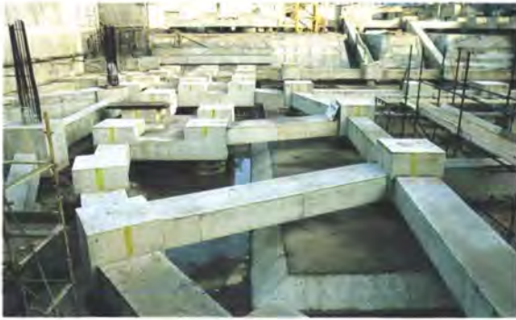
5. Undercroft showing the beams and bearings (Photo: Peter Mackinven).
