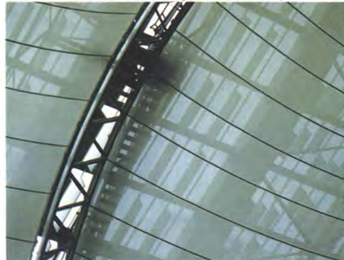
△ 2. Suspended absorbers and ▽ 3. ceiling (Photos: Arup Acoustics).
