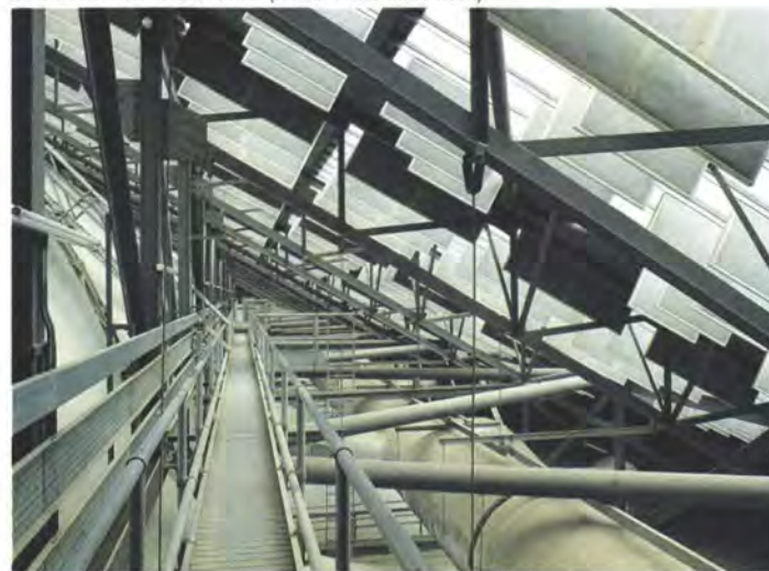
△ 2. Suspended absorbers and ▽ 3. ceiling (Photos: Arup Acoustics).
