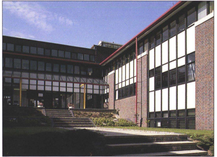
Earth Sciences: Courtyard, below: Roofscape
