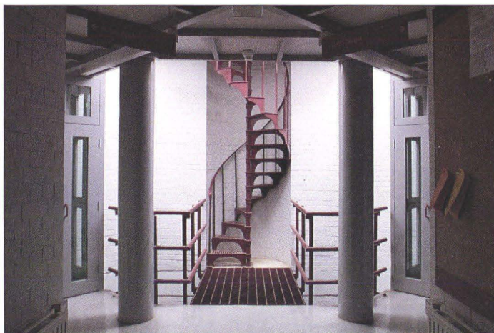
Physics II: Spiral stair to rooftop observatory
