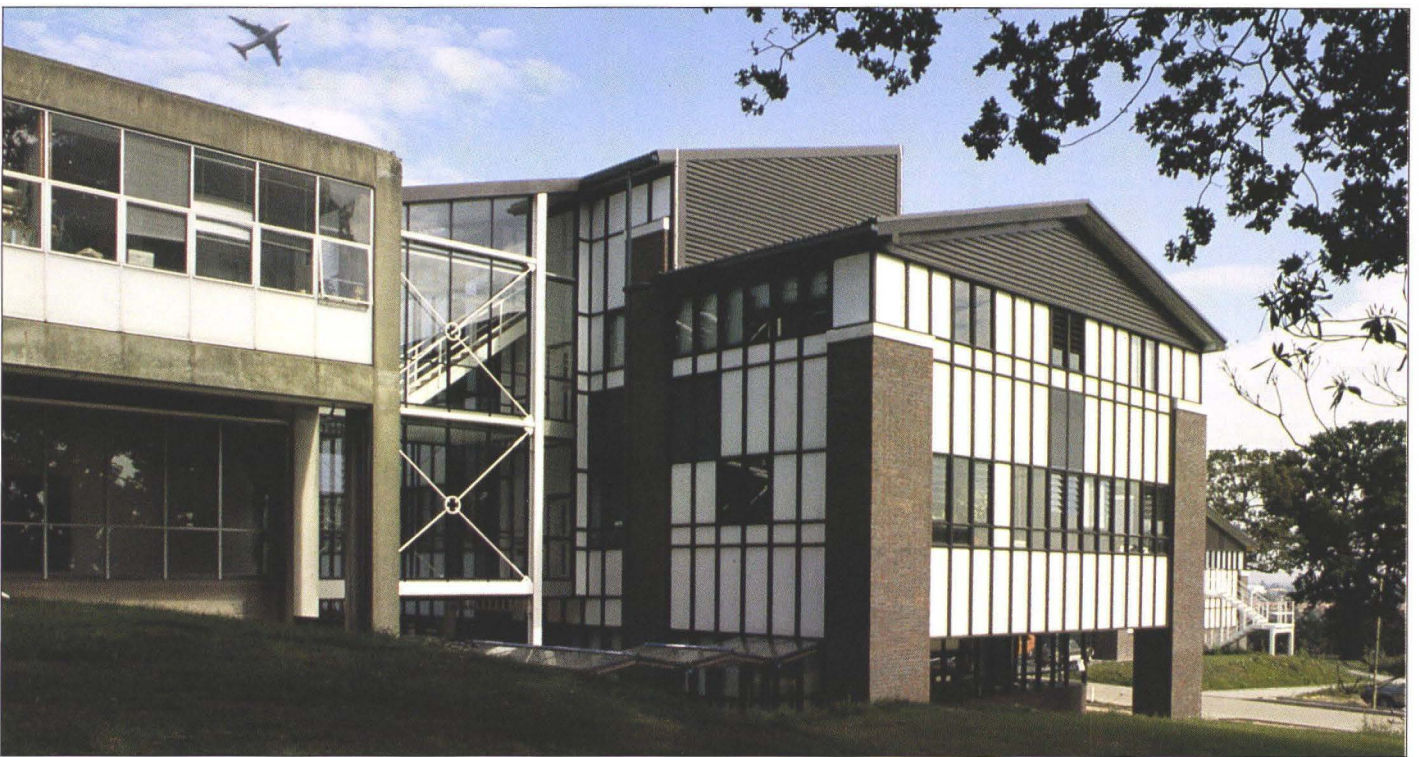
Life Sciences: Link block to Bourne chemistry building
