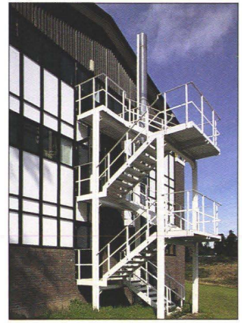
Earth Sciences: Fire escape stair
