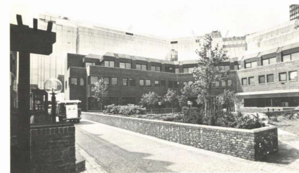
Fig. 12 View from Euston Road during construction
