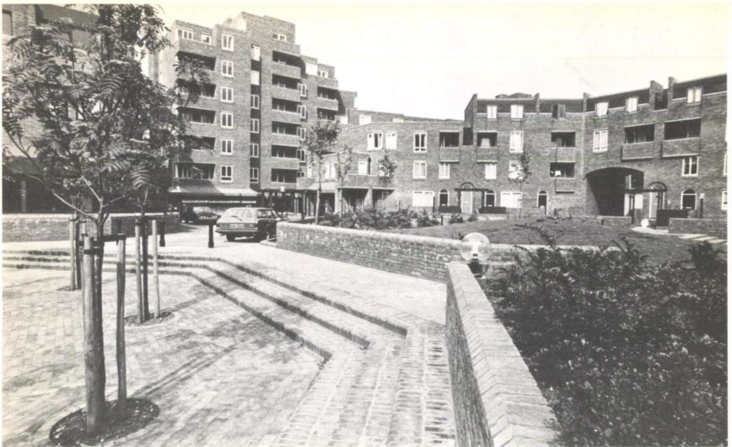
Fig. 17 Local Authority Housing view across square from south-west
