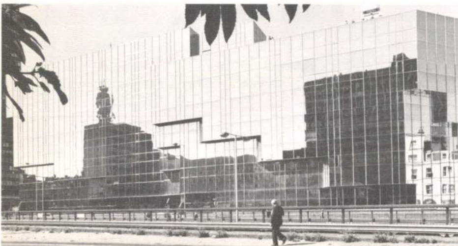
Fig. 18 Detail from square looking from north-east Fig. 19 General view from Euston Road
