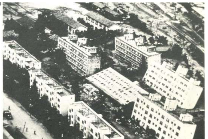
Fig.3 Liquefaction damage (Niigata earthquake, Japan 1964)
