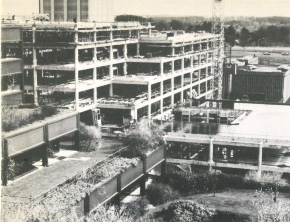
Fig. 7 Erecting the external curtain walling
