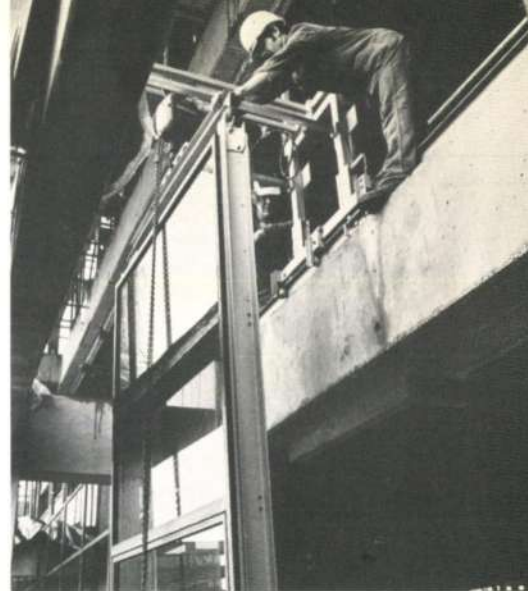
Fig. 7 Erecting the external curtain walling
