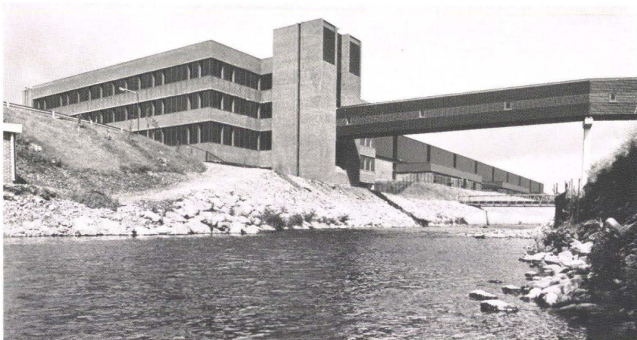
Fig. 4 Bridge Link: Office block to the original Hoover complex (Photo: Harry Sowden)
