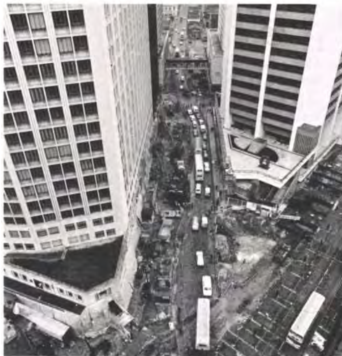
Fig. 21 Construction of the diaphragm wall adjacent to Swire House (Photo: Richard Davies)
