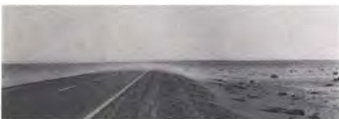
Fig. 10 Saltation across a road surface
