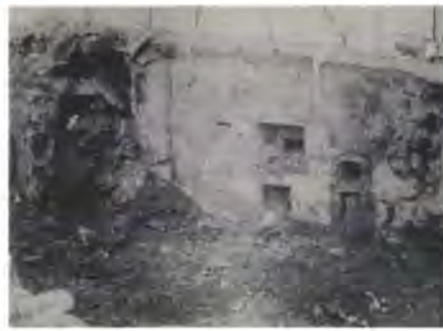
Fig. 4 Basement wall exposed during construction
