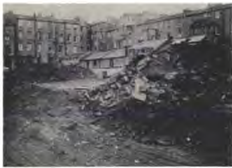
Fig. 3 Stockpile of basement fill material (Photos: Ove Arup Partnership)
