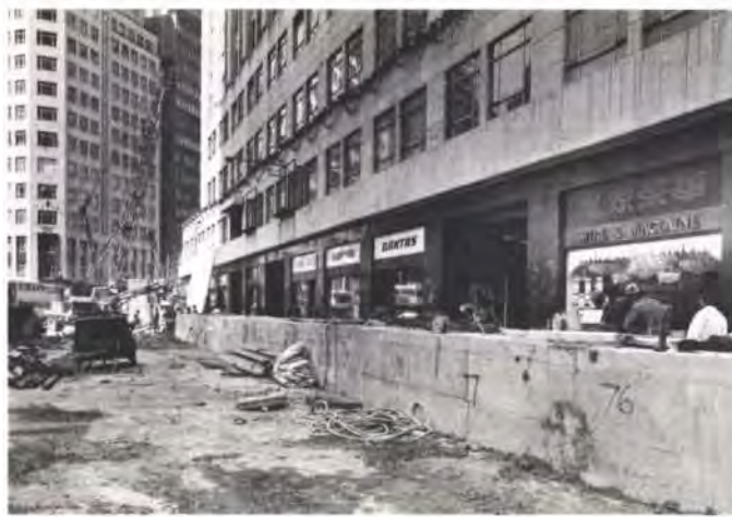
Fig. 23 Initial measurements of settlements of high rise piled building due to dewatering (prior to main excavation)
