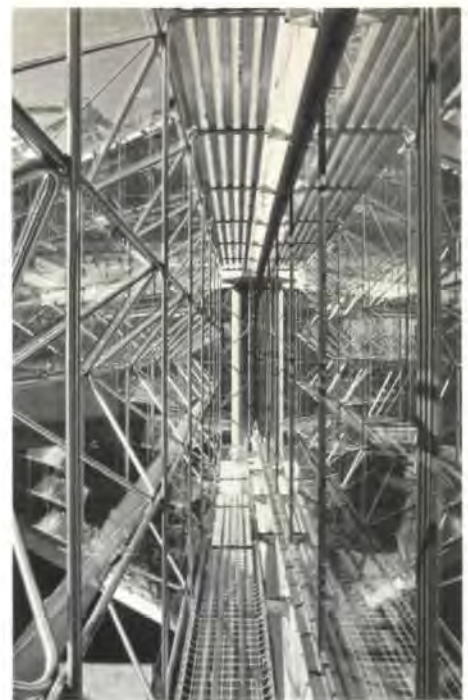
Fig. 5 Space frame sun shading (Photo: David Moore)
