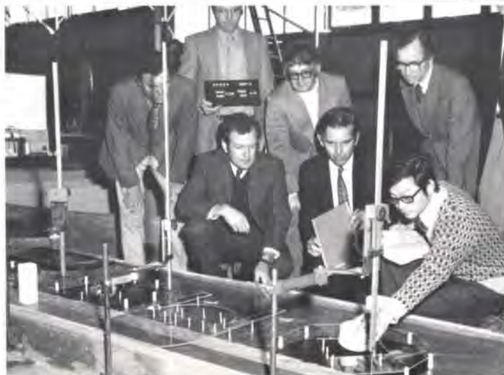
Fig. 4 Model testing of effect of 1000 year flood on proposed channel (Photo: National Capital Development Commission)
