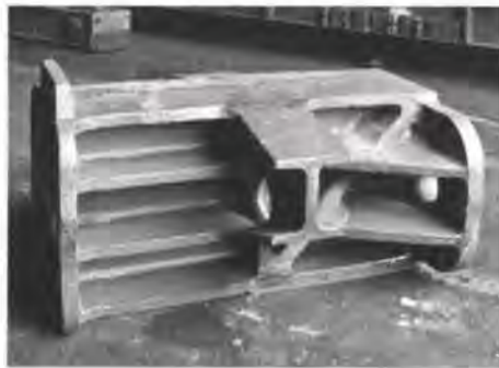
Fig. 7 Casting for corner section of vierendeel girder (Photo: Max Dupain)
