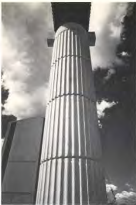
Fig. 8 Conveyor support shaft (Photo: Max Dupain)
