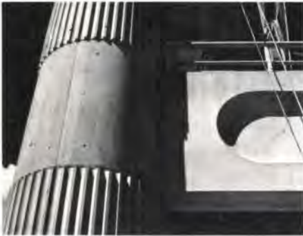
Fig. 4 Detail of preheater tower (Photos: Max Dupain)
