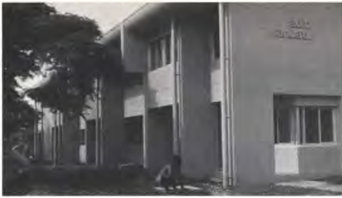
Fig. 4 Studio building showing the emphasis on sun shading to windows and rain water dispersal (Photo : H. Calverley)
