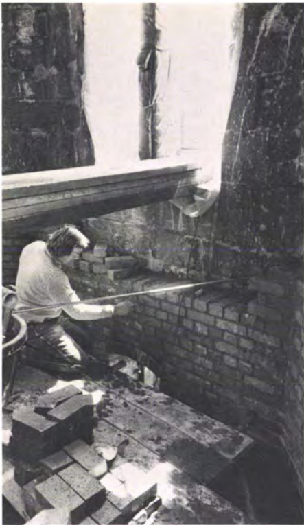
Fig. 14 Laying the brick lining (Photo: Poul Beckmann)
