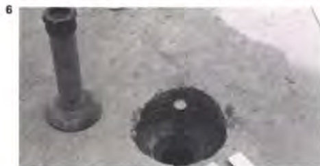
Figs. 3-6 Sequence of rock anchor installations on site for Ministry of PTT Headquarters building (Photos : Robert Pearson)
