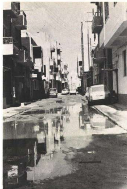
Fig. 4 Side road showing lack of pavement and drainage. (Photo: Malcolm Simpson)
