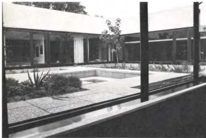
Fig. 9 One of the enclosed, elevated courtyards (Photo: Antoine Raffoul)
