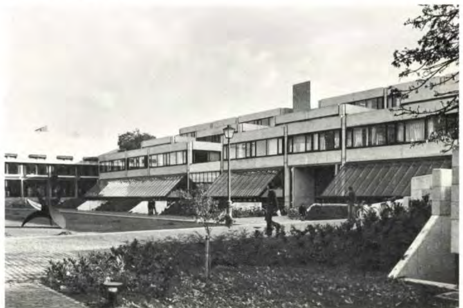
Fig. 5 North face: the clear sloping glazing forms the roof to the double-storey library (Photo: Antoine Raffoul)
