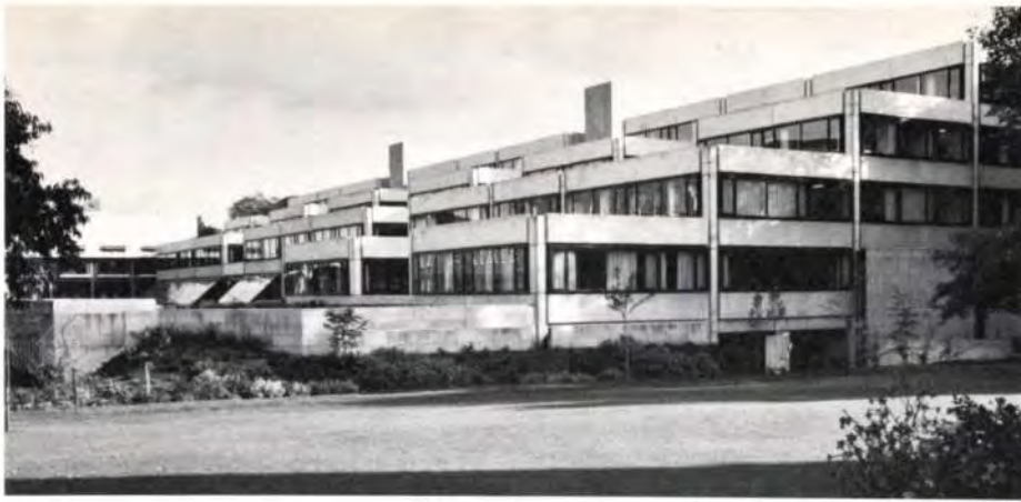
Fig. 7 West face, showing the flank wall of the 400-seat lecture theatre unobtrusively tucked almost below ground and beneath the glazed accommodation in the middle foreground (Photo: Antoine Raffoul)
