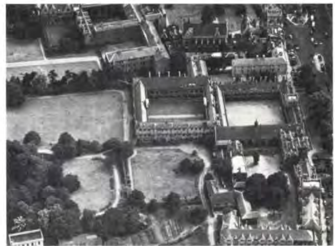
Fig. 5 Aerial view of site
