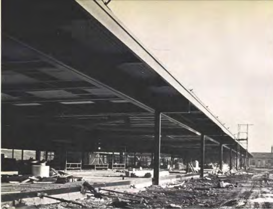
Figs. 4 & 5 Main block under construction (Photo: Emgas)
