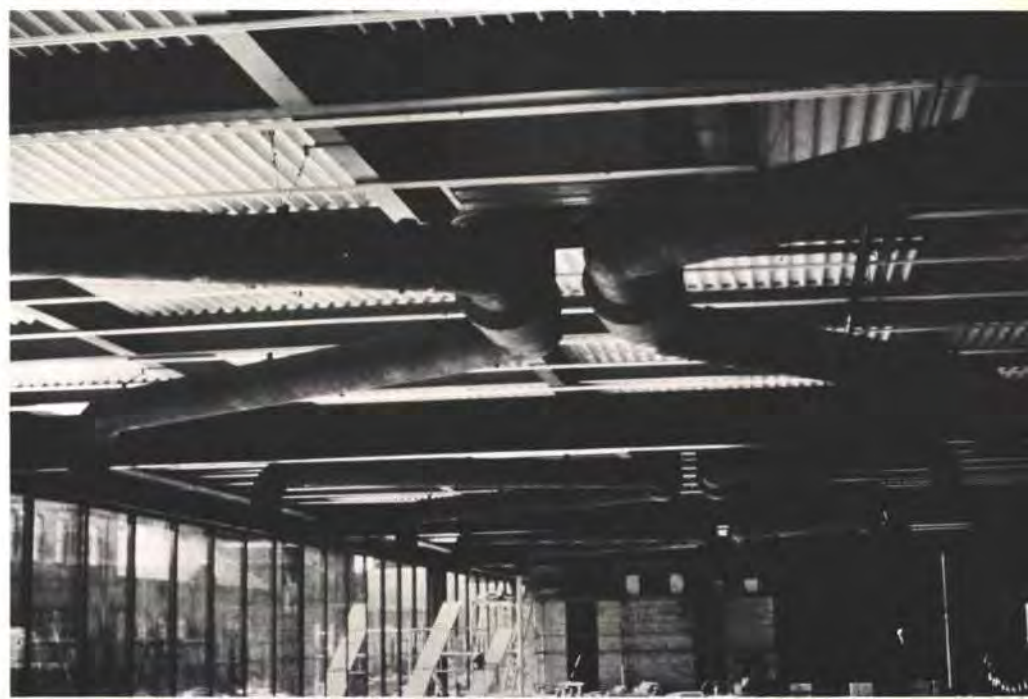
Fig. 6 below Office block under construction, showing main air ducts (Photo: Ken Tune)
