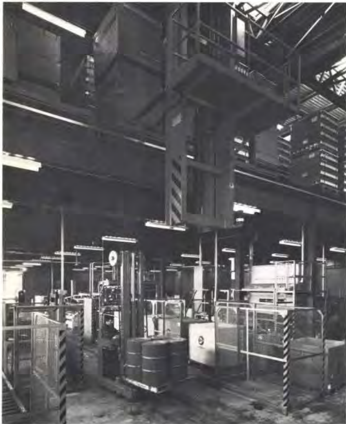
Fig. 4 Overhead storage and filling (Photo: John Whybrowe Ltd.)
