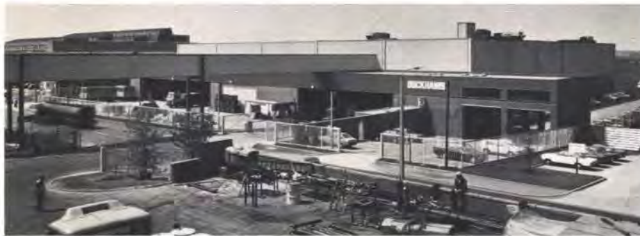
Fig. 16 below New facilities and bridges (Photo: John Whybrowe Ltd.)
