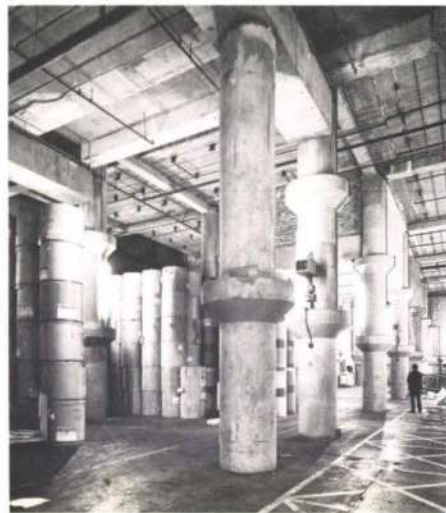
Fig. 17 B3 basement reel store (Photo: Sydney Newbery)
