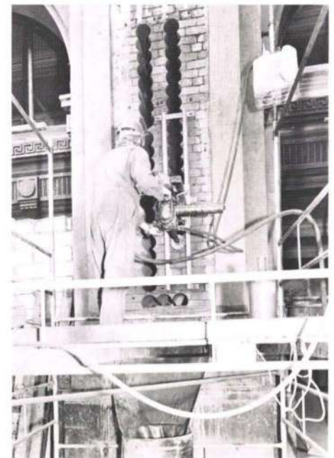
Fig. 5 Drilling the slots into the brick piers (Photo: Elsam, Mann & Cooper)
