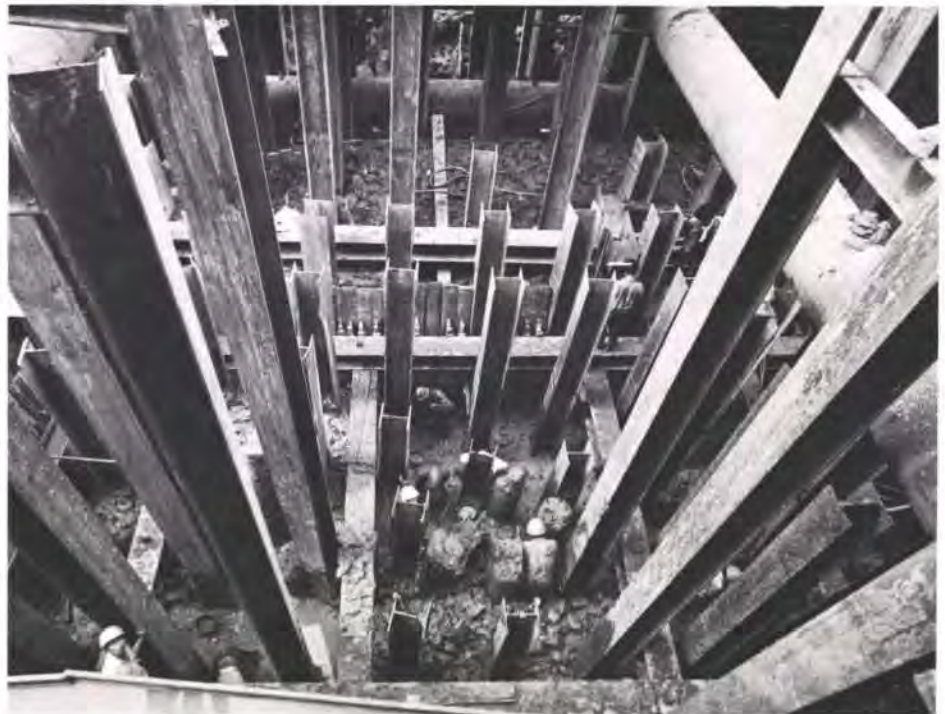
Fig. 5 Foundation piling (Photo: Kouo Shang-Wei)
