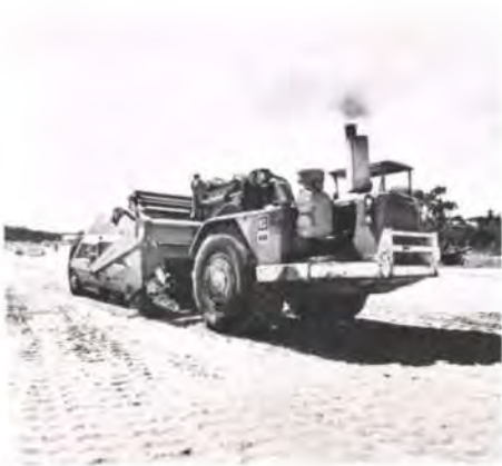
Fig. 7 Caterpillar 621 elevating scraper at work on road construction (Photo: David Gordon)
