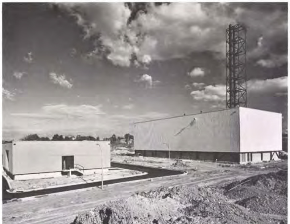
Fig. 6 General view of service area, with the zone substation on the left and the boiler house on the right. (Photo: Lincoln Harvey)
