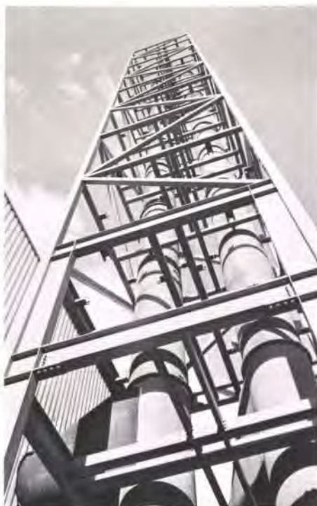
Fig. 8 Boiler house flue structure (Photo: Lincoln Harvey)
