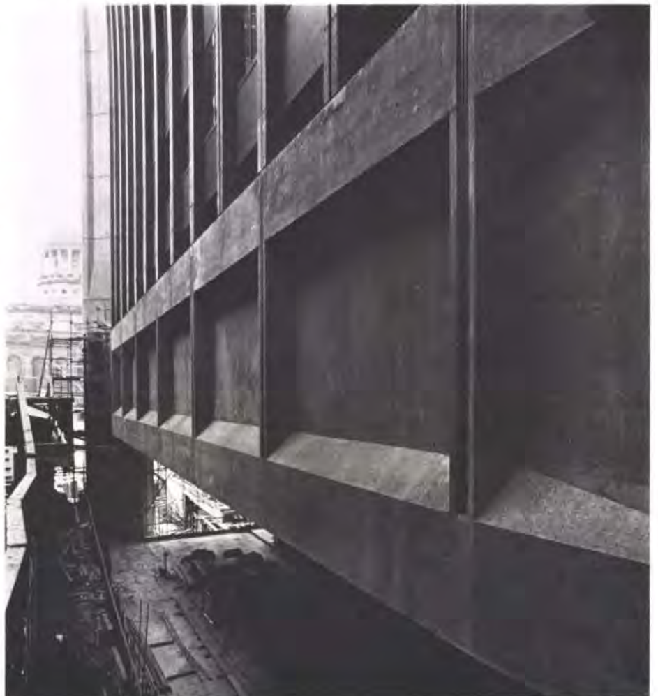
Fig. 8 Level 1 prestressed beam, west façade (Photo: Ian Mckenzie)
