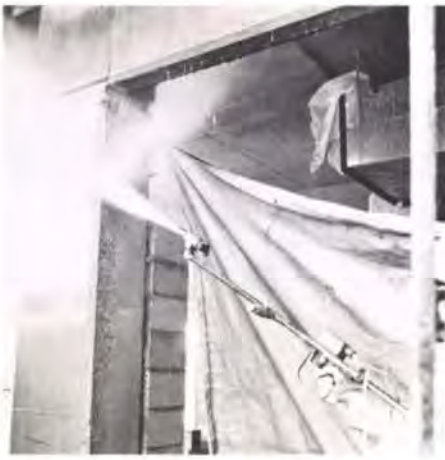
Fig. 4 Water blasting in situ concrete to expose aggregate. (Photo: Lincoln Harvey)
