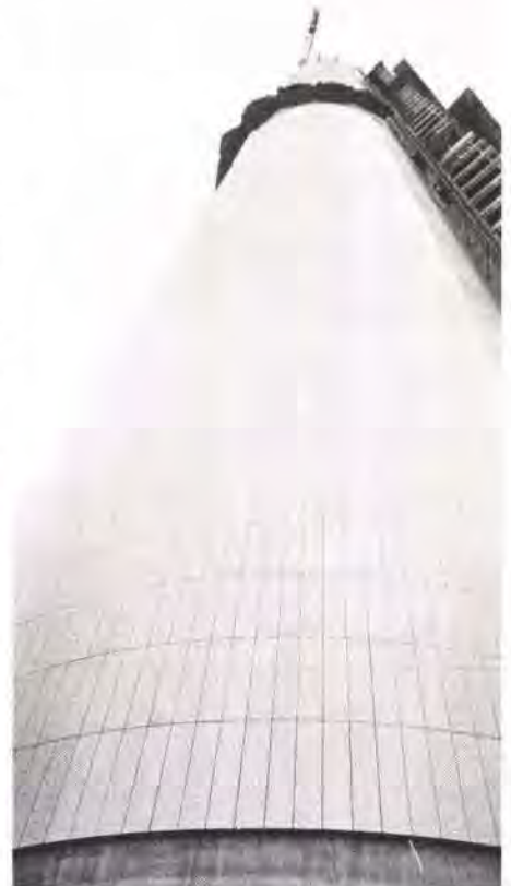
Fig. 15 Granite cladding to the core (Photo: Kouo Shang-Wei)
