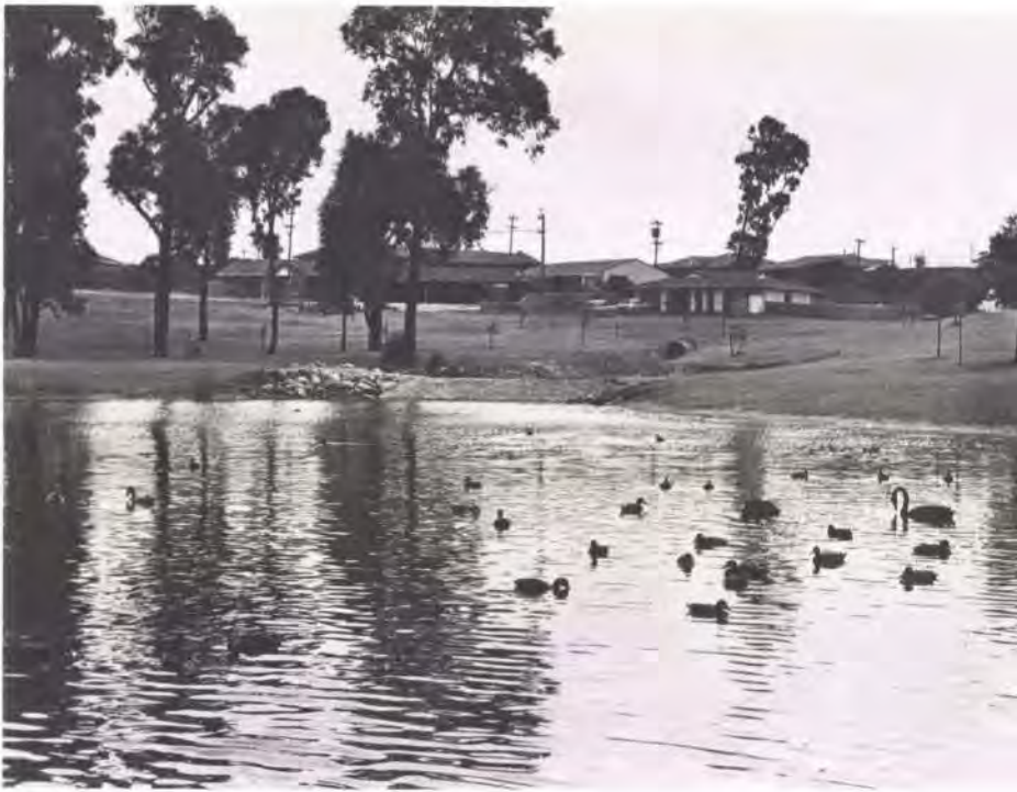
Fig. 5 Pond for stormwater disposal (Photo: David Gordon)
