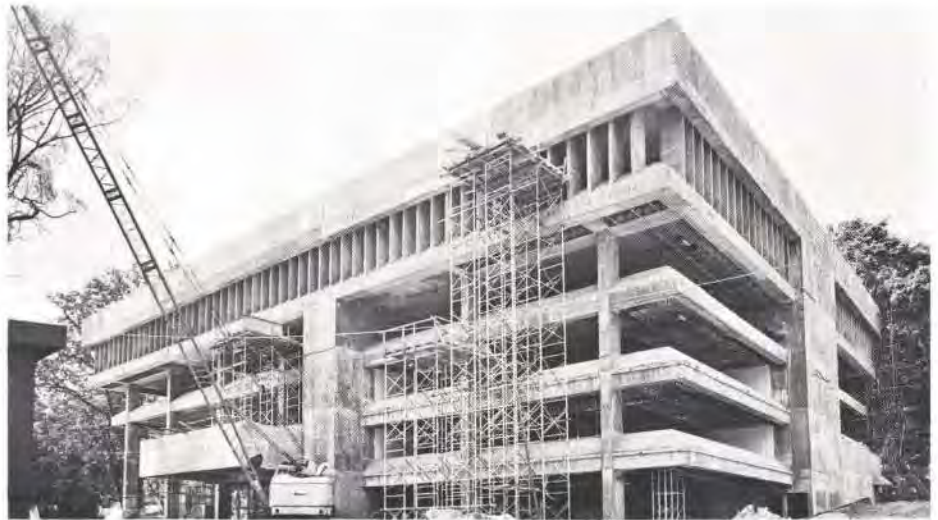
Fig. 7 Singapore High Commission under construction in 1976 (Photo: Liang's Photo Service)
