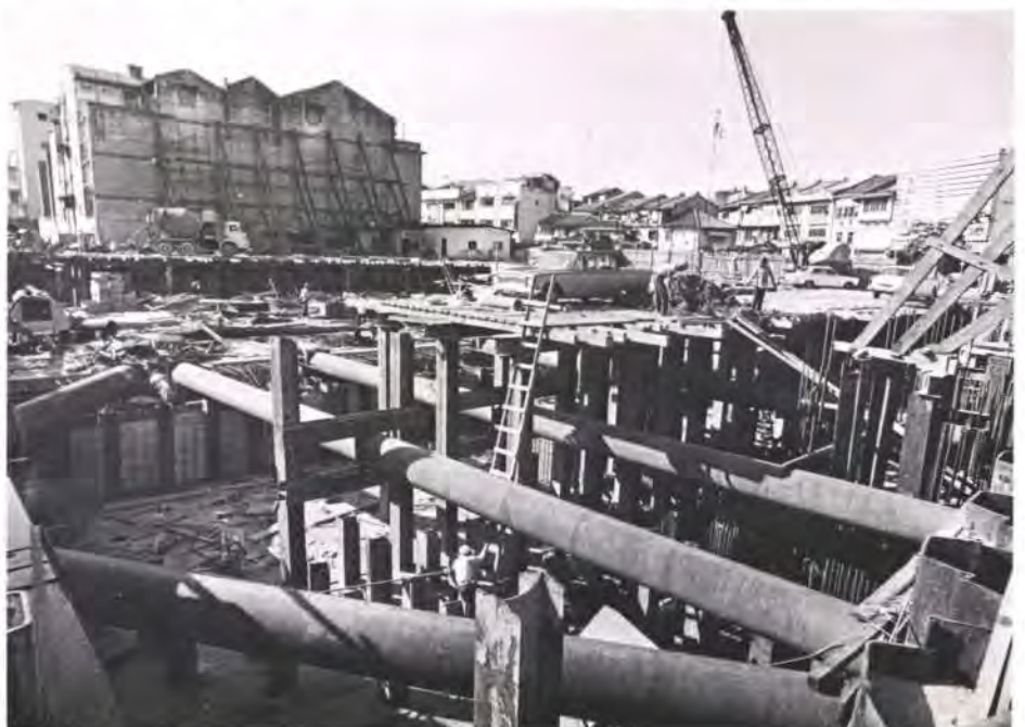
Fig. 5 Foundation piling (Photo: Kouo Shang-Wei)
