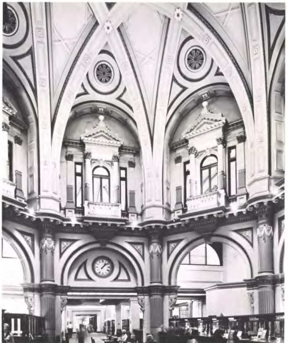
Fig. 1 Interior of the CBA banking chamber (Photo: Ian McKenzie)
