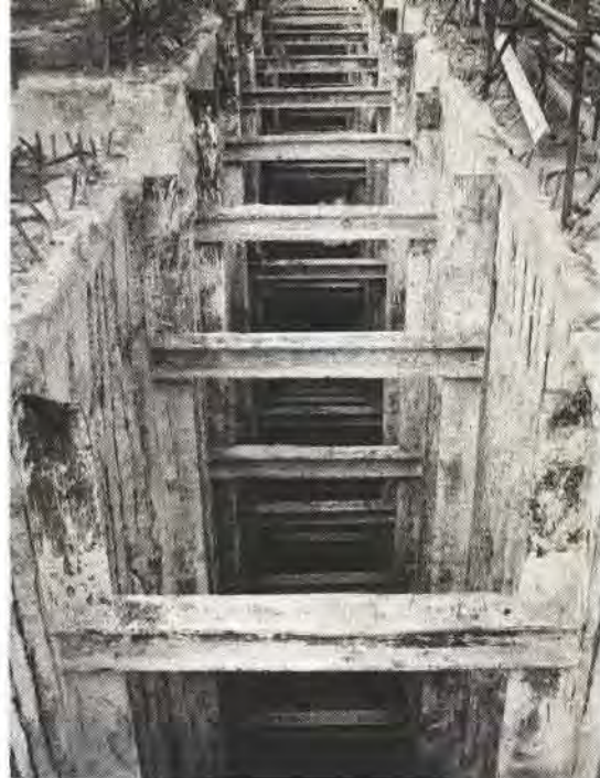
Fig. 6 The completed excavation of the south cellular wall in the theatre, showing the steel ladders (Photo: John Maltby)
