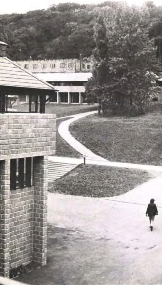
Fig. 14 Classroom block from double house
