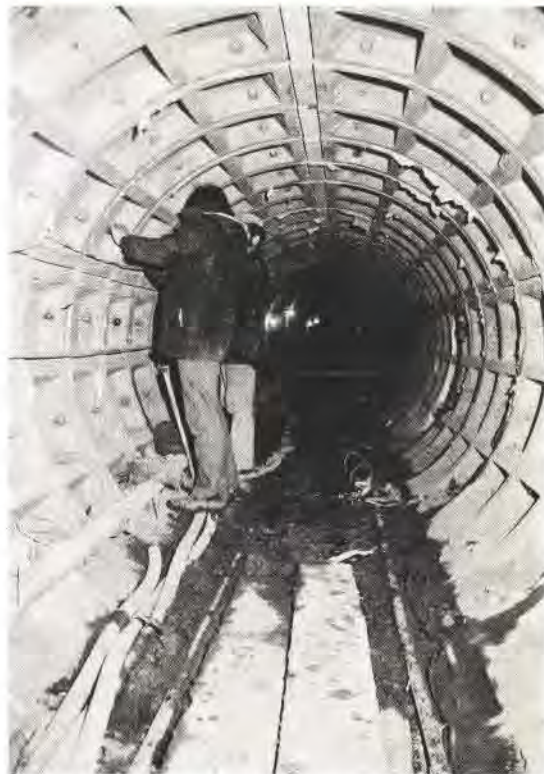
Fig. 7 The interior of the prop tunnels (Photo: John Maltby)
