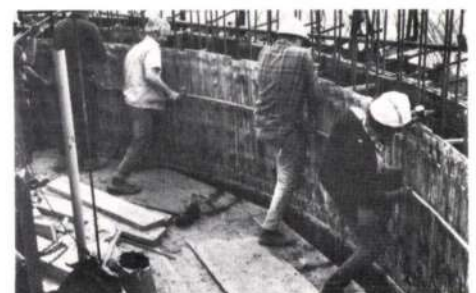
Fig. 16 Working platform (Photo : David Aldred)
