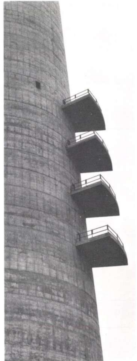
Fig. 7 above GPO platforms (Photo: Geoff Rooke)
