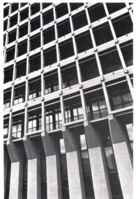
Fig 4 Close-up of precast units (Photo: Harry Sowden)
