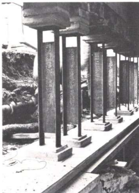
Fig. 11 Close-up of steel underpinning stools (Photo: Stan Parkinson)
