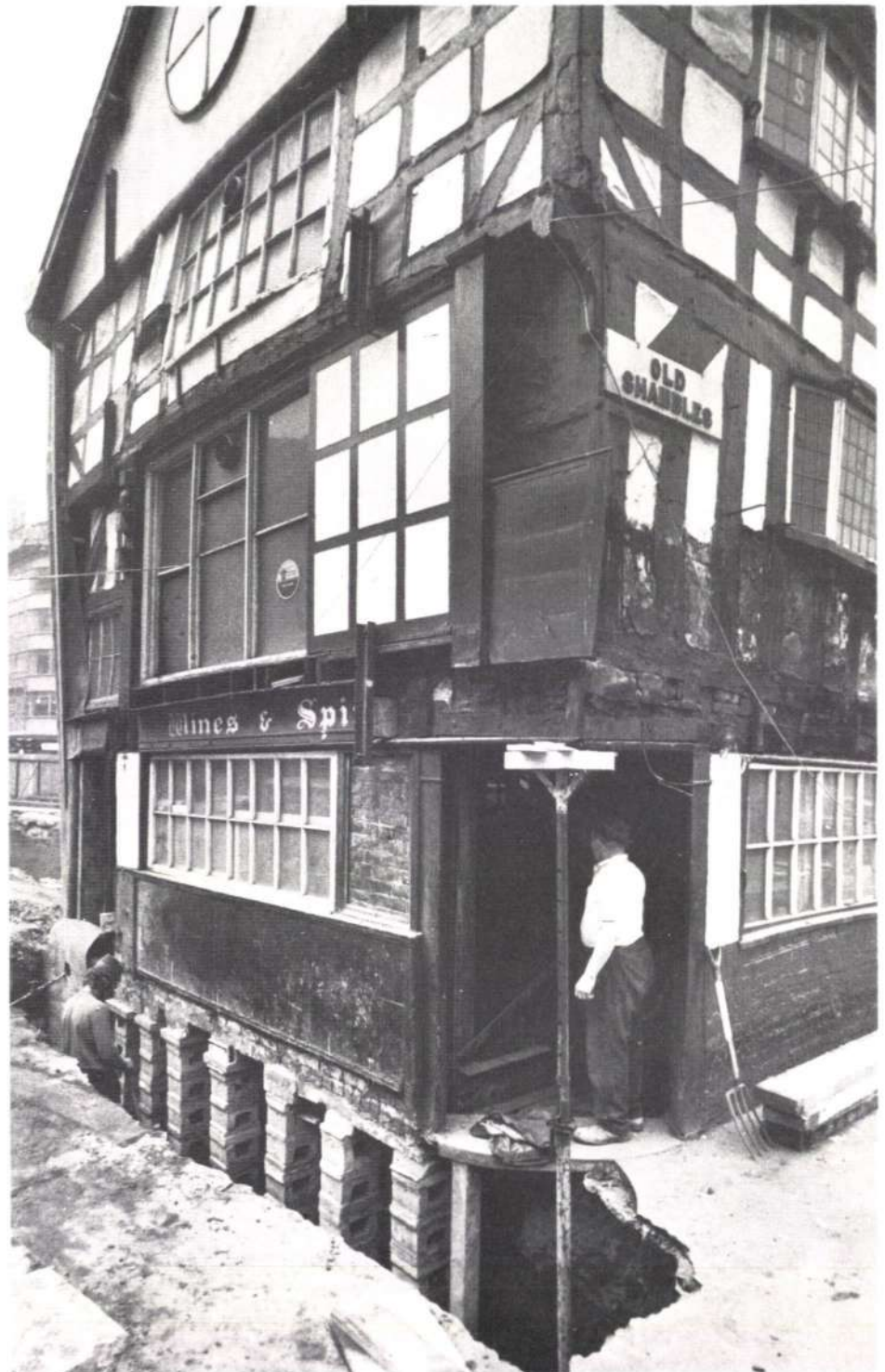
Fig. 10 Close-up of precast concrete underpinning stools (Photo: Stan Parkinson)
