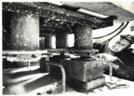
Fig. 15 All jacks on pier location No. 1 in position and first three packed against pier. Note Tentest board, angle support grillage, night rings, and continuity reinforcement. (Photo: Martin Koretz)
