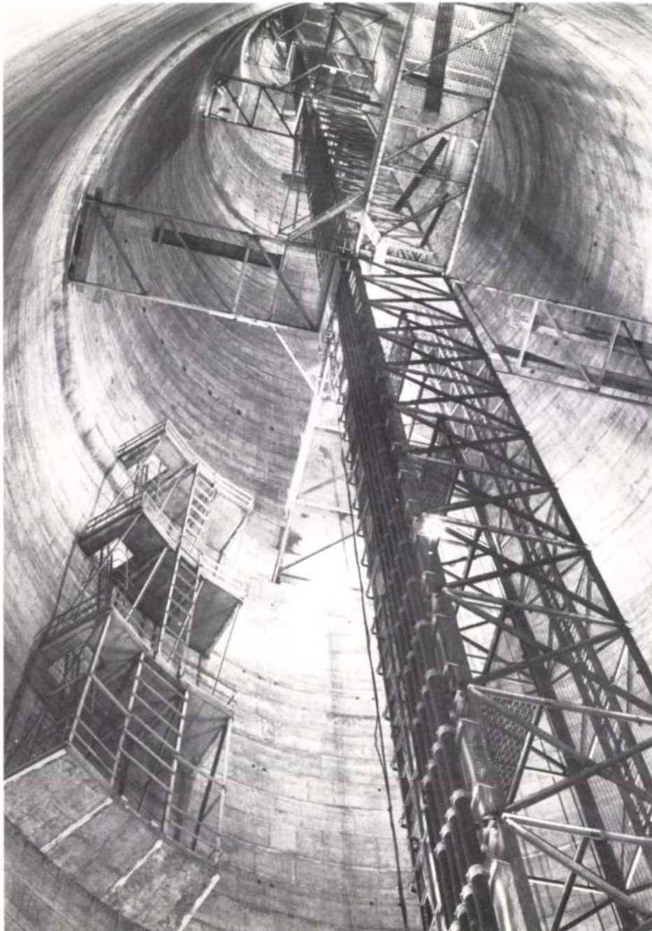
Fig. 6 below Lift cage and internal platforms (Photo: Geoff Rooke)
