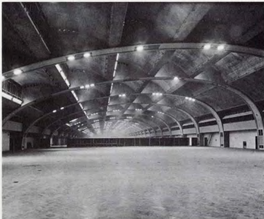
Fig. 10 Bank of England Printing Works, Debden, Loughton, Essex Architects: Easton & Robertson Completed: 1956
