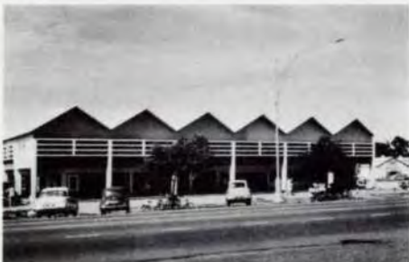
Fig. 13 UK Pavilion, Johannesburg, South Africa Architects: Fleming & Cooke Completed: 1959
