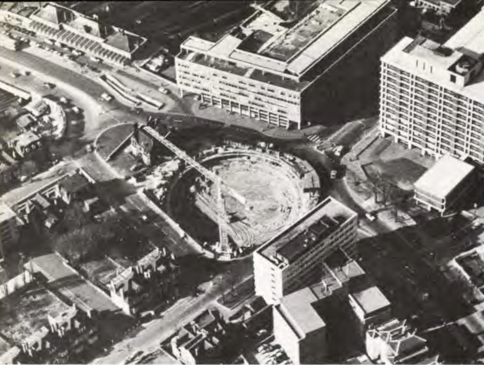
Fig. 1 Aerial view of the site during excavations. (Photo : Handford Photography)
