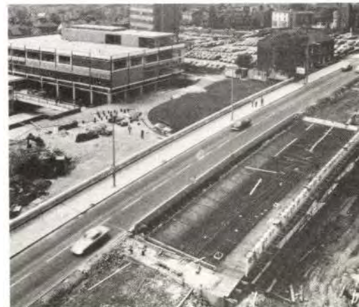
Fig. 12 above North bridge before concreting. (Photo: M. T. Walters and Associates Ltd.)
