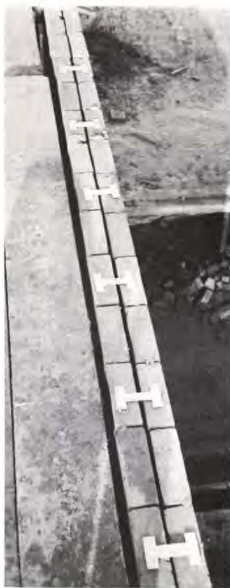
Fig. 4 6 in. loadbearing wall in stretcher bond with bricks on edge. (Photo: Peter Carr)
