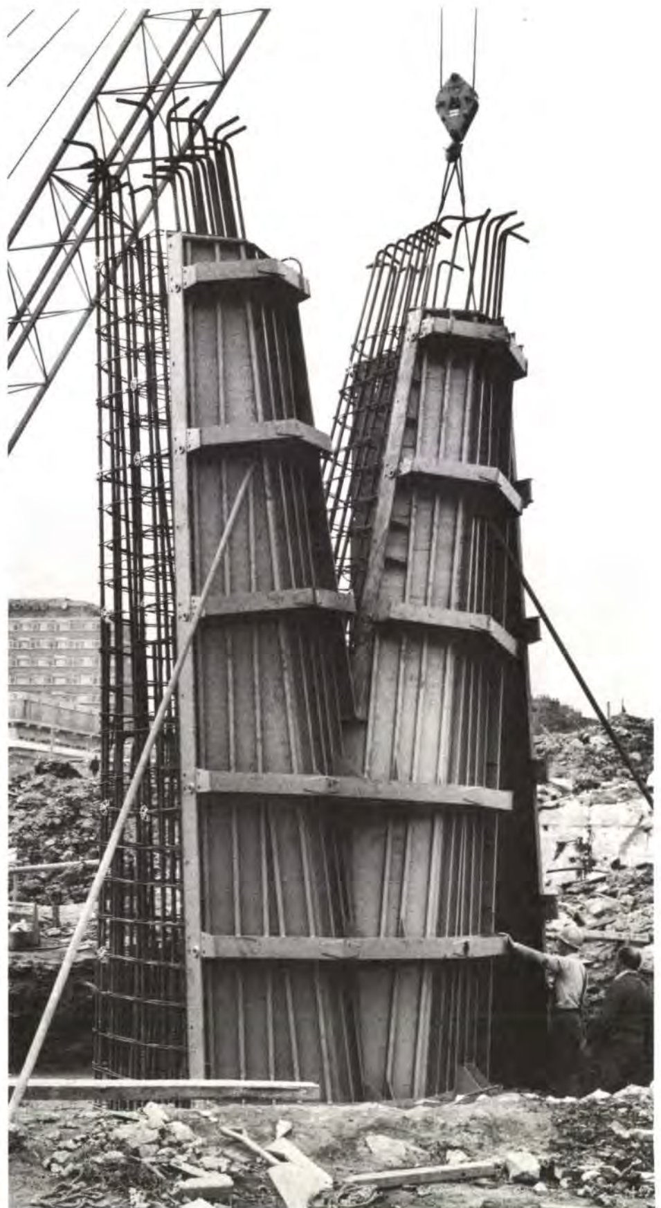
Fig. 13 Reinforcement and shuttering for main viaduct column. (Photo by : R. Knibbs)
